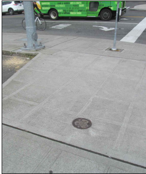
Photograph 1: View looking north at well MW-10 prior to well modification work. This well is situated on the sidewalk adjacent to the west of Queen Anne Avenue North.
