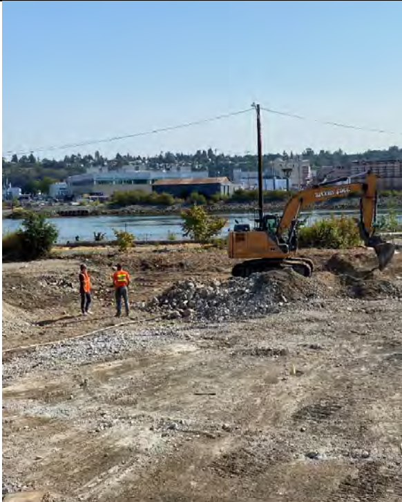
Concrete Demo and Surface Soil Removal
