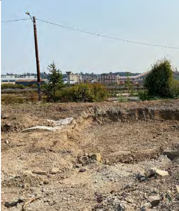
Concrete Demo and Surface Soil Removal
