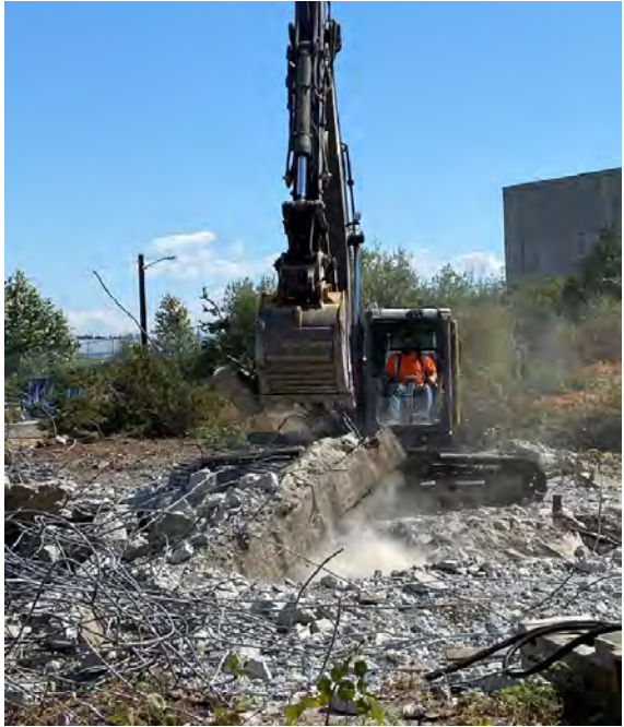
Site Preparation Concrete Demo – Notice 1' – 2' thick concrete
