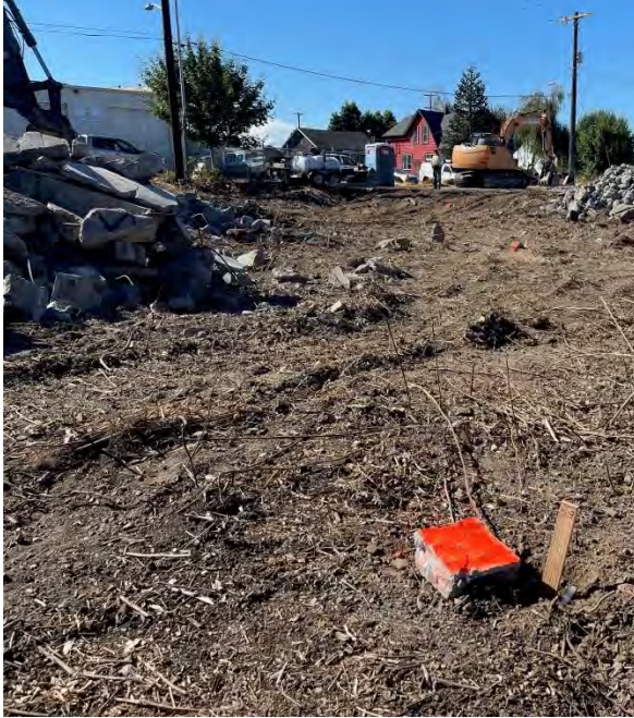
Cleanup Excavation In Area where Former Owner Removed Soil
