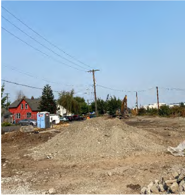
Cleanup Excavation Zone 2 Soil Excavation
