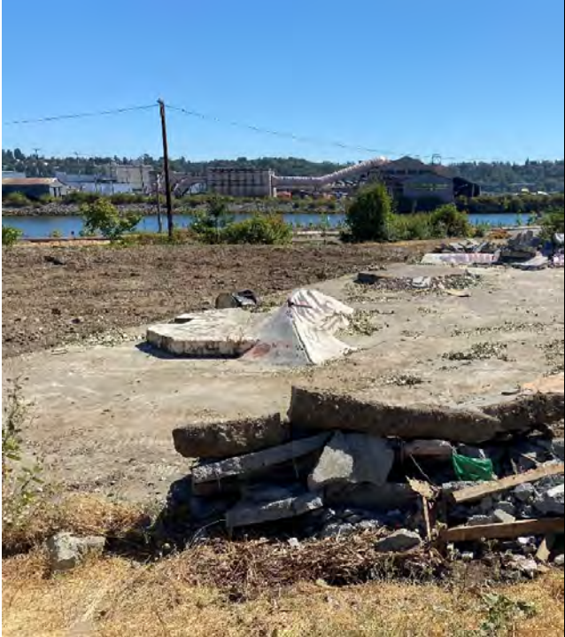
Site Preparation Clearing and Trash Removal
