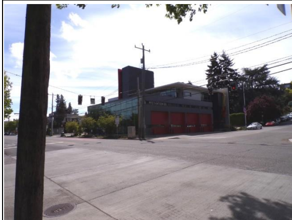
Photo # 17 Fire Station adjoining to the southeast
