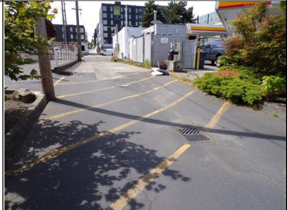
Photo # 22 Storm drain and monitoring wells
