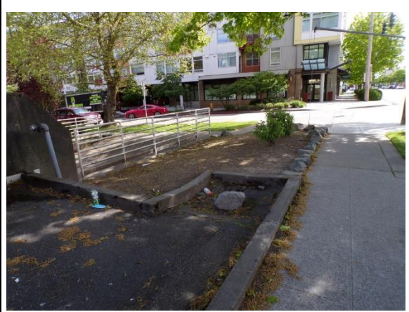
Photo # 14 One of the storm drains on the subject property
