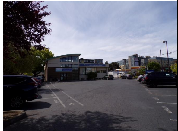
Photo # 24 South-facing view of the subject property and the adjoining gasoline station
