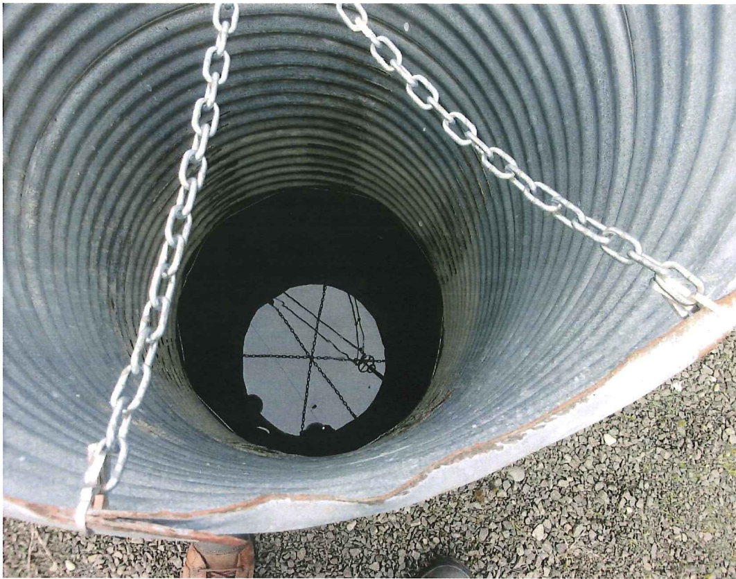
Interior of Groundwater Monitoring Culvert.
