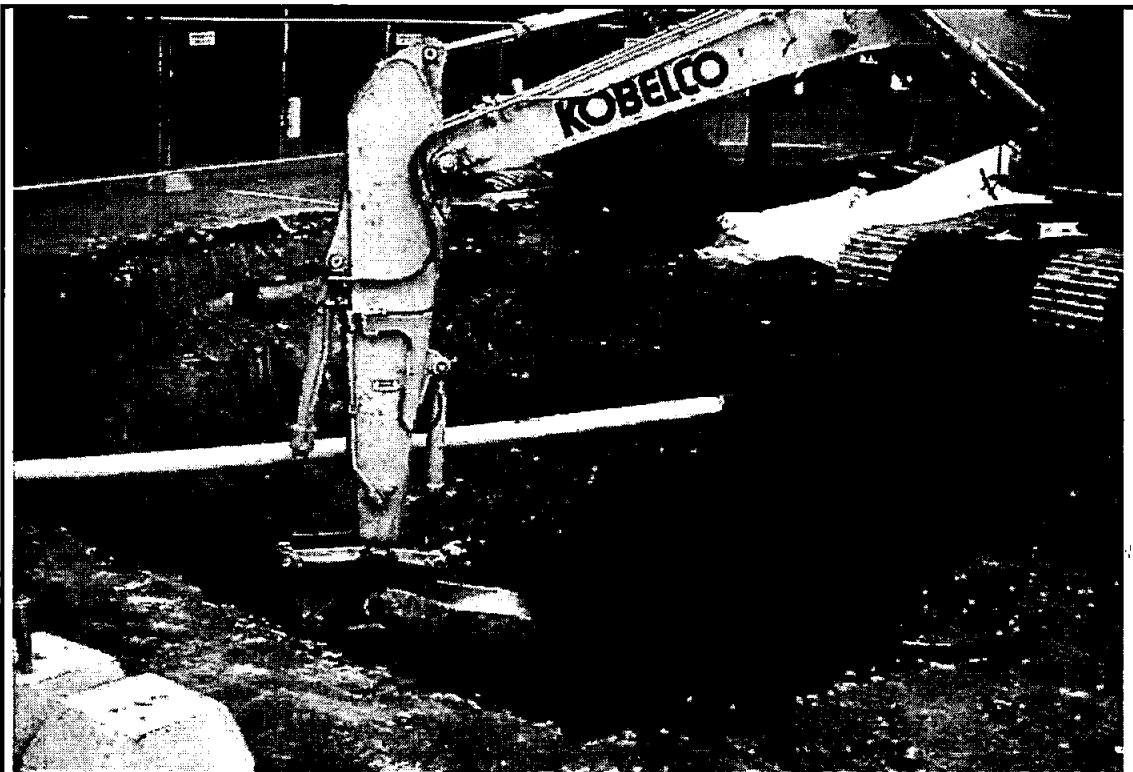
Photograph: 4 Snohomish Square Cleaners Facility ERM Active Excavation
