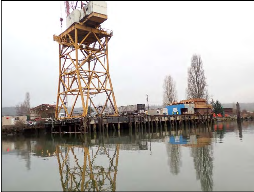
Photo 3 : Overall view, looking west.
