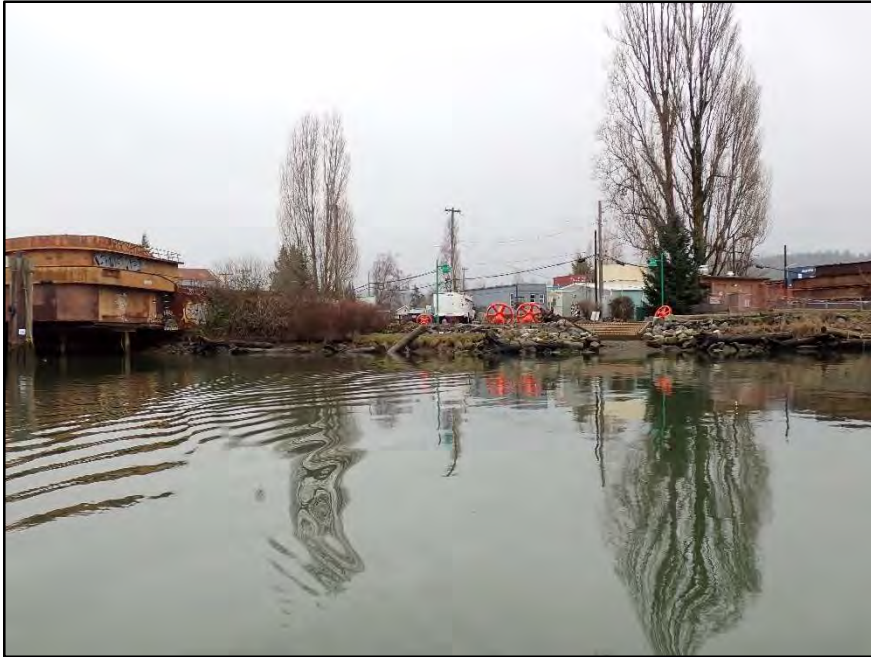
Photo 5 : North embankment, looking west.
