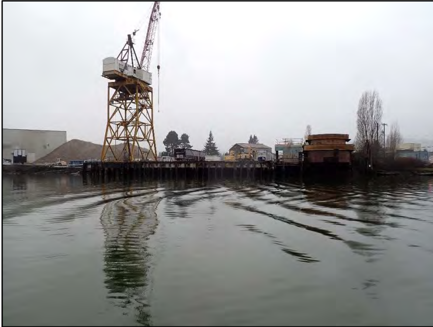
Photo 1 : Overall view, looking southwest.
