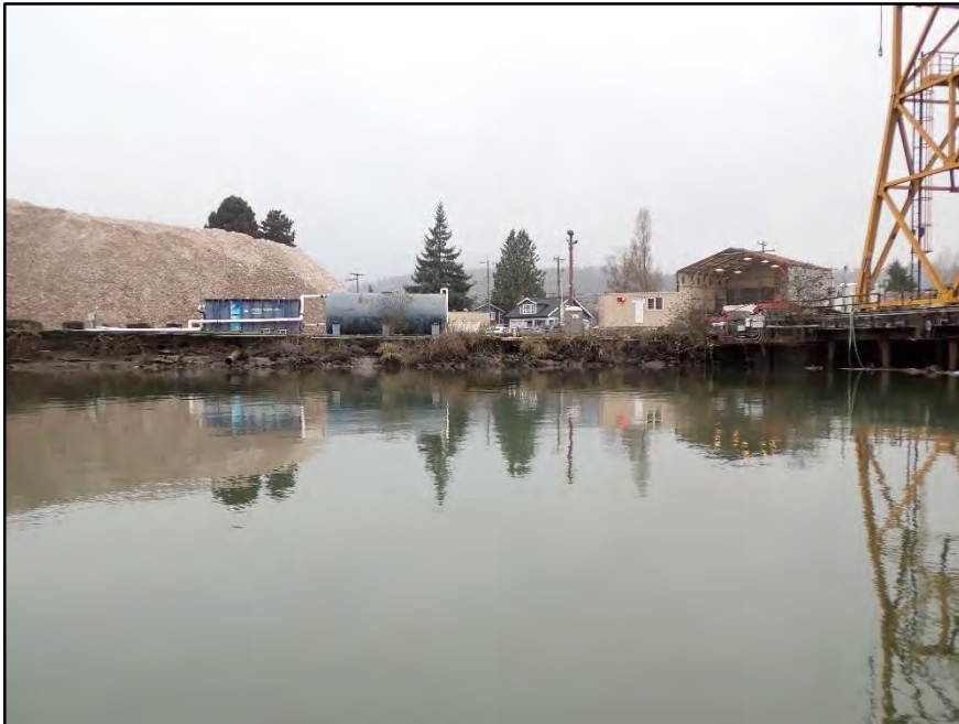
Photo 4 : South embankment, looking west.
