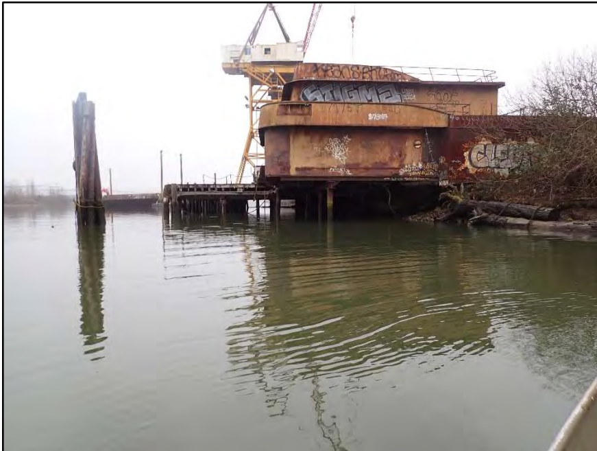
Photo 2 : Overall view, looking southeast.
