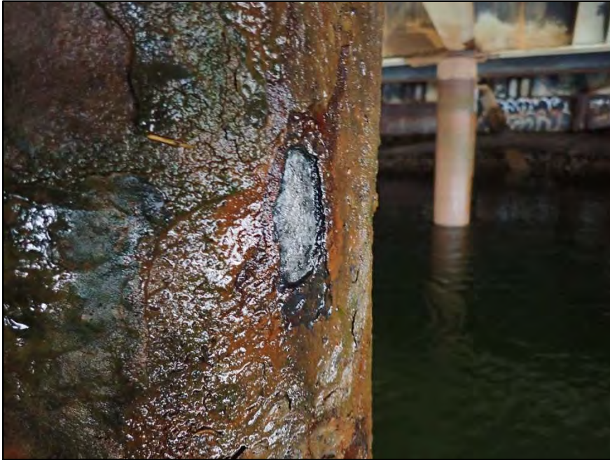
Photo 11 : Typical condition of cleaned steel, Bent 10 Pile E, looking west
