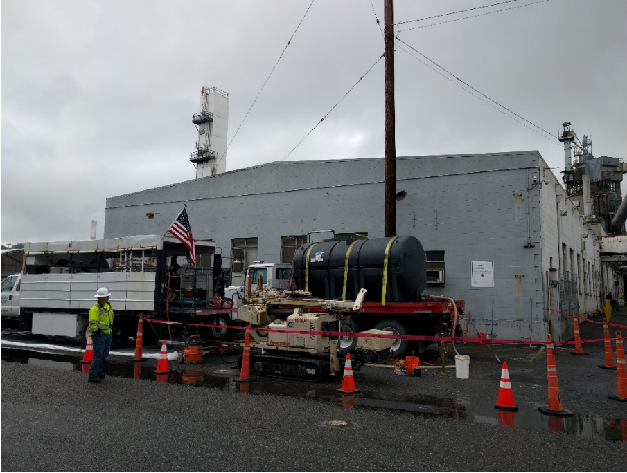
Photograph 1. Cascade's equipment layout for direct push injections.
