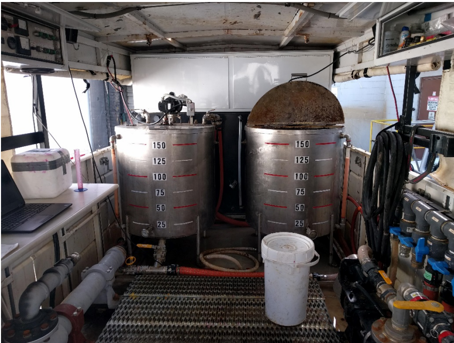
Photograph 2. Batch mixing set-up.
