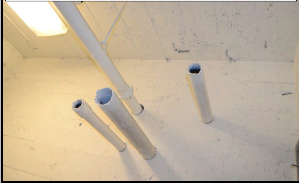
Fig. 4: Numerous Penetrations in Walls Complicates Positive or Negative Pressurization of the Air Spaces.
