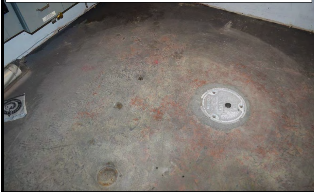
Fig. 6: Interior Monitoring Well
