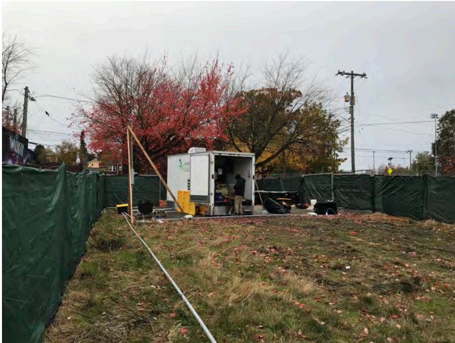
Photograph 19 Date: 11/11/22 Southwestern view of gravel pad, remediation system trailer, temporary power pole with bracing per Seattle City Light specifications, conveyance line conduit and junction box, injection well nests INJ-4s/4d and INJ 3s/3d and drilling waste storage
