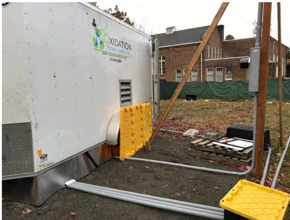
Photograph 13 Date: 11/11/22 Northwestern view of gravel pad, remediation system trailer, temporary power pole with bracing per Seattle City Light specifications, electrical conduit, conveyance line conduit and junction box, and injection well nests INJ-4s/4d near the trailer and INJ-1s/1d in the background
