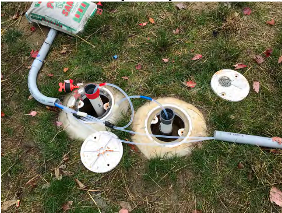
Photograph 18 Date: 11/11/22 View of conveyance line conduit and injection wells INJ-2d and INJ-2s
