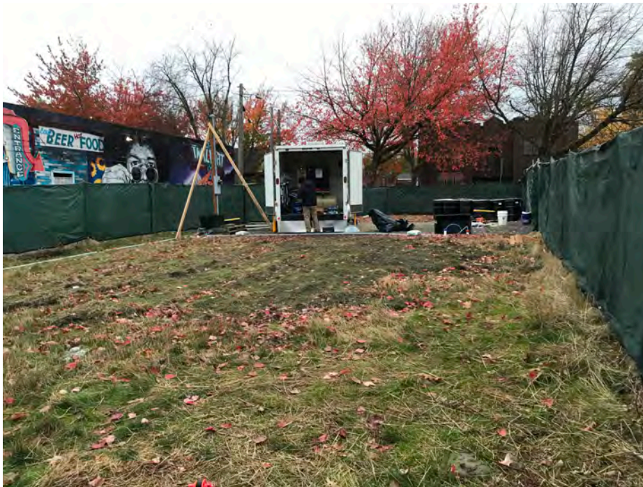
Photograph 17 Date: 11/11/22 Southeastern view of gravel pad, remediation system trailer, temporary power pole with bracing per Seattle City Light specifications, conveyance line conduit and junction box, injection well nests INJ-4s/4d and INJ 3s/3d and drilling waste storage
