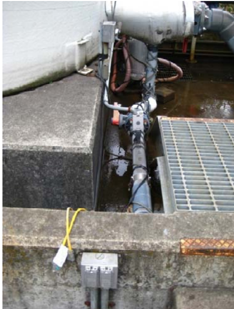
Figure 5. Heat tracing (black) placed throughout lines near effluent storage tank.
