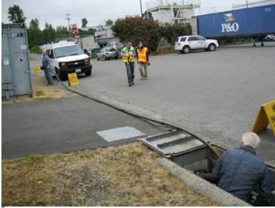
Figure 9. EW-3 during pump pull. Black HDPE tubing was replaced due to fouling.
