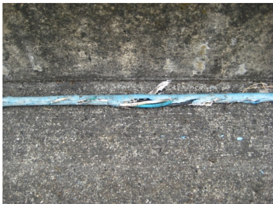
Figure 7. Frayed wiring present in several locations at the GETS.
