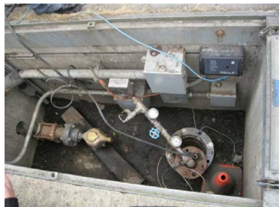
Figure 8. EW-3 during pump pull. Piping was dismantled to remove the pump.
