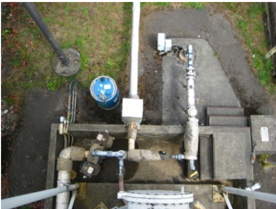
Figure 3. Extraction well 1 (EW-1).
