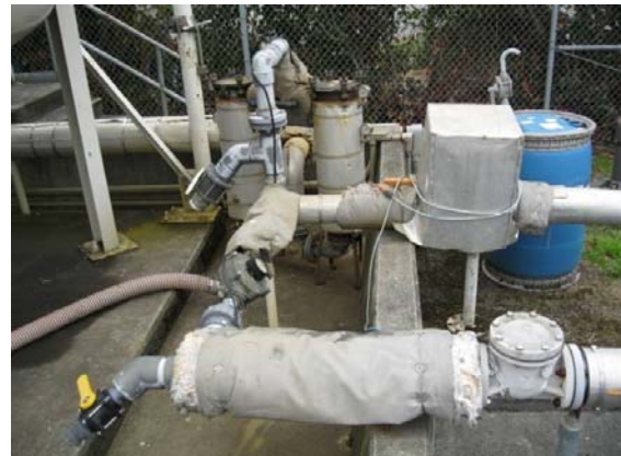
Figure 4. Header for water from extraction wells to treatment system. Dual bag filters in background.
