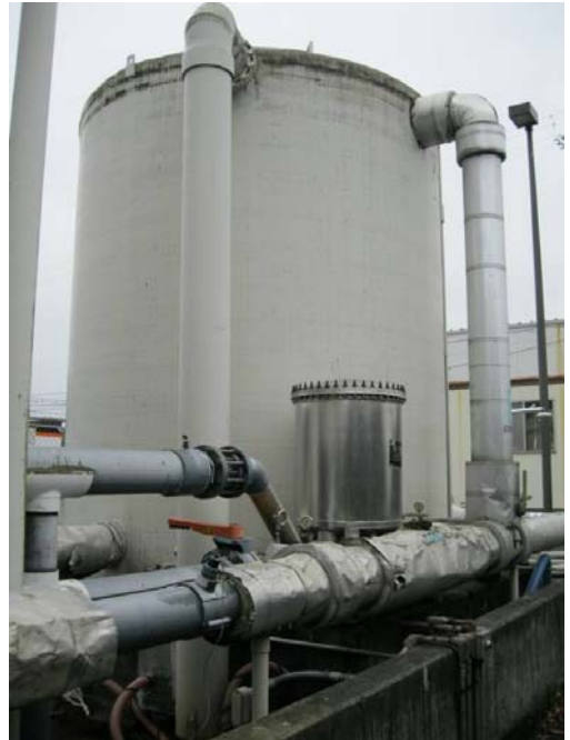
Figure 6. Effluent storage tank and piping. Several stretches of piping without insulation.
