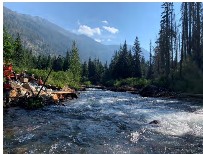
Photo 220 — Downstream view of SG-9.
