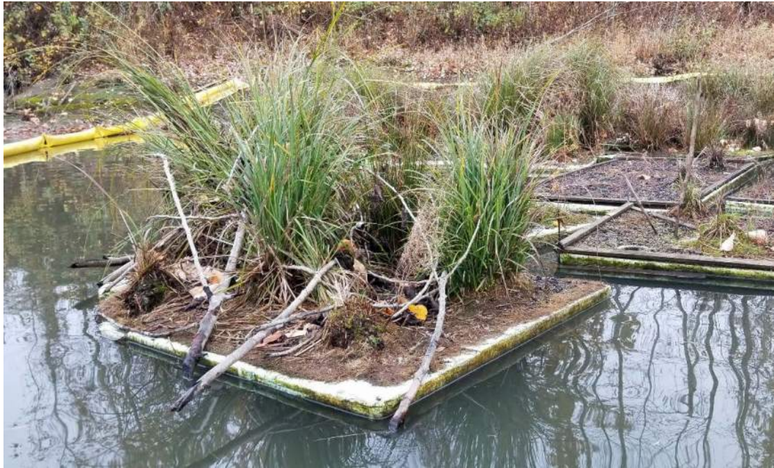
Photo #7: Damage to FTW: Evidence of beaver activity
