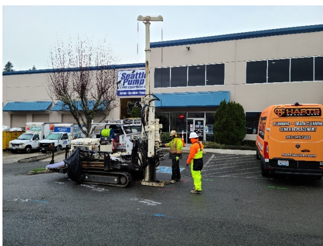
15. Collecting soil samples along the southeast side of the building.
