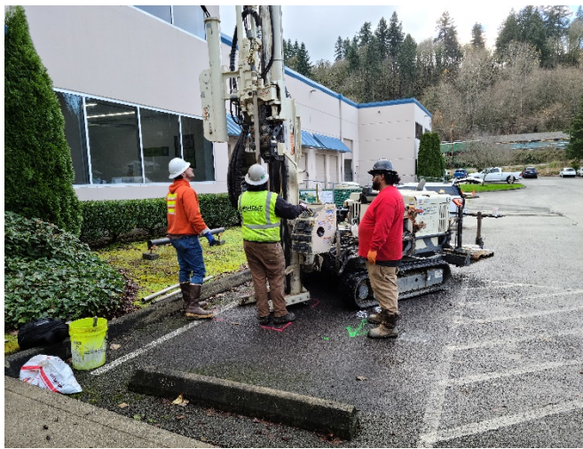
13. Collecting soil samples along the north side of the building.
