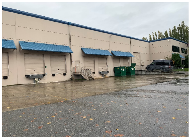
2. View of the south side of the 16750 building.
