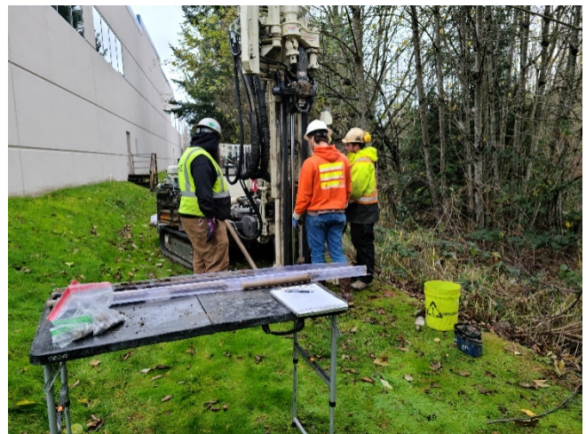
10. Collecting soil samples along the southeast side of the building.
