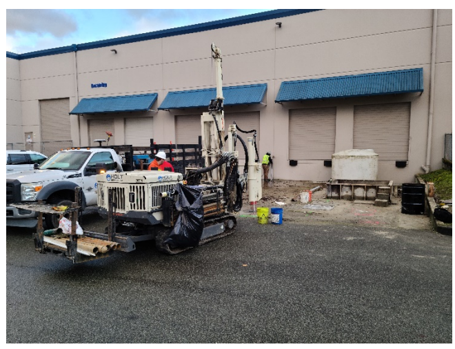
14. Collecting soil samples near the oil/water separator at the north side of the building.
