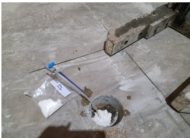
17. Sealing borehole with VOC playdough before collecting soil gas sample.
