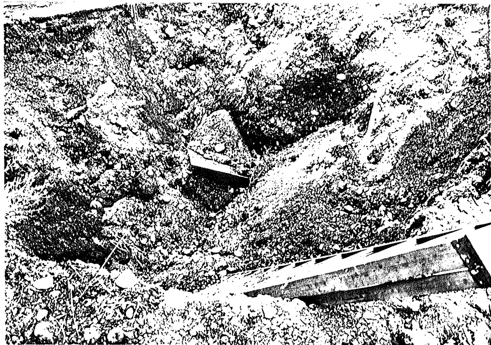
Photograph 14. The pit after the UST was removed. Note the soil discoloration beneath the metal sheet in the center of the photograph. The discoloration along the right side of the photograph is from the liquid spilled from the UST. Looking west-southwest.
