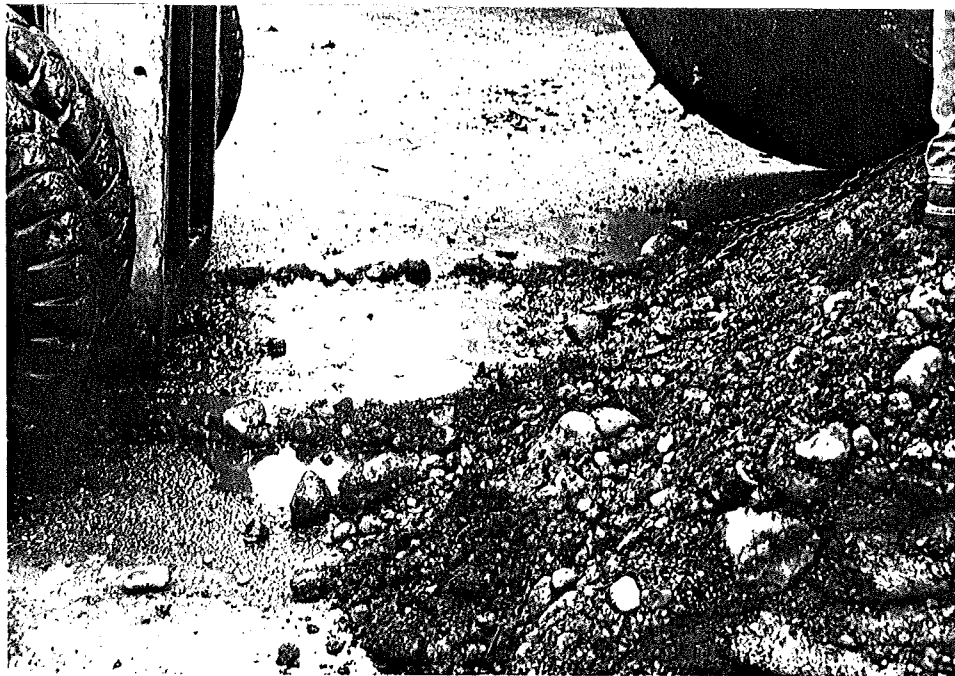
Photograph 8. The liquid which spilled from the tank while it was being removed from the pit.
