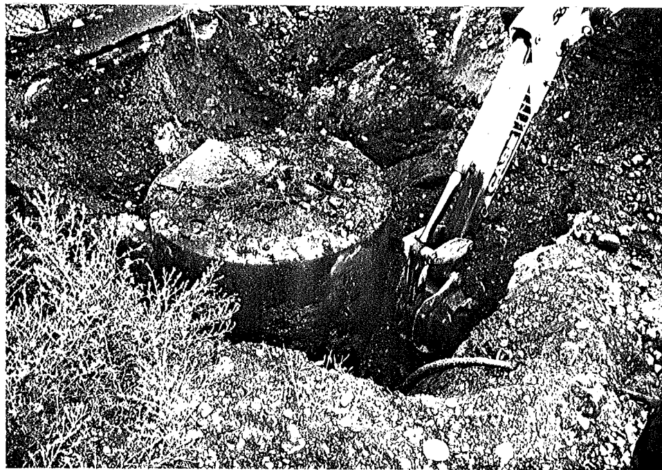
Photograph 4. Excavating the UST. Note the broken water pipe in the lower right corner of the picture, Looking southwest.
