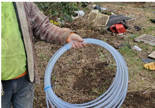
Photo number 3: 0.25" diameter Teflon tubing installed at each probe.
