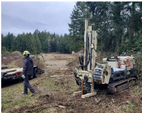
Photo number 1: geoprobe drill rig used to install temporary probes.
