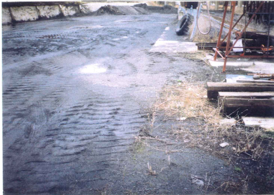
NOTE STAINED SOIL AT BASE OF TANK
