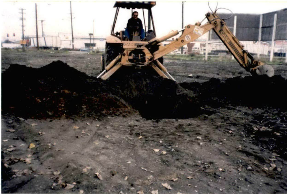
Completion of Test-Pit #5; note sawdust which can be found in fill material at the site.
