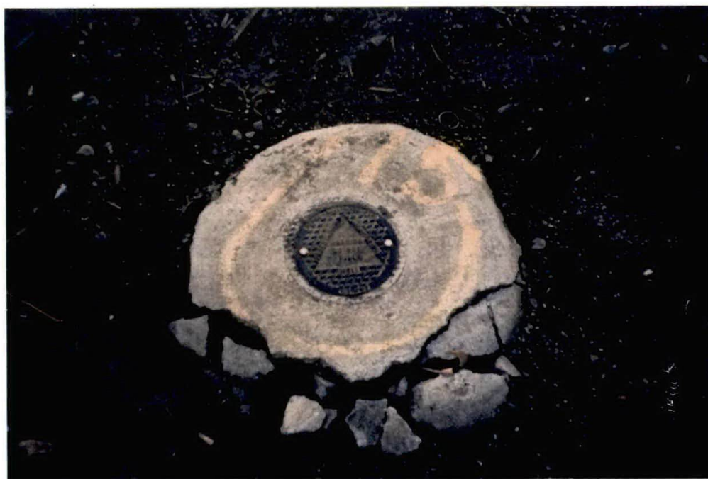
Existing groundwater monitoring well (MW-15) along E. Marginal Way South.
