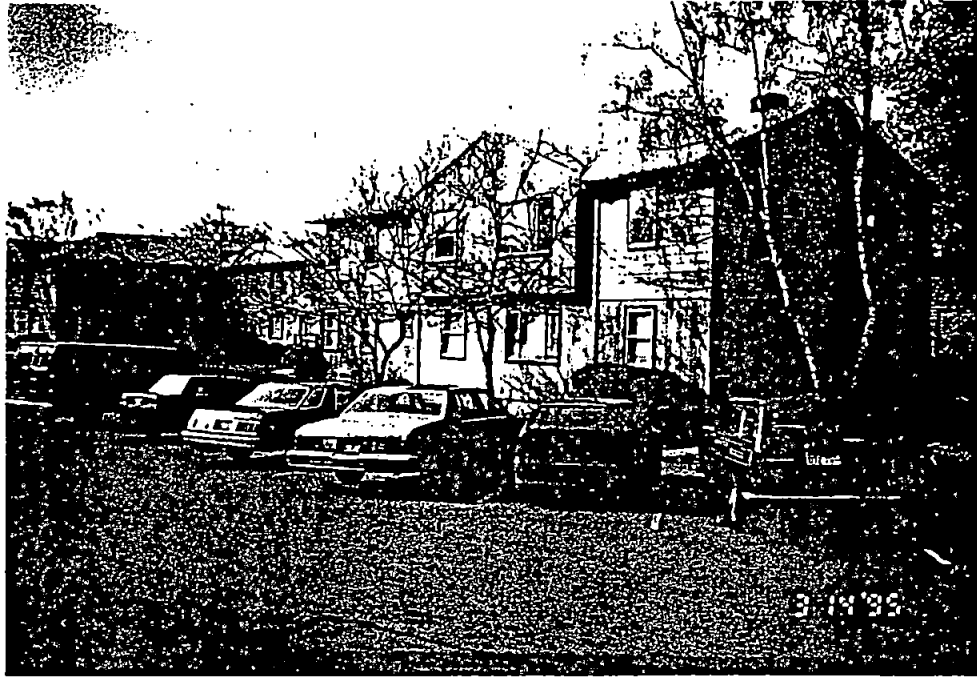
Exterior view of subject site, photo taken 03/14/95.
