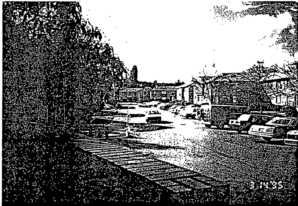
Exterior view of subject site, photo taken 03/14/95.
