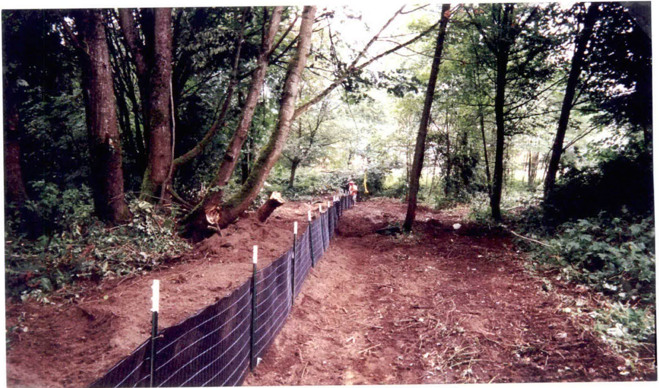
Silt Fence Installation – Eastern Property Boundary
