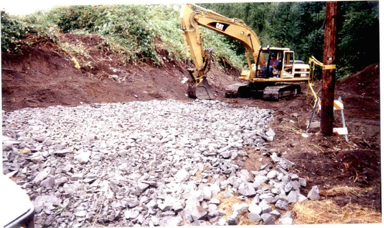
Construction Entrance For Phase I Excavation
