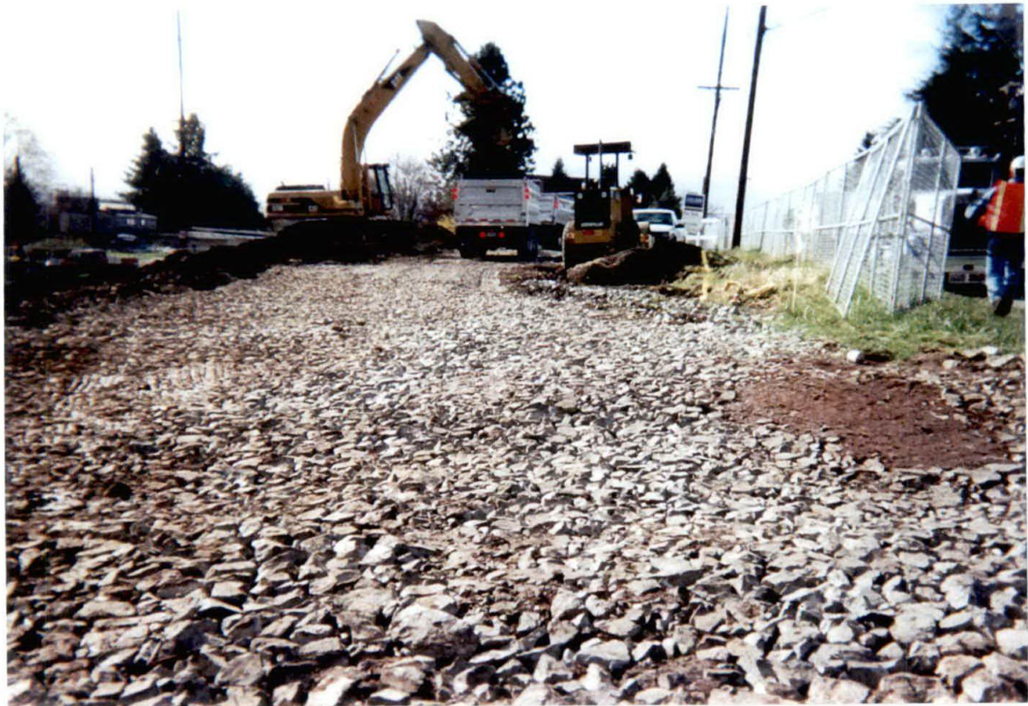
Construction Entrance Phase II Excavation
