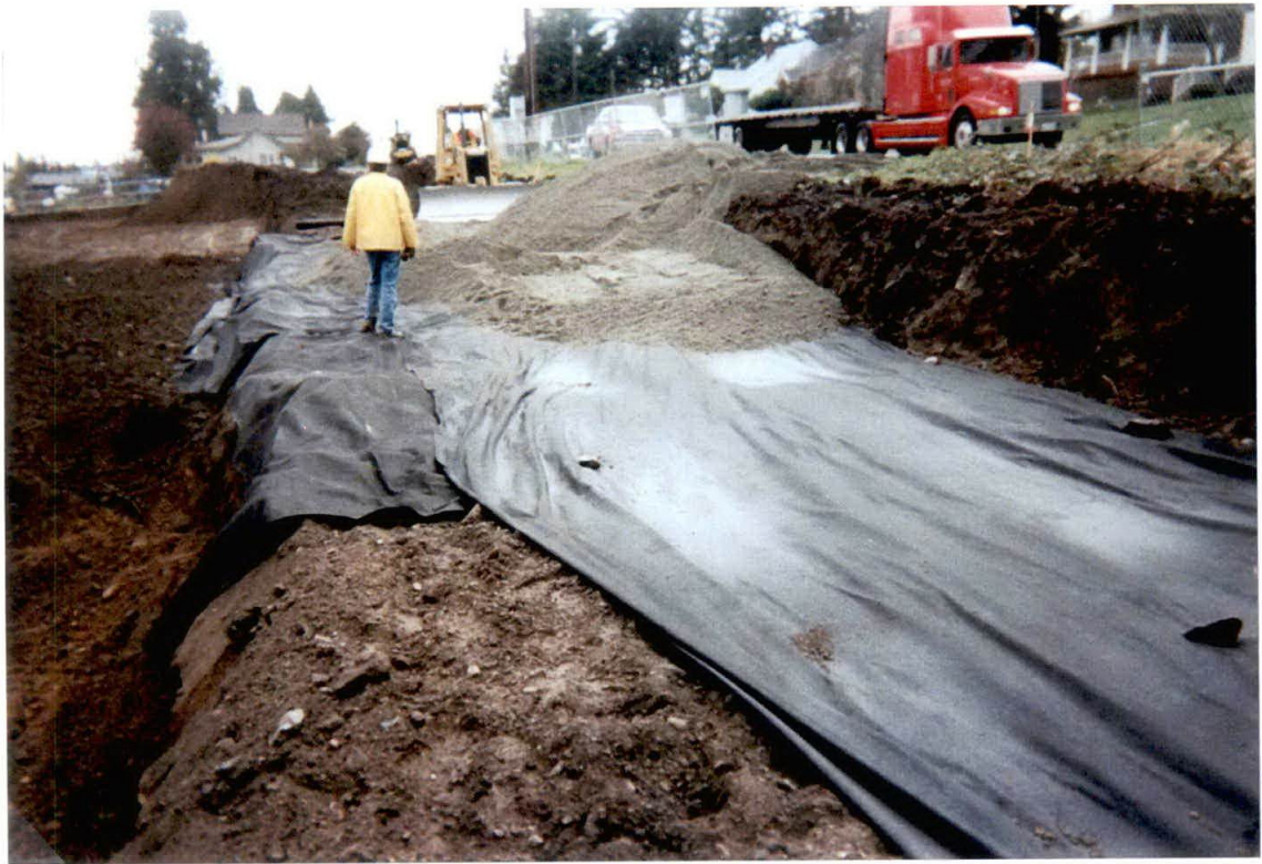
Placement Of Fill Sand And Fabric In Landscape Strip – Phase II
