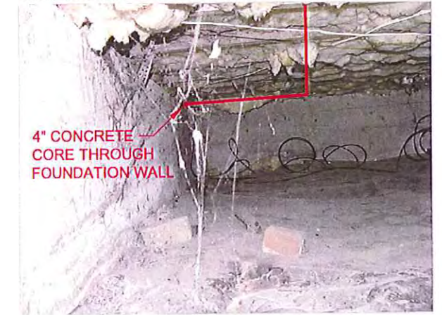
VIEW OF DISCHARGE LOCATION
