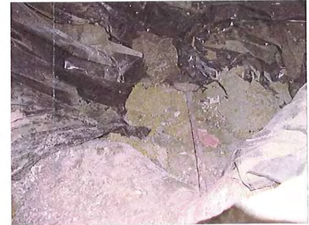
VIEW OF CRAWLSPACE SUMP AREA
