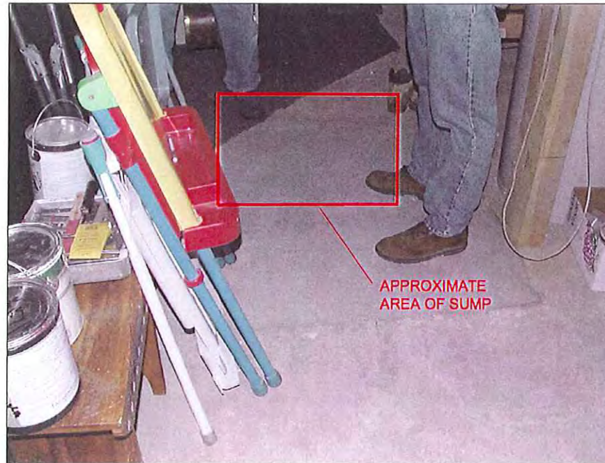
UNFINISHED FLOOR - SUMP AREA
