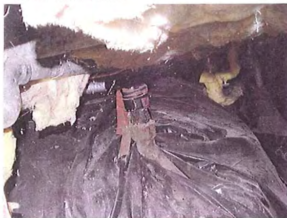
VIEW OF CRAWLSPACE
