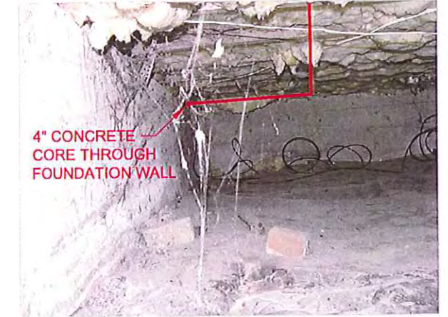
VIEW OF DISCHARGE LOCATION
