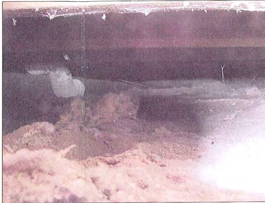
PHOTO "B" VIEW OF CRAWL SPACE ACCESS - VIEW 1
