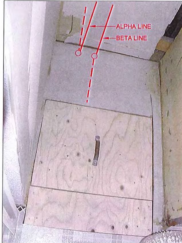
LAUNDRY CLOSET SUBFLOOR ACCESS POINT
