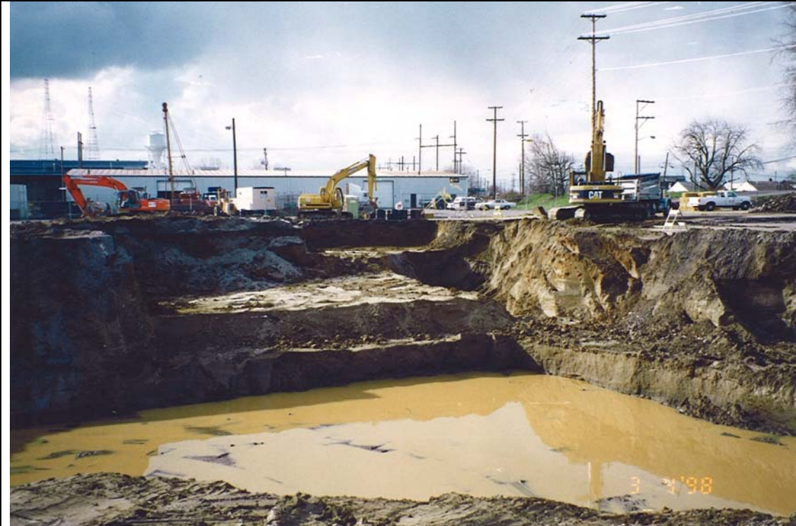
Photograph 35: Remedial excavation at greatest depth. Groundwater fills bottom of excavation.
