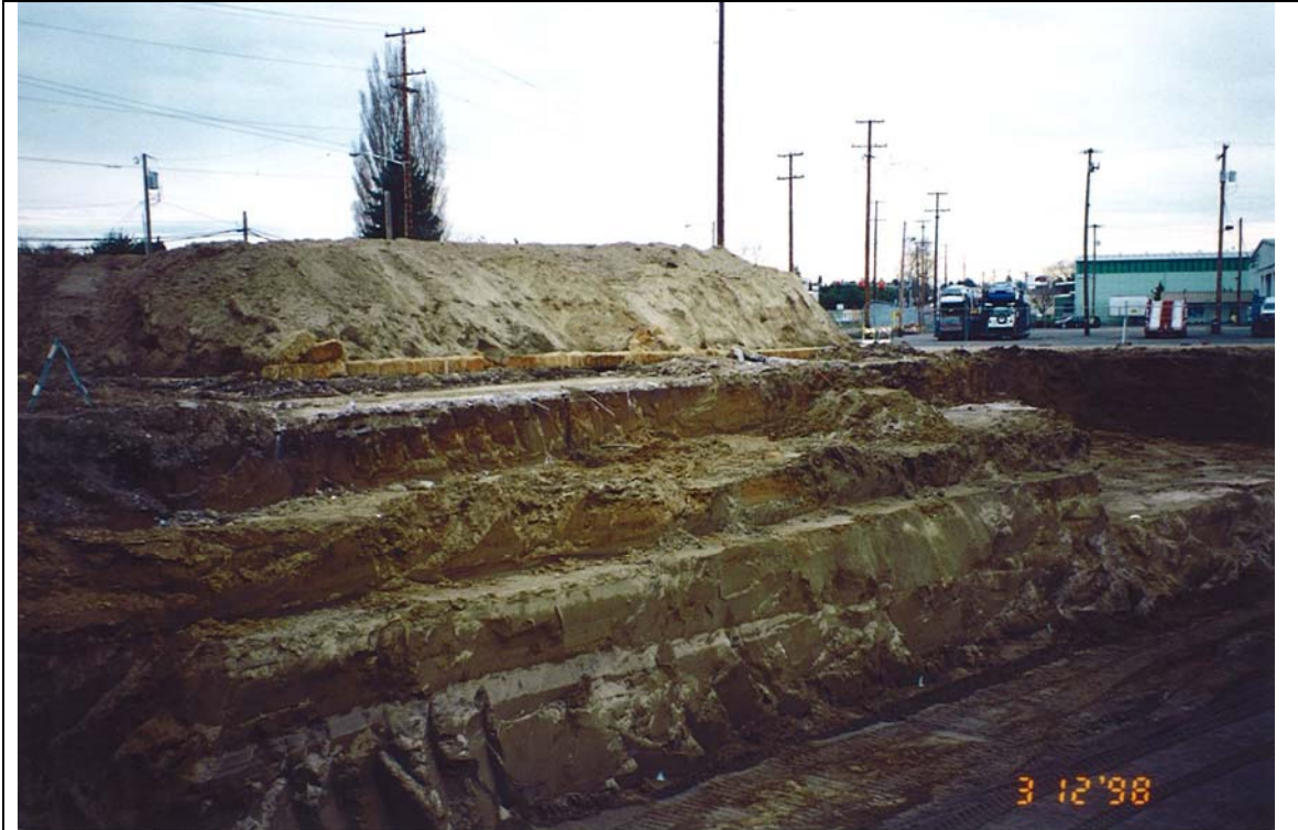
Photograph 39: Remedial excavation showing SMC concrete slab. Looking northeast.
