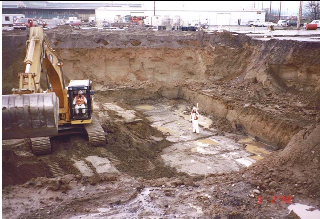
Photograph 34: Remedial excavation, looking northwest.
