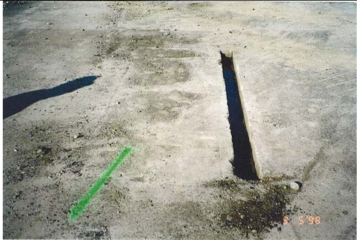
Photograph 10: Slot in central part of SMC concrete slab, looking west.
