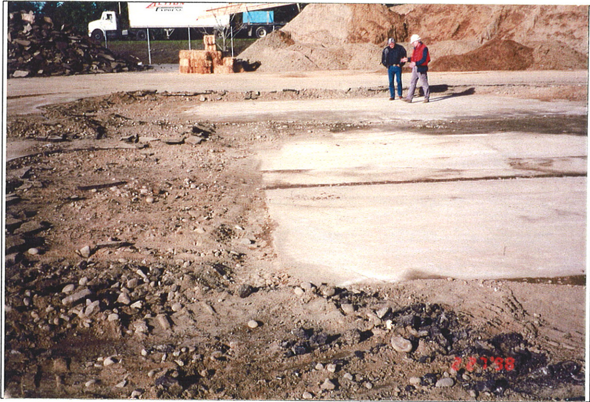
Photograph 5: Southern extension and western part of SMC concrete slab, looking north.
