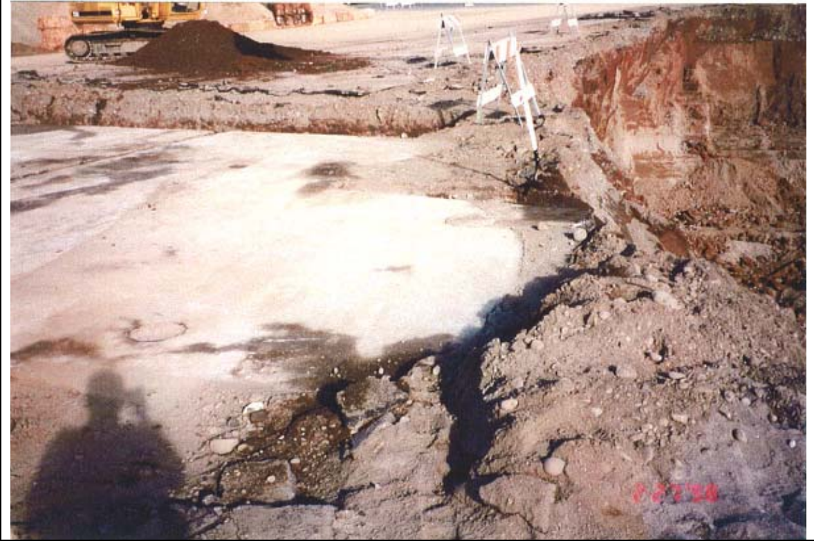
Photograph 1: Southern extension of SMC concrete slab, looking northeast.
