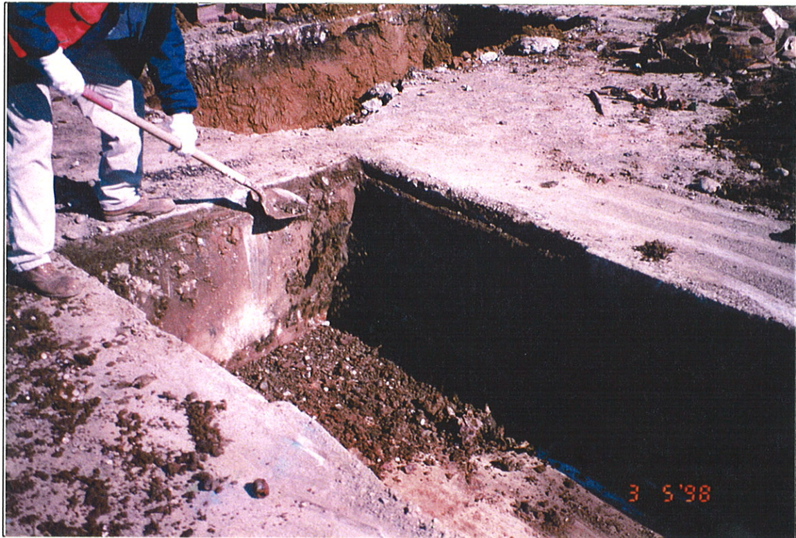
Photograph 16: Concrete vault/pit in SMC concrete floor slab, looking northeast.
