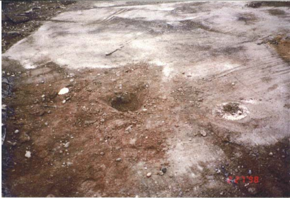
Photograph 2: Southwest corner of southern extension of SMC concrete slab, looking north.
