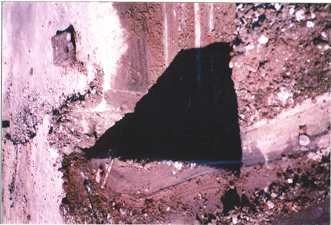
Photograph 18: Southern end of concrete vault/pit. Photograph shows short "leg" of vault to west of the large section of vault.
