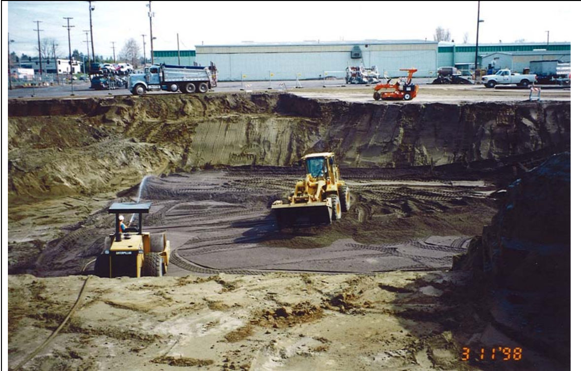
Photograph 37: Backfilling of remedial excavation begins.
