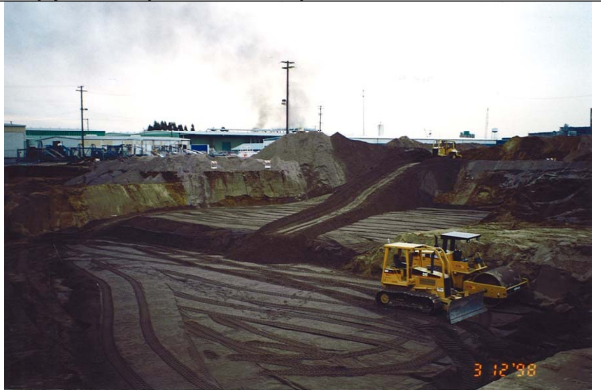
Photograph 38: Backfilling of remedial excavation.
