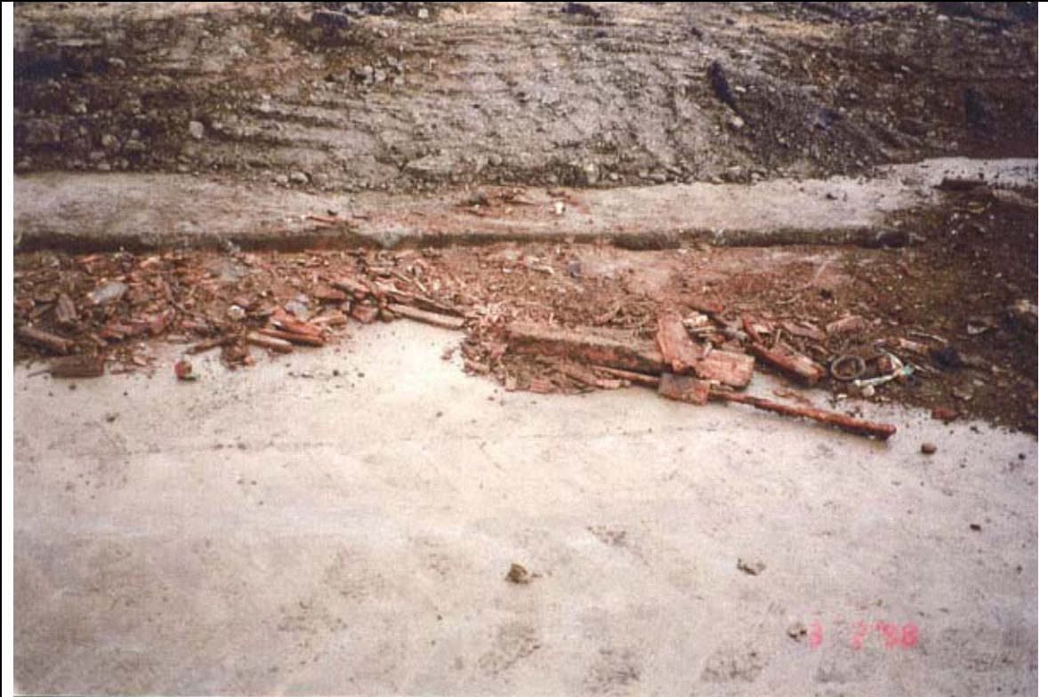
Photograph 9: Slot in central part of SMC concrete slab, looking north.
