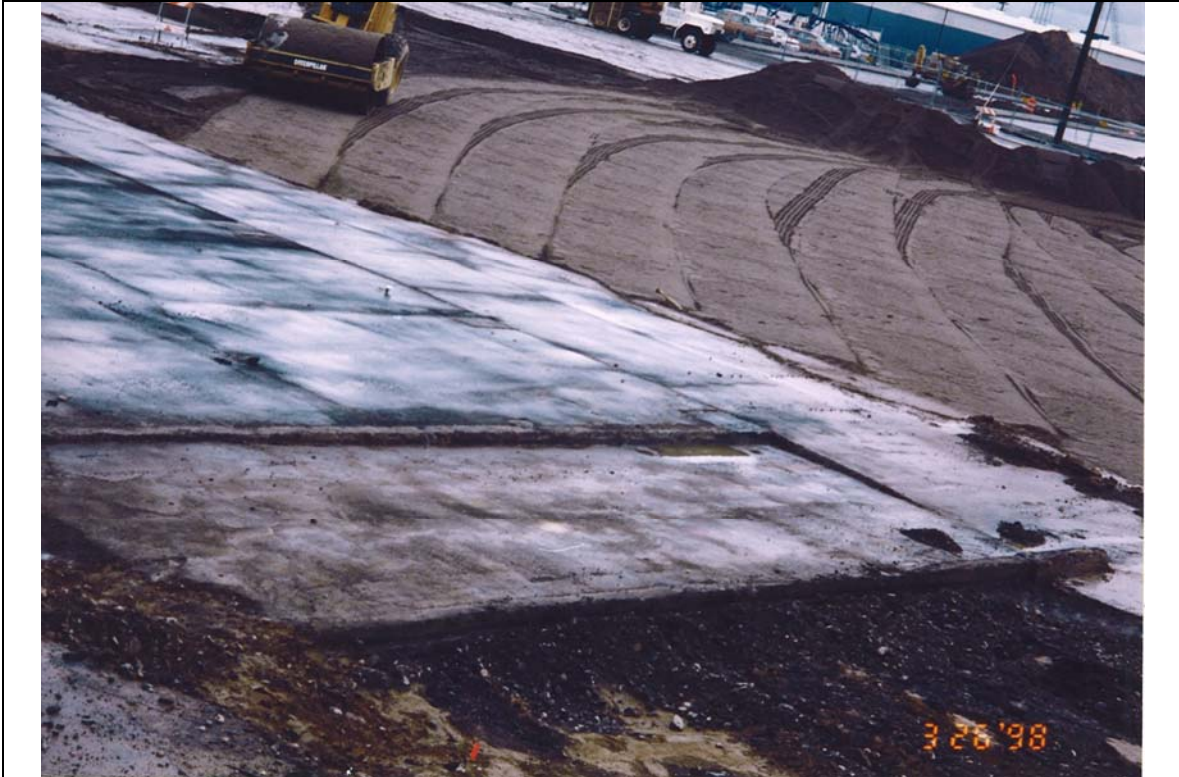
Photograph 41: Backfilling of remedial excavation. SMC slab in foreground.
