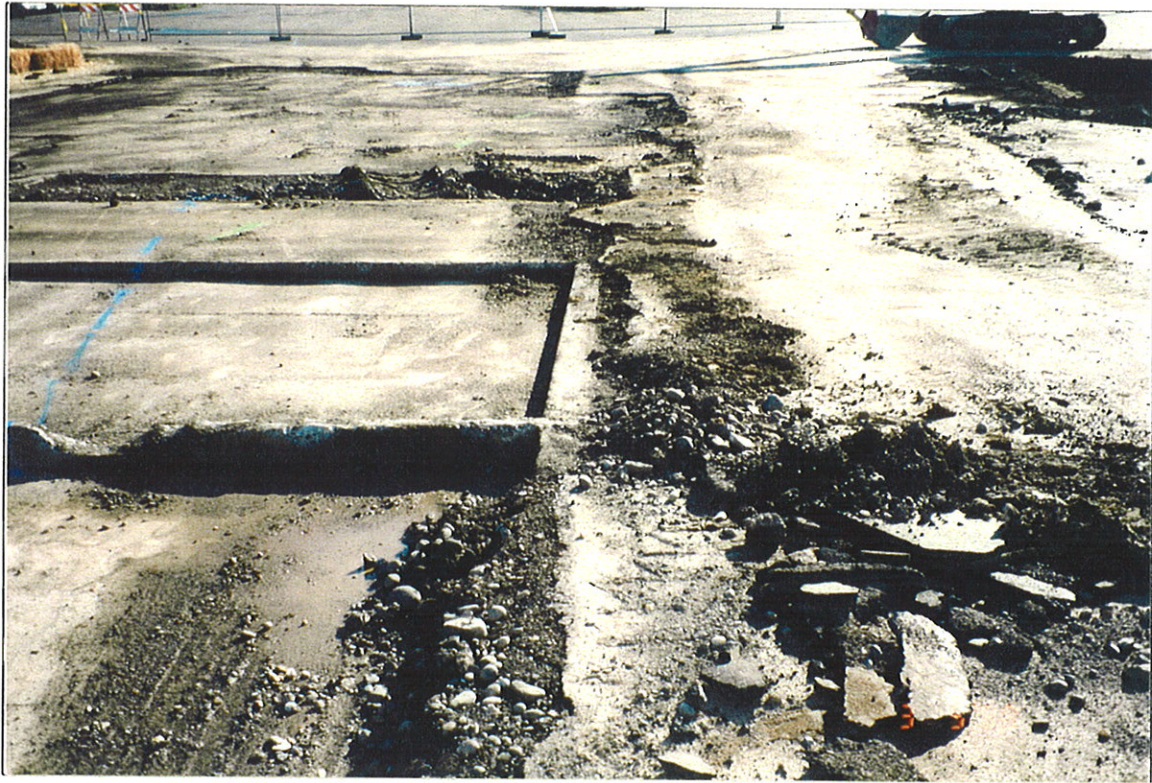
Photograph 13: Central part of SMC concrete floor slab, looking east.
