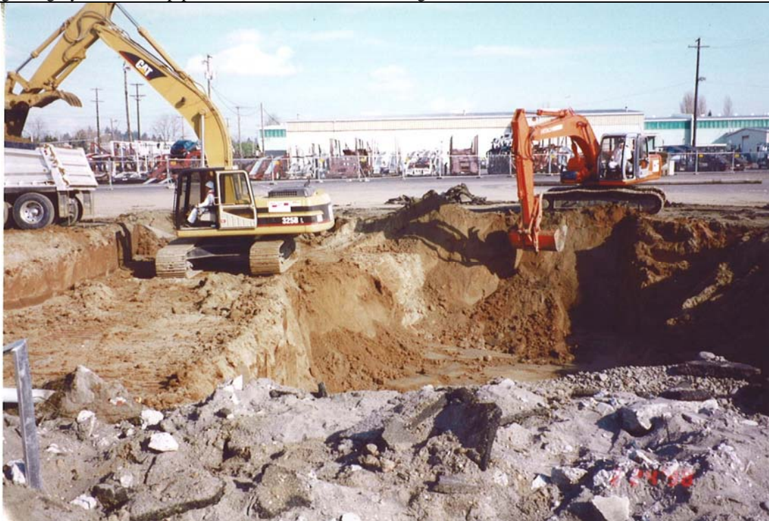
Photograph 32: Remedial excavation begins on east side of the former building 2220.
