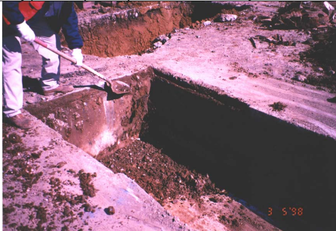
Photograph 16: Concrete pit in SMC concrete slab, looking northeast.
