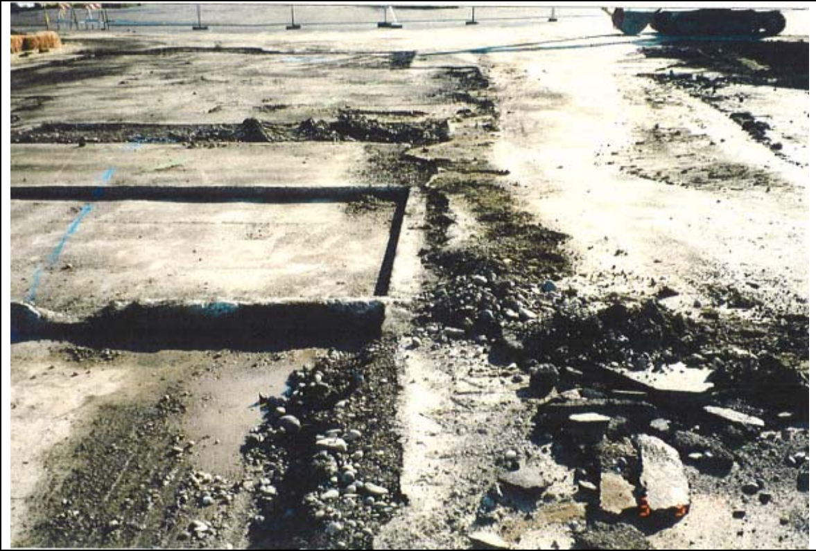
Photograph 13: Central part of the SMC concrete slab, looking east.
