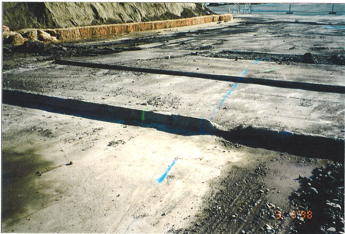
Photograph 12: Central part of SMC concrete floor slab, looking northeast.
