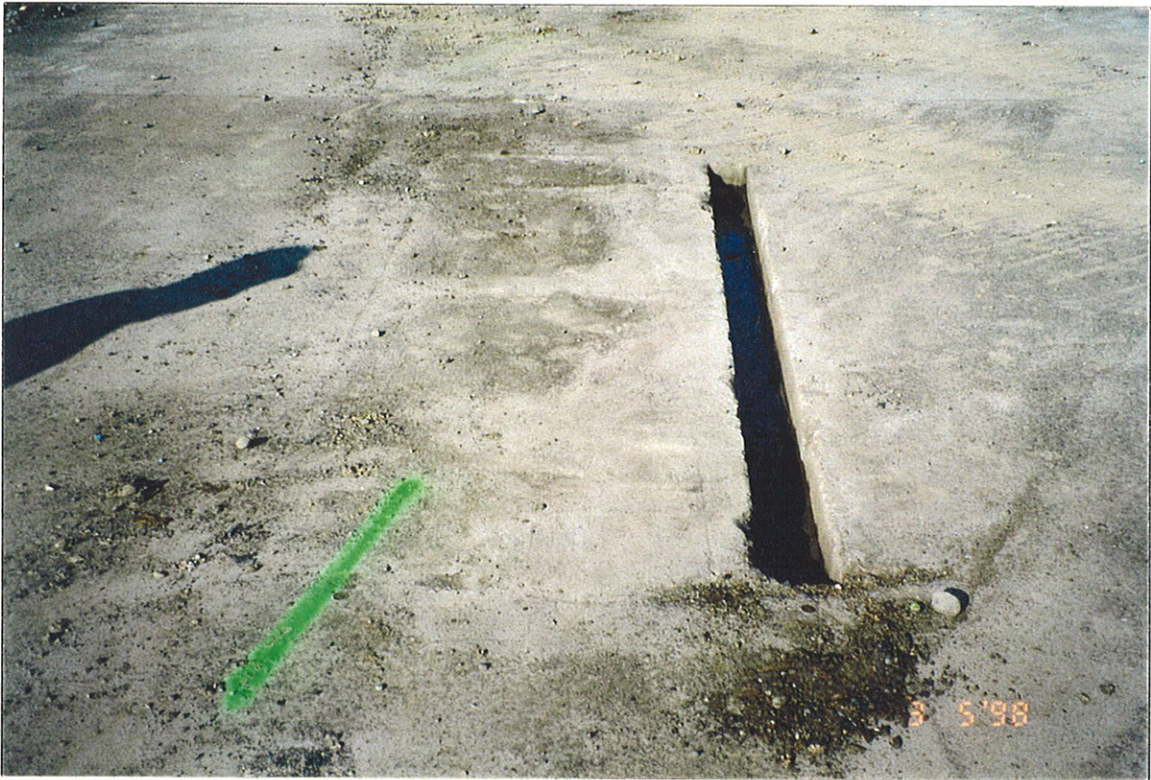
Photograph 10: Slot in central part of SMC concrete floor slab, looking west.
