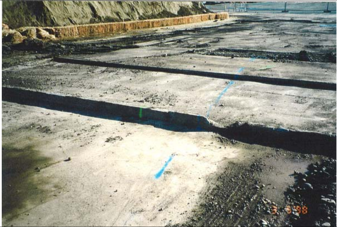
Photograph 12: Central part of the SMC concrete slab, looking north east.
