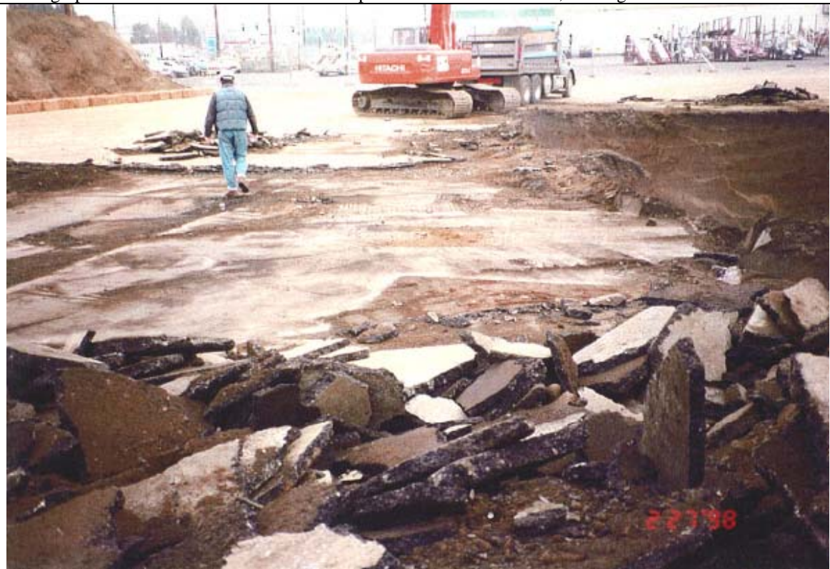
Photograph 4: Southwest corner and central part of SMC concrete slab, looking east.
