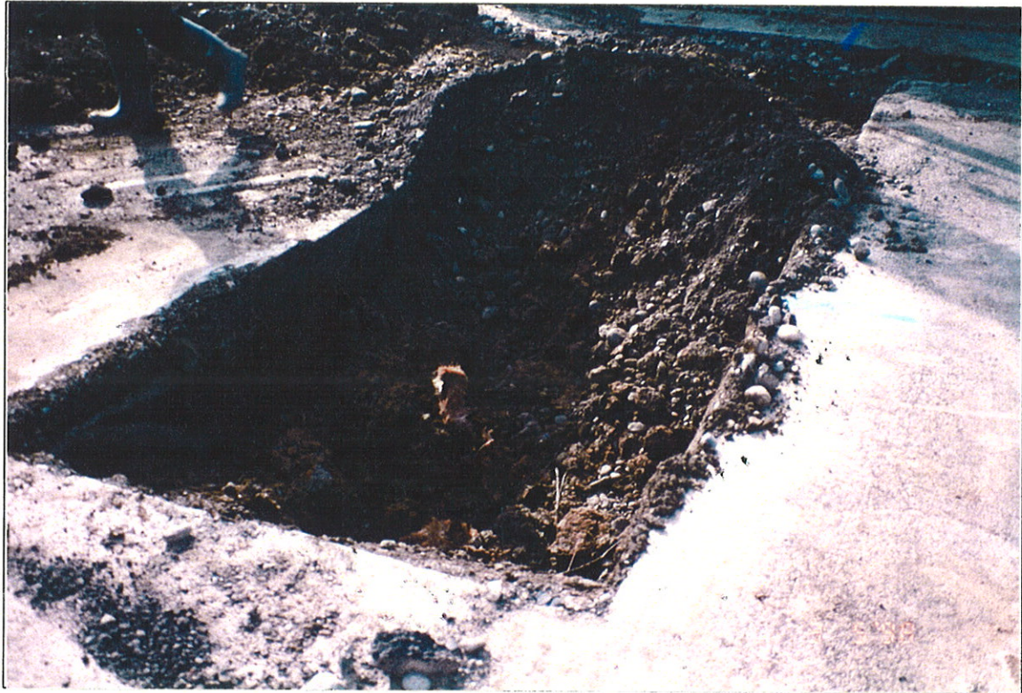
Photograph 15: Concrete vault/pit in eastern part of SMC concrete floor slab, looking south.
