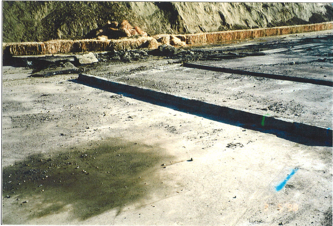
Photograph 11: Central part of SMC concrete slab, looking northeast.
