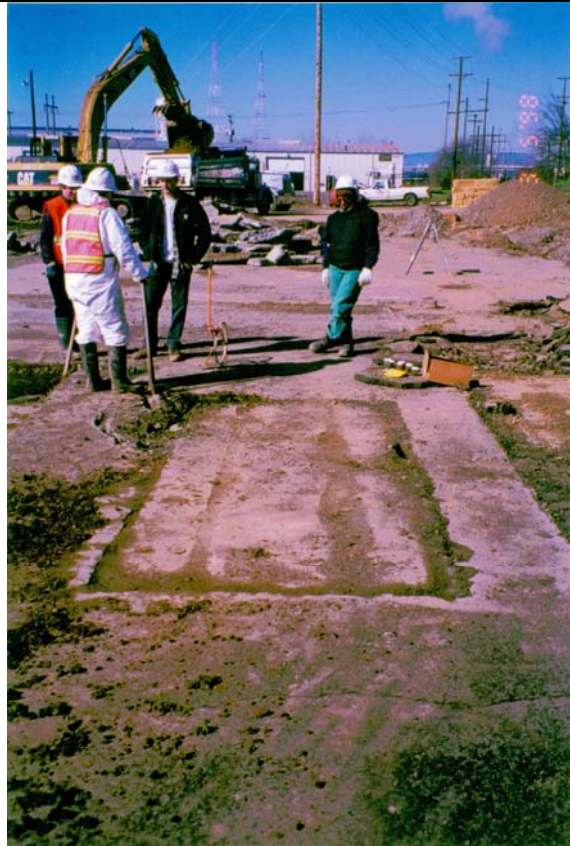
Photograph 24: Grooved concrete embedded in SMC concrete slab.
