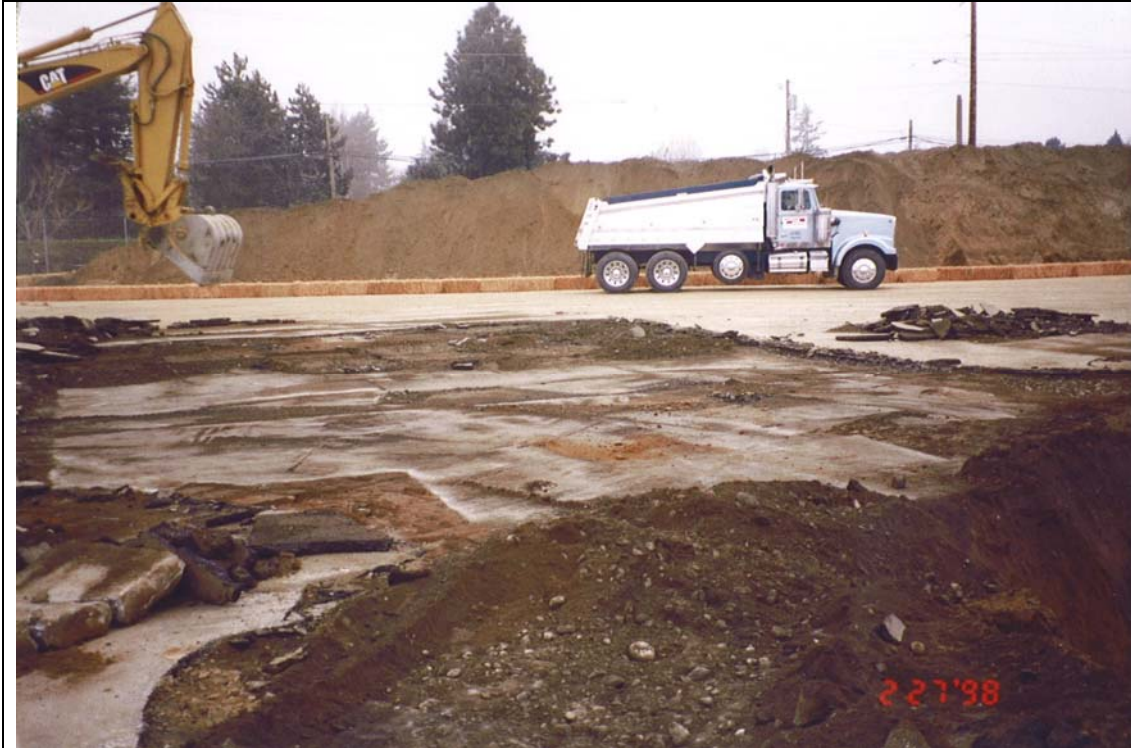
Photograph 33: Former SMC concrete slab discovered. Looking north.
