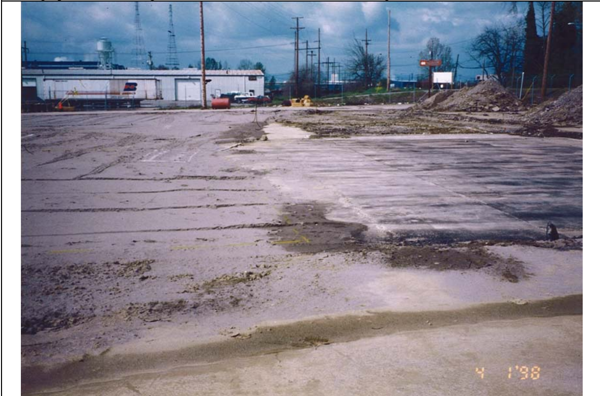
Photograph 42: Backfilling of remedial excavation complete. SMC slab in foreground.
