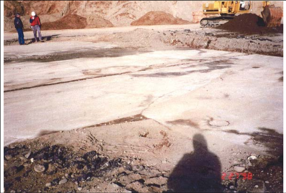
Photograph 3: Southern extension and central part of SMC concrete slab, looking northeast.
