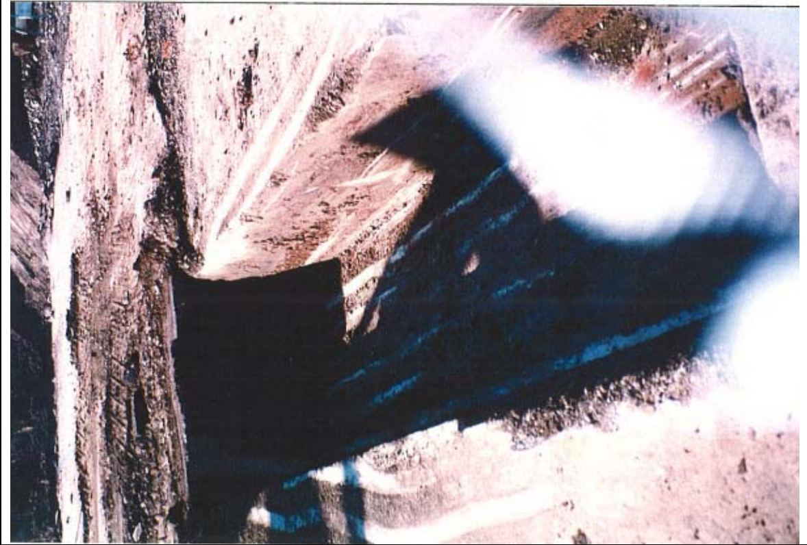
Photograph 17: Concrete pit in SMC concrete slab, looking south.
