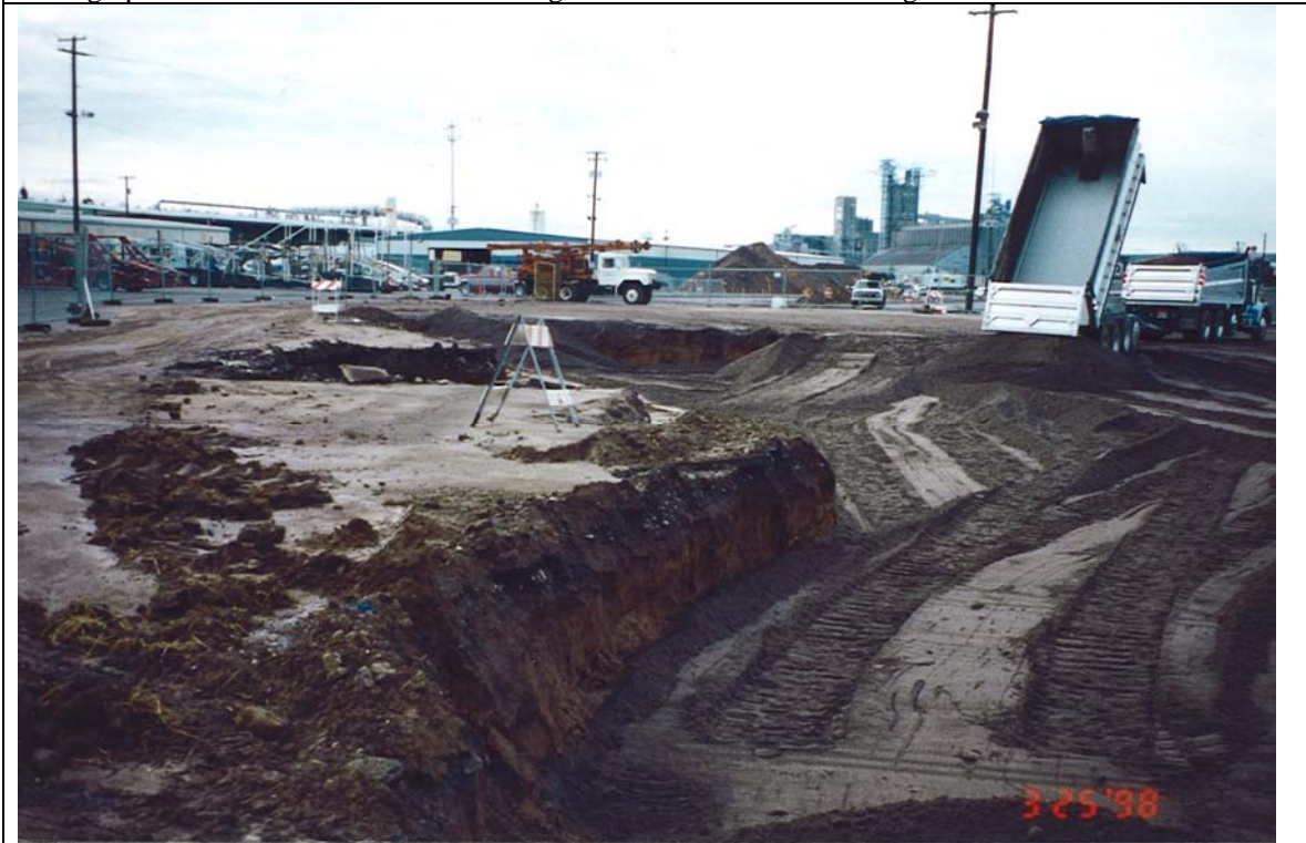
Photograph 40: Backfilling of remedial excavation. Looking south from SMC slab.
