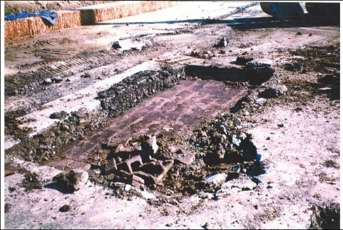
Photograph 25: Cinder blocks below the grooved concrete.
