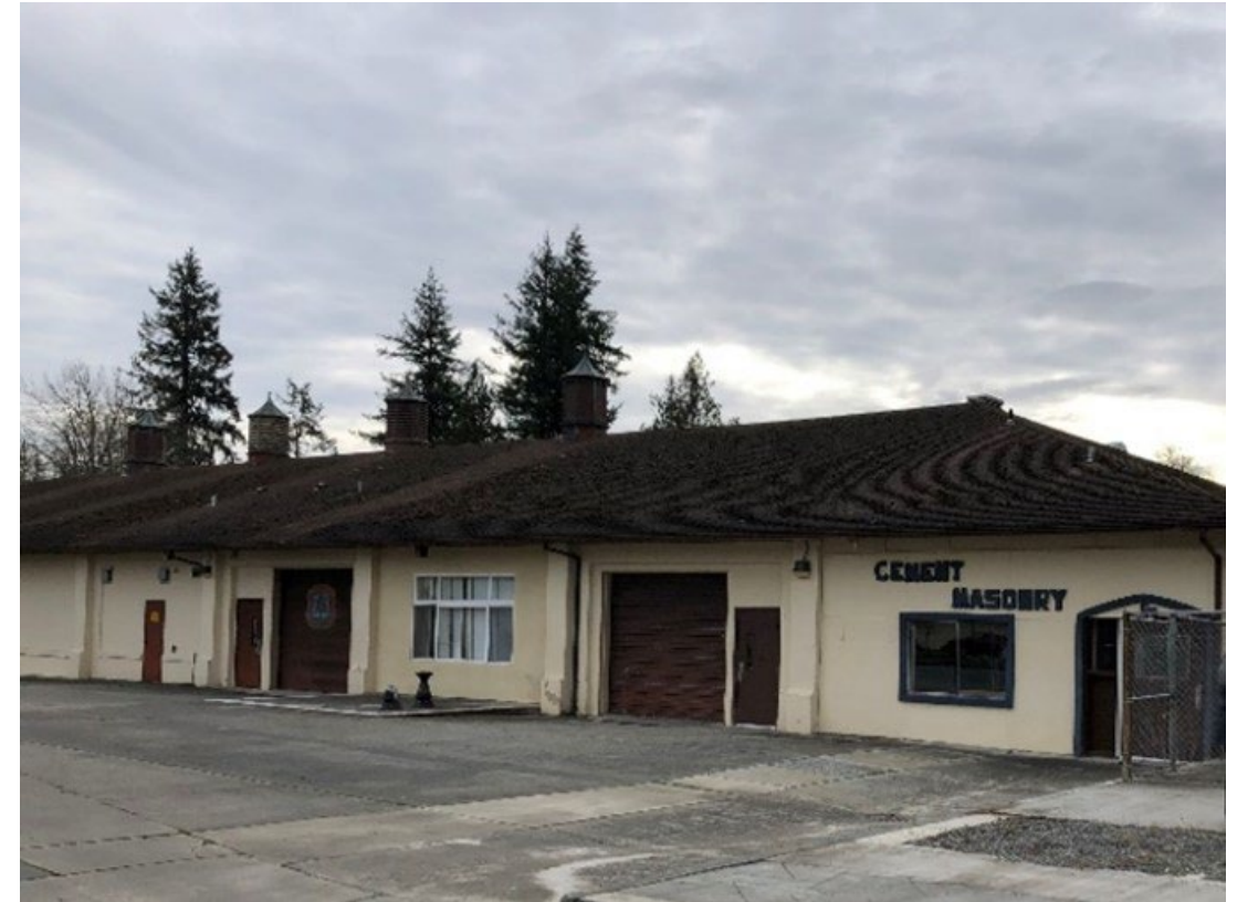
AOC 1, Former Laundry Building, January 2019
