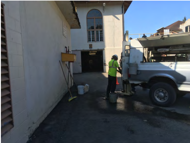
Photograph 3. Drilling boring B01, north of the Power House Building.
