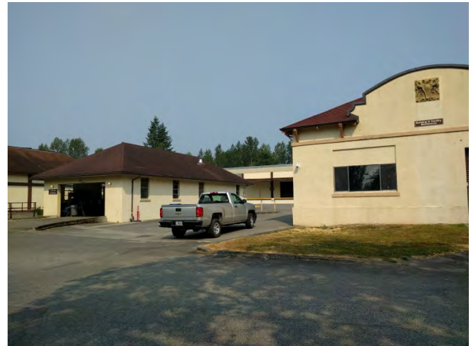
Photograph 2. View of the Maintenance Building area, looking northwest.
