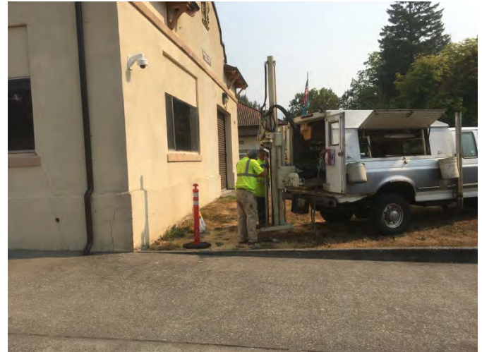
Photograph 4. Drilling boring B11, south of the Maintenance Building.
