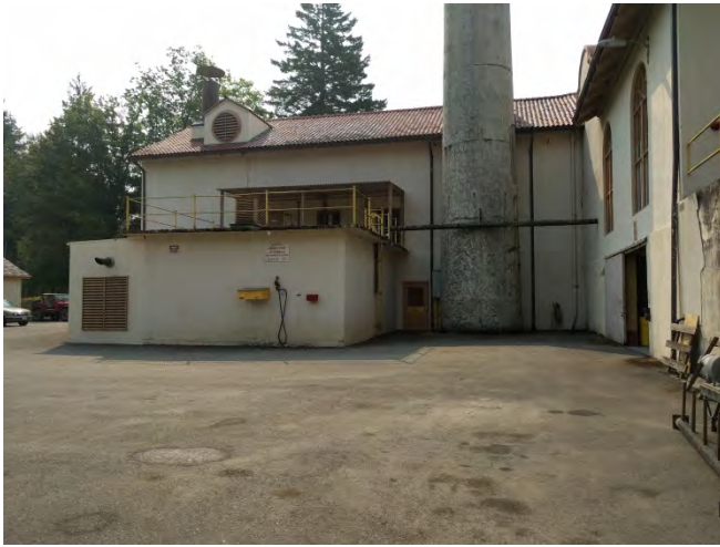
Photograph 1. View of the Power House Building area, looking southeast.
