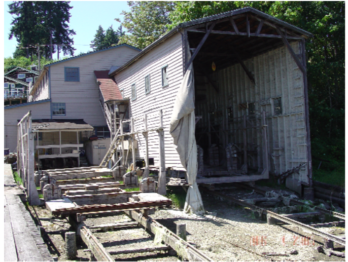
Eddon Boat Park boathouse and marine haul-out rails.
