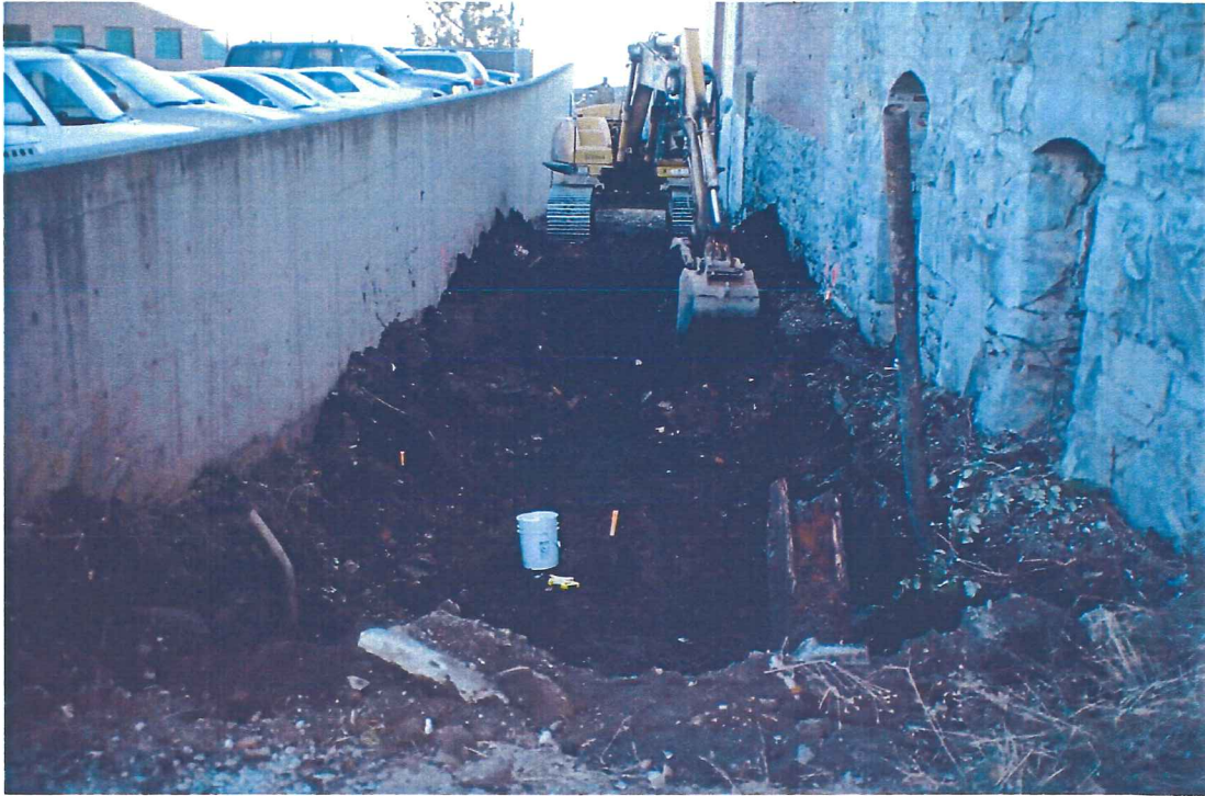
Photograph 5 – View to east of CNA remedial excavation.
