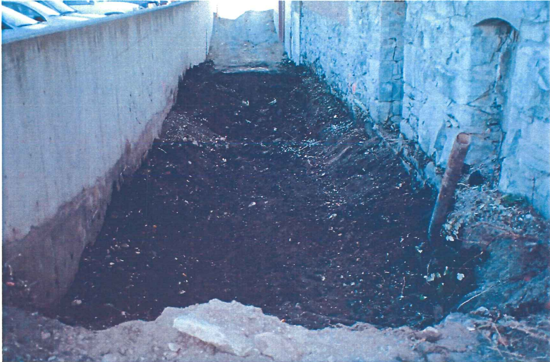
Photograph 7 – View of CNA remedial excavation following cleanup action.
