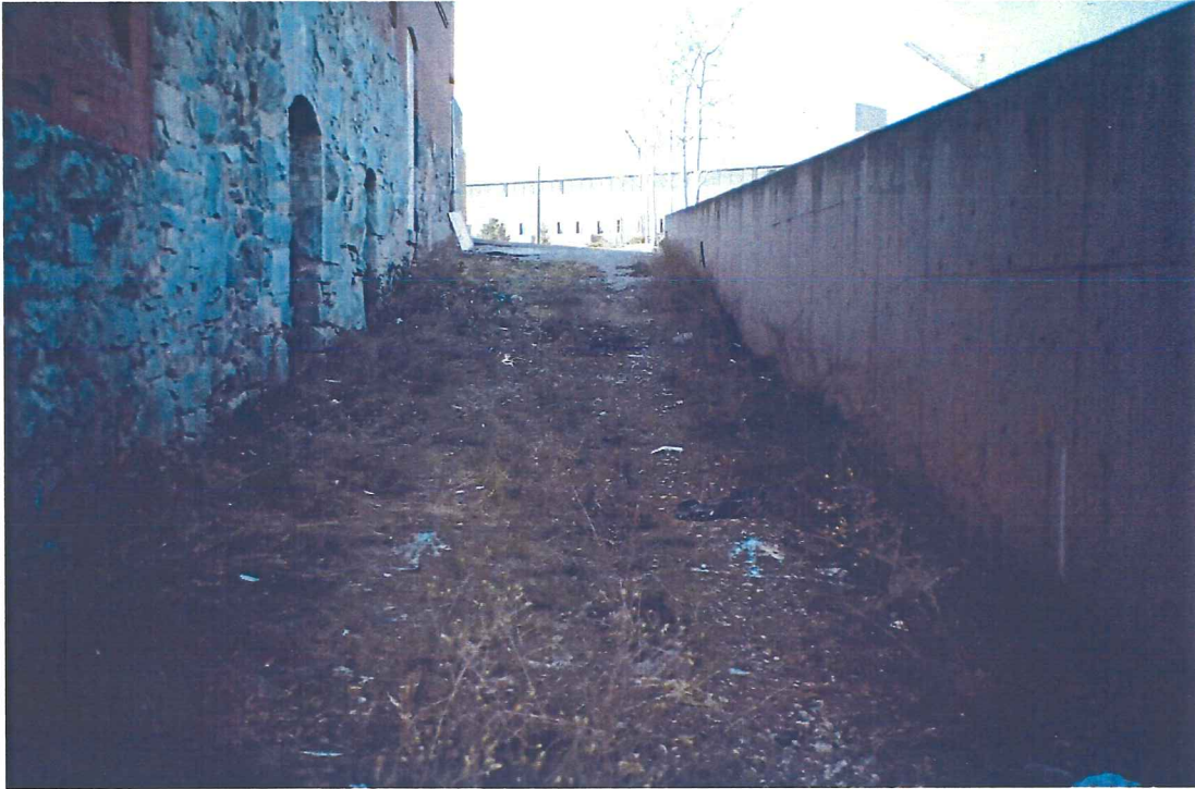
Photograph 1 – View to west of north alley and CNA and WNA remedial excavation areas (pre-remedial).
