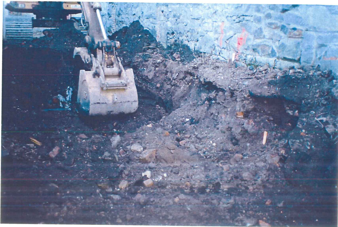
Photograph 6 – View of south sidewall of CNA remedial excavation and building foundation.
