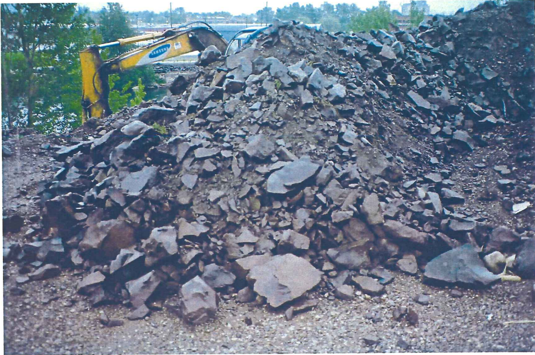
Photograph 15 – View of fractured basalt material stockpile from riverside pedestrian walkway excavation, prior to screening operations.
