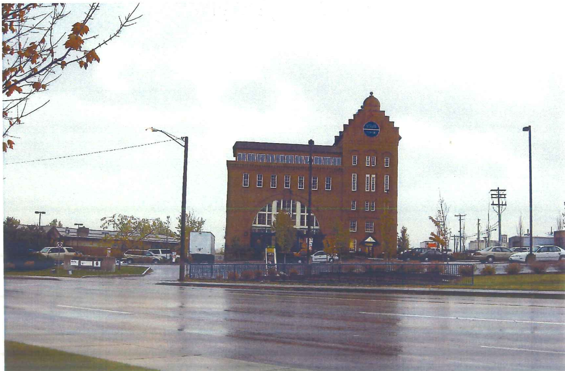
Photograph 24 – View to east of Schade Brewery western parking area from across East Trent Avenue.
