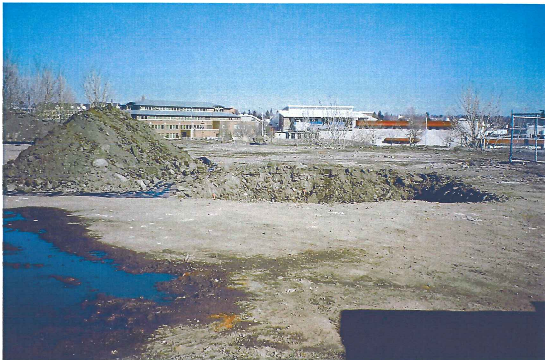
Photograph 9 – View to north of TP5 remedial excavation.
