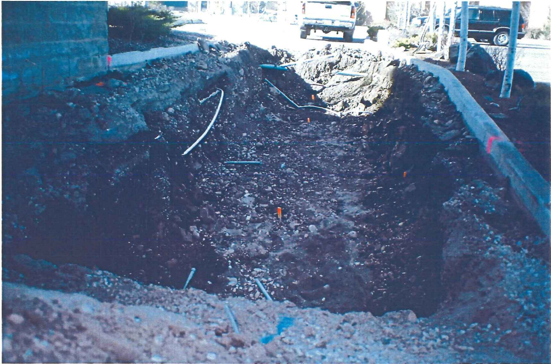
Photograph 3 – View to west of WNA remedial excavation.
