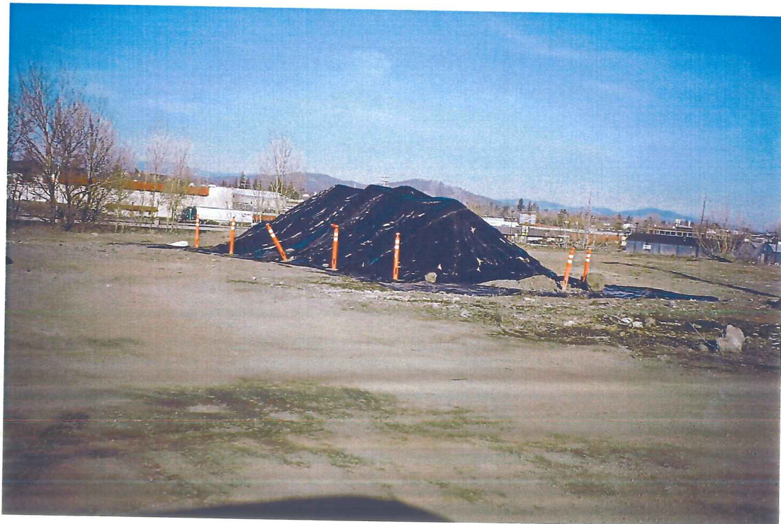
Photograph 12 – View of temporary waste soil stockpile.
