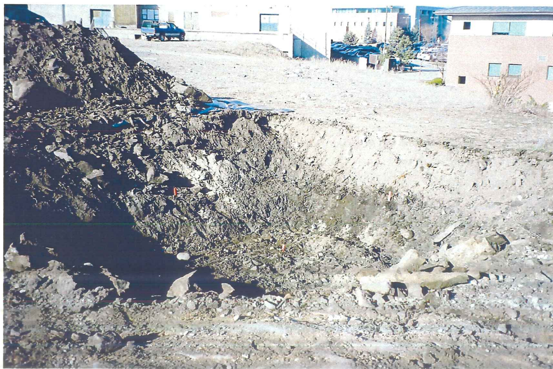
Photograph 10 – View to west of TP7 remedial excavation.
