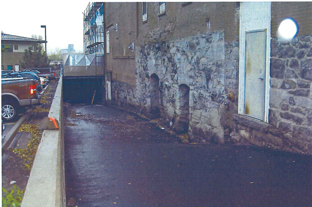
Photograph 29 – View of north alley improvements with asphalt cover.
