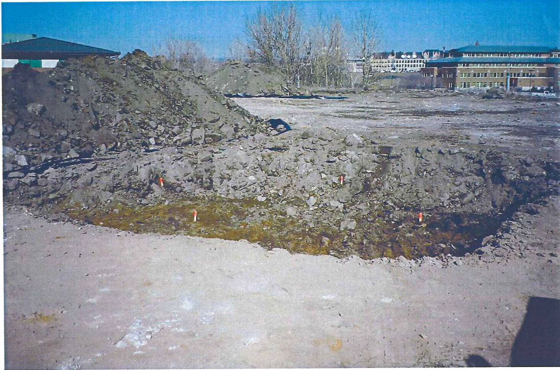
Photograph 11 – View to north of TP5 (foreground) and TP7 (background) remedial excavations.
