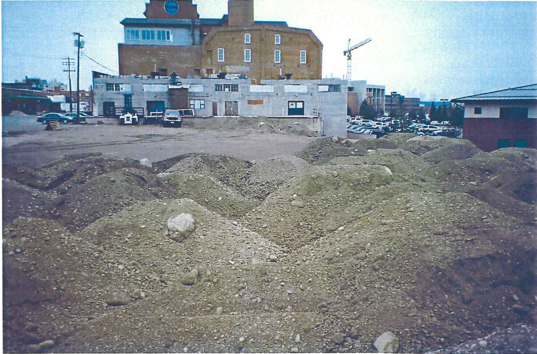
Photograph 17 – View to west of imported soil fill used to raise eastern parking area elevation.
