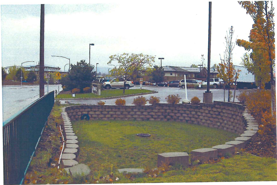
Photograph 25 – View to northeast of storm water swale located in northwest corner of western parking area.
