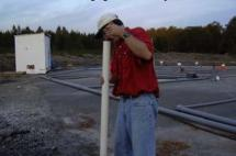
2) Place tube on table and expose the first segment by pulling on the bottom end of the PFM.
