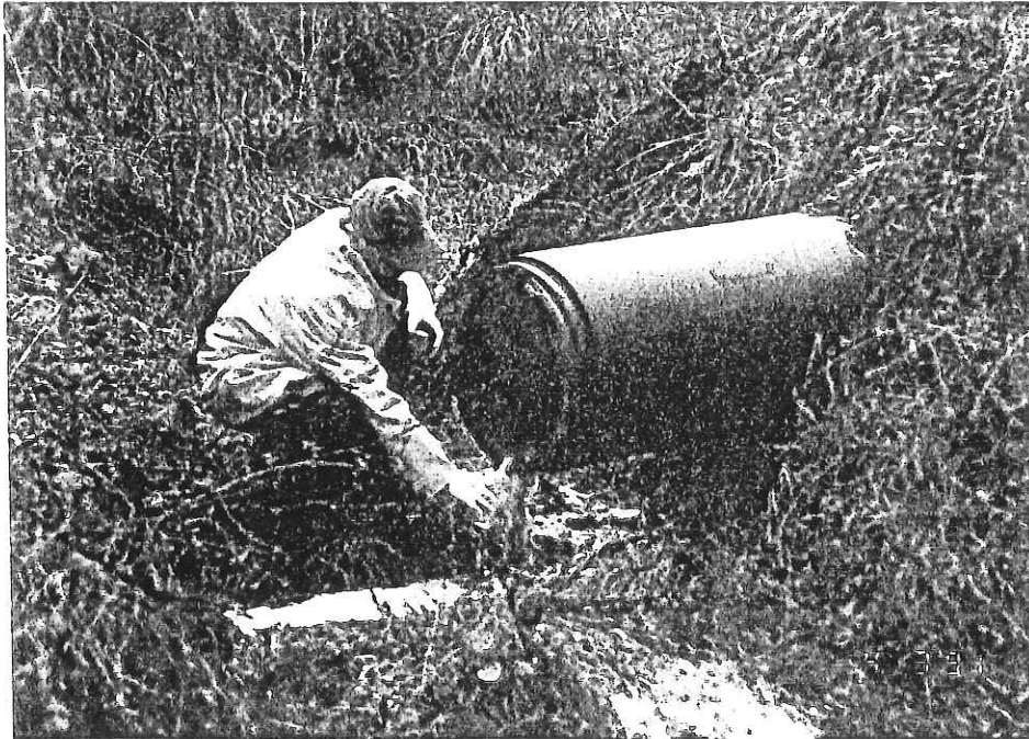
FIGURE 5 SW1 CULVERT PIPE WHICH RUNS NORTH & SOUTH BELOW THE FILL
