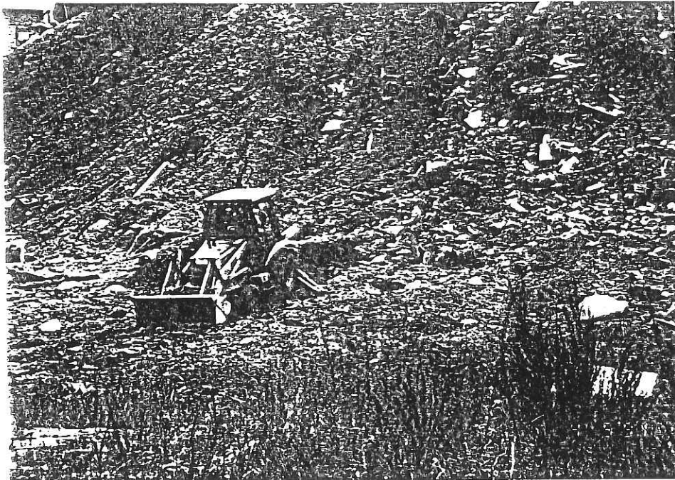
FIGURE 3 TP8 DUG INTO LOWER FACE OF THE FILL
