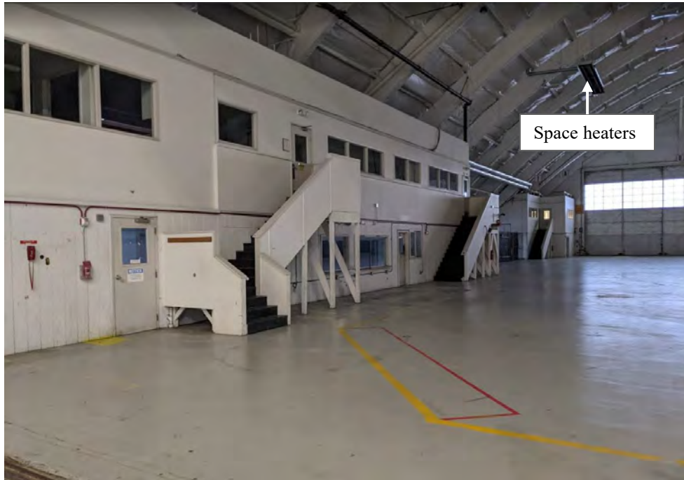
Photograph 5. C-1 Hangar offices located on west-southwest side of building. Sample locations SS-1, -2, -3, IA-2, and DP-2 were located in this area.
