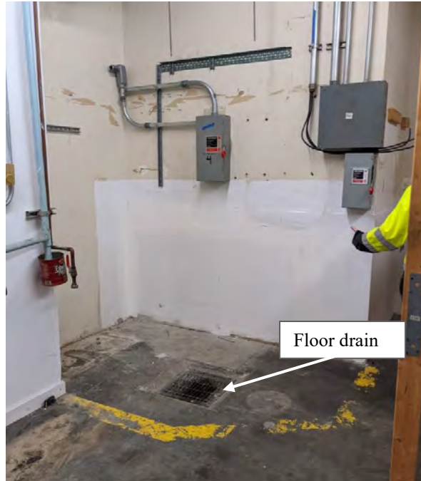
Photograph 3. Floor drain identified in C-1 Building near in office areas near sample location IA-9. No strong odors were observed.
