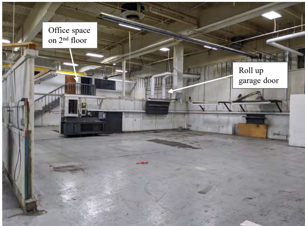
Photograph 4. Main workshop area in C-1 Building with view of 2 nd floor office space. Sample location for IA-12. Roll up garage doors lead to outdoor, gated parking lot.
