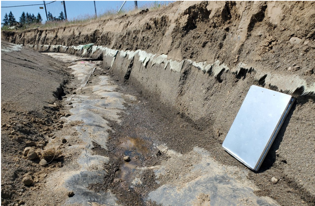
June 22 nd , 2023: Detail of sand layer atop Landfill cover liner.
