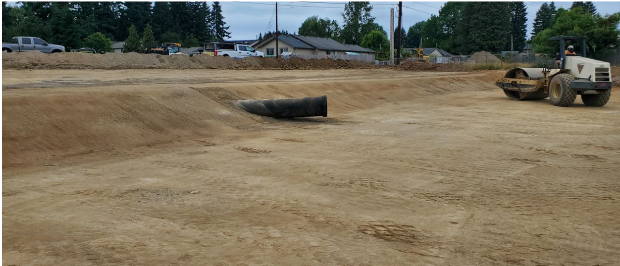
June 26 th , 2023: Installation of drain rock around exposed corrugated plastic drain pipes.
