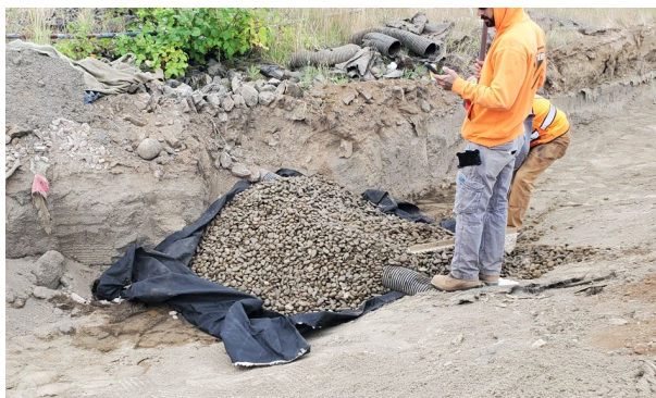
June 26 th , 2023: Installation of drain rock around exposed corrugated plastic drain pipes.
