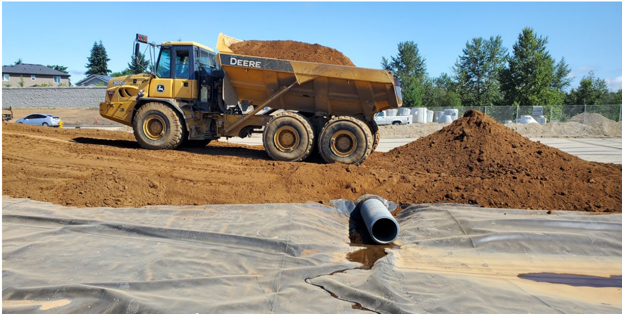
June 28 th , 2023: Placement of cover layer soil.
