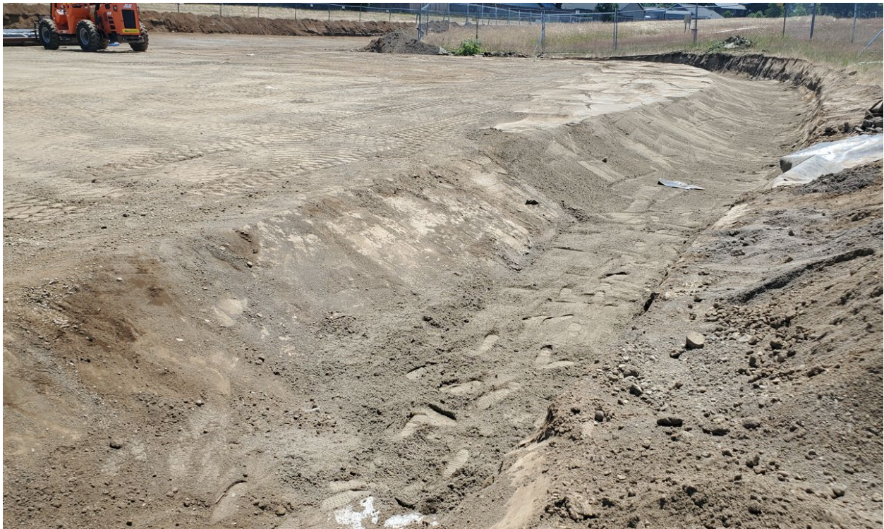
June 23 rd , 2023: Sand layer placed atop exposed existing Landfill cover liner.
