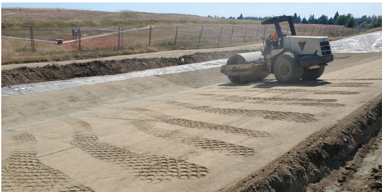
June 15 th , 2023: Preparation of subgrade for liner deployment.
