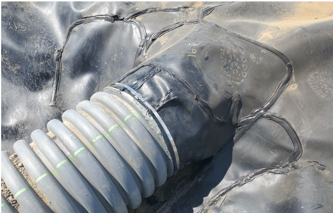
June 27 th , 2023: Storm collector pipe penetration HDPE boot.
