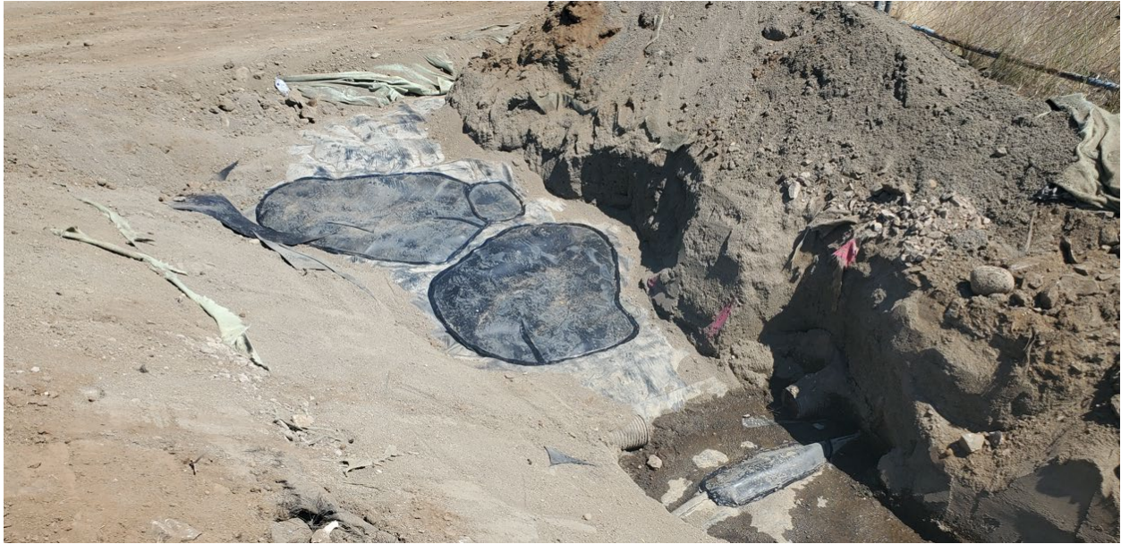
June 22 nd , 2023: Repairs to existing Landfill cover liner.
