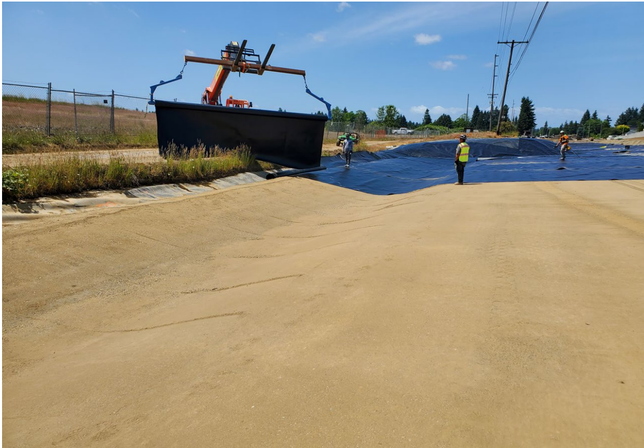
June 15 th , 2023: Deployment of geomembrane liner over prepared subgrade.
