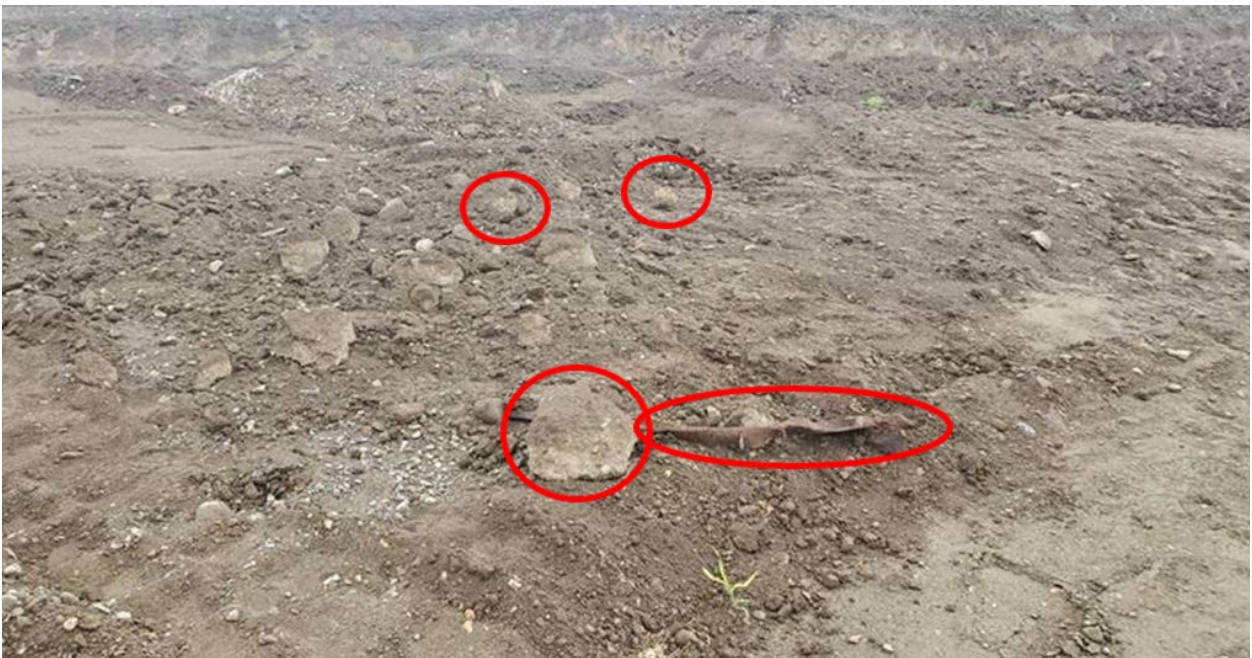
Photo 2 - Soil includes rocks, wood debris, and metal.
