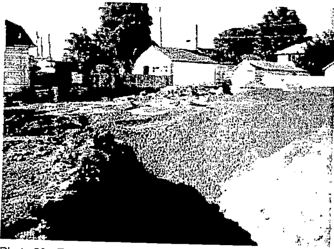
Photo 29 - Excavation during backfill placement - View southwest
