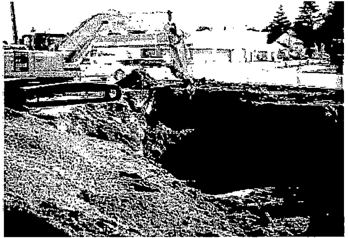
Photo 16 - Backfill placement - View northeast
