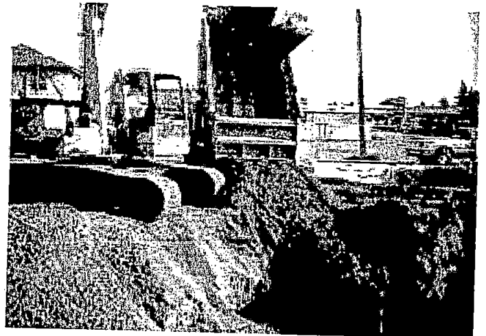
Photo 28 - Backfill placement - View north
