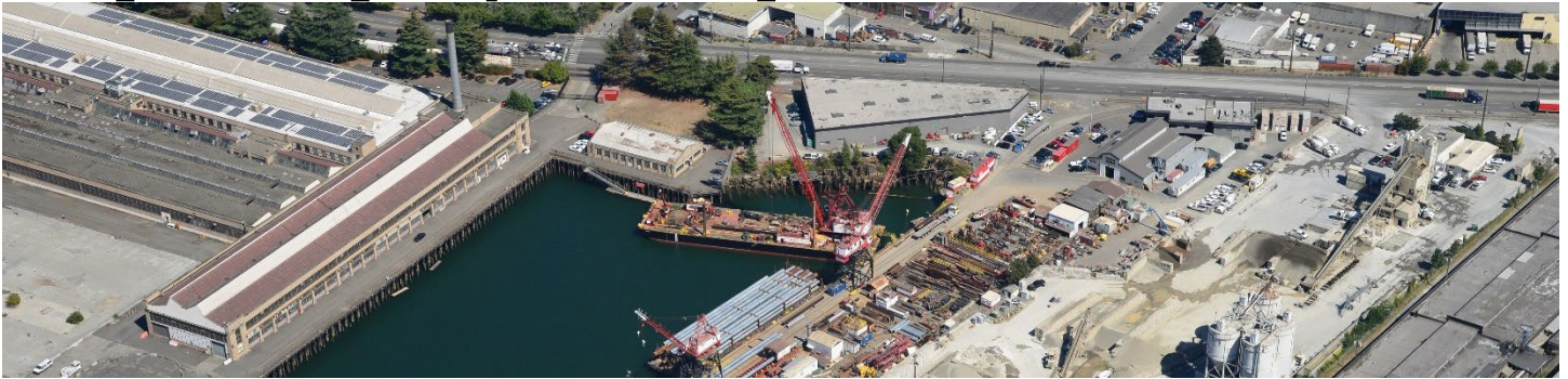
Aerial View of Snopac Property
