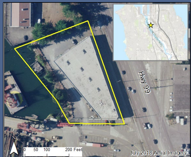
Aerial View of Snopac Property
