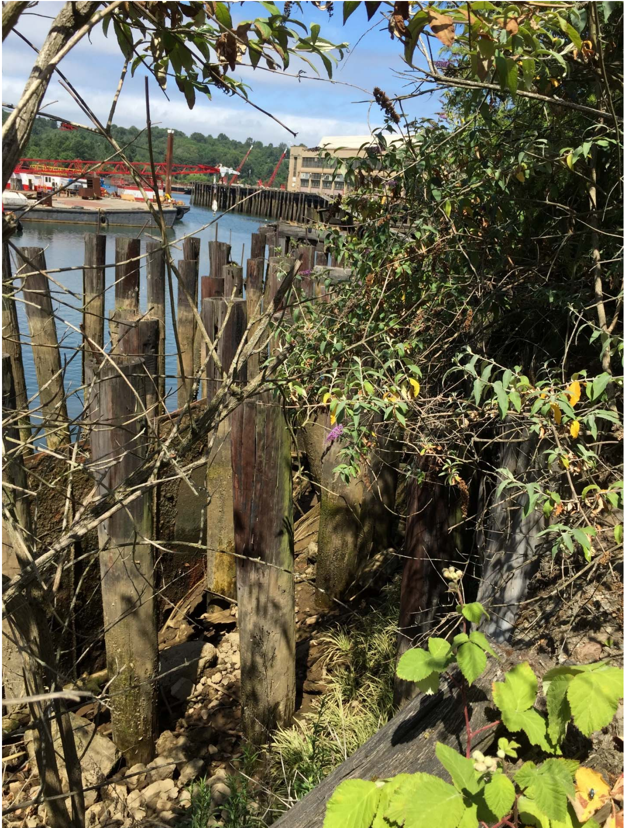
Top of bank showing steel retaining wall and pilings.
