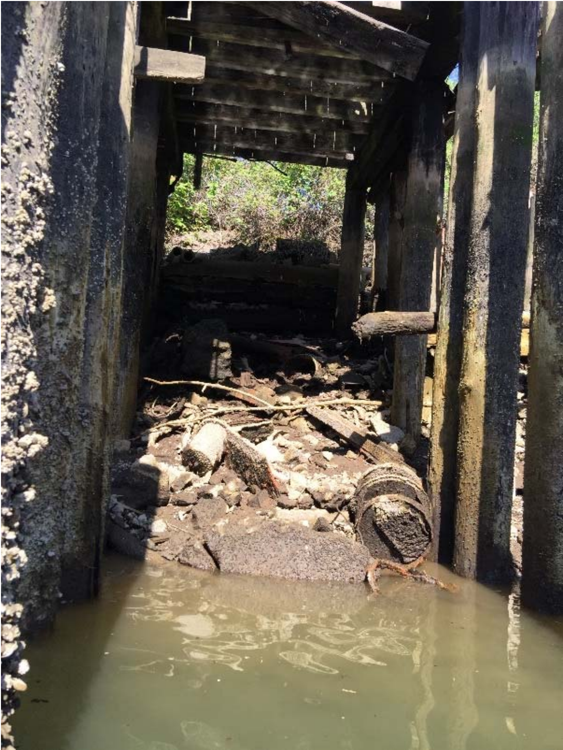
Shoreline and bank beneath remaining dock structure.
