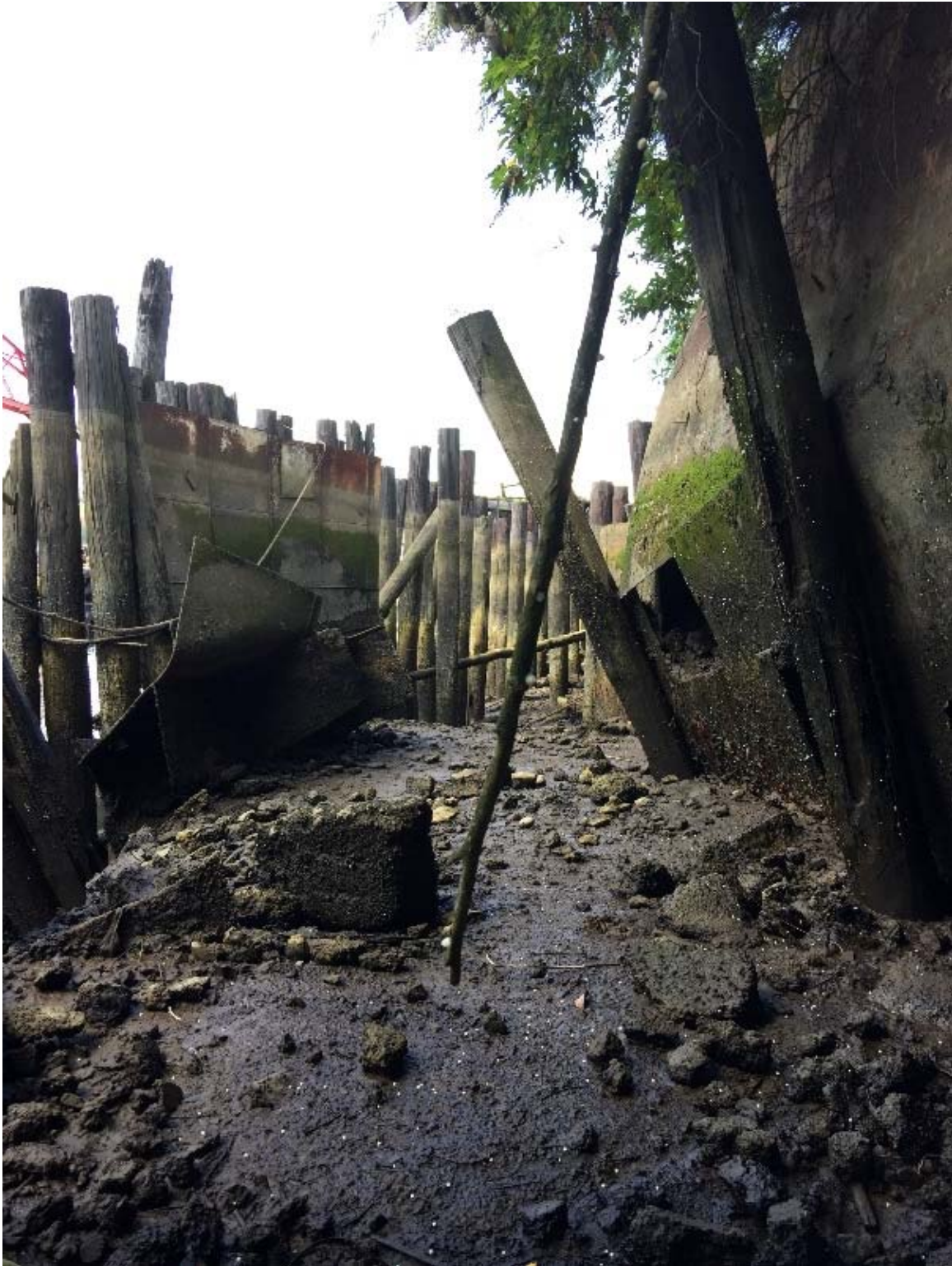
Shoreline and retaining wall with supporting pilings.
