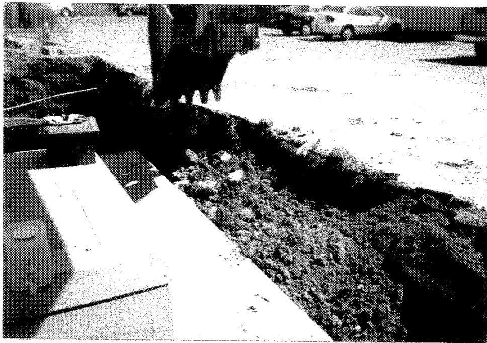
Start of excavation on south side of vault.
