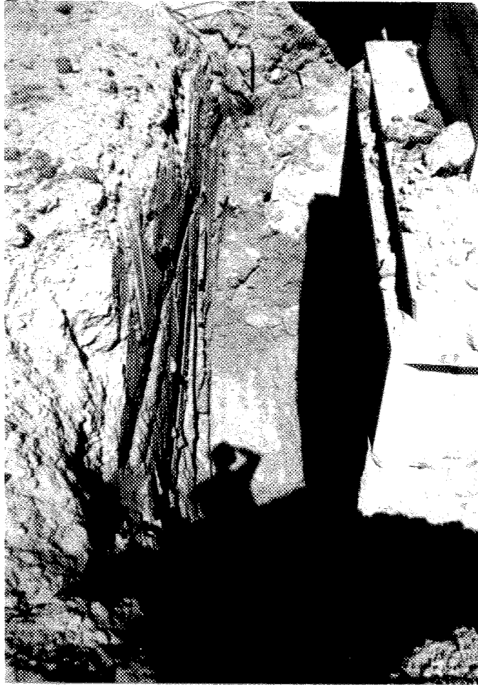
West end of vault excavated to +/- 12 1/2' bgs. Soil sampling around vault at non-detect level. East end of excavation lined with poly prior to backfill. Vault area filled with slurry.
