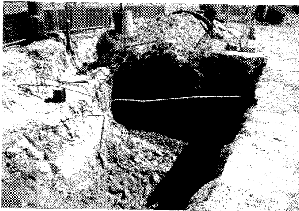
East end of trench was excavated to an approximate depth of 9 ½' x 20' wide. Note water line at top of photograph.
