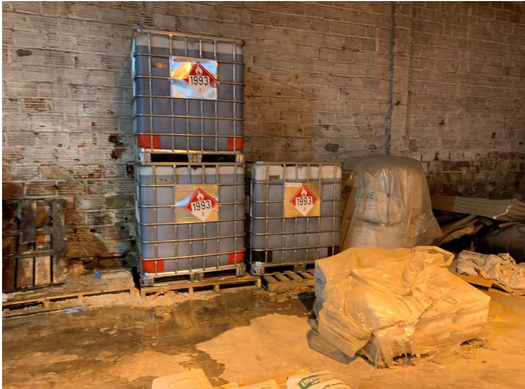
Photo 7: Storage of flammable pep set binder system in Bay 2 (rainwater from leaks in ceiling visible).
