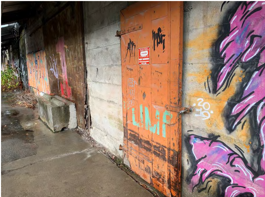
Photo 13: View of one of three fire suppression system pump rooms (not accessible to Ramboll) located to the south of warehouse.
