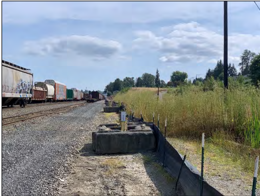
Photograph 2. Well BP-03S location
