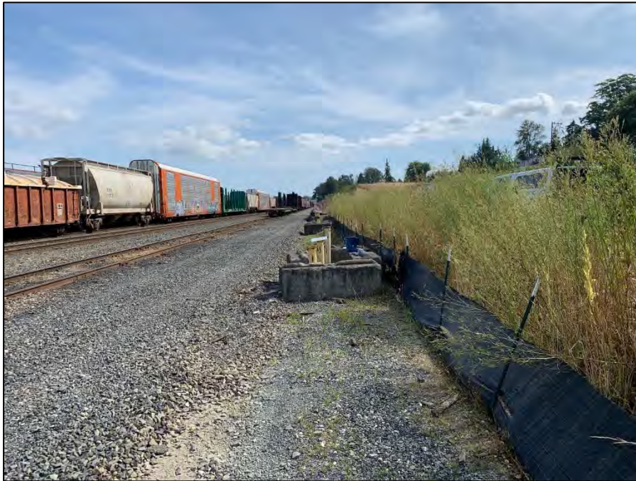
Photograph 2. Well BP-05D location
