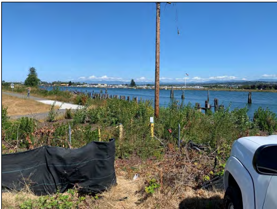
Photograph 2. Well PZ-3B location
