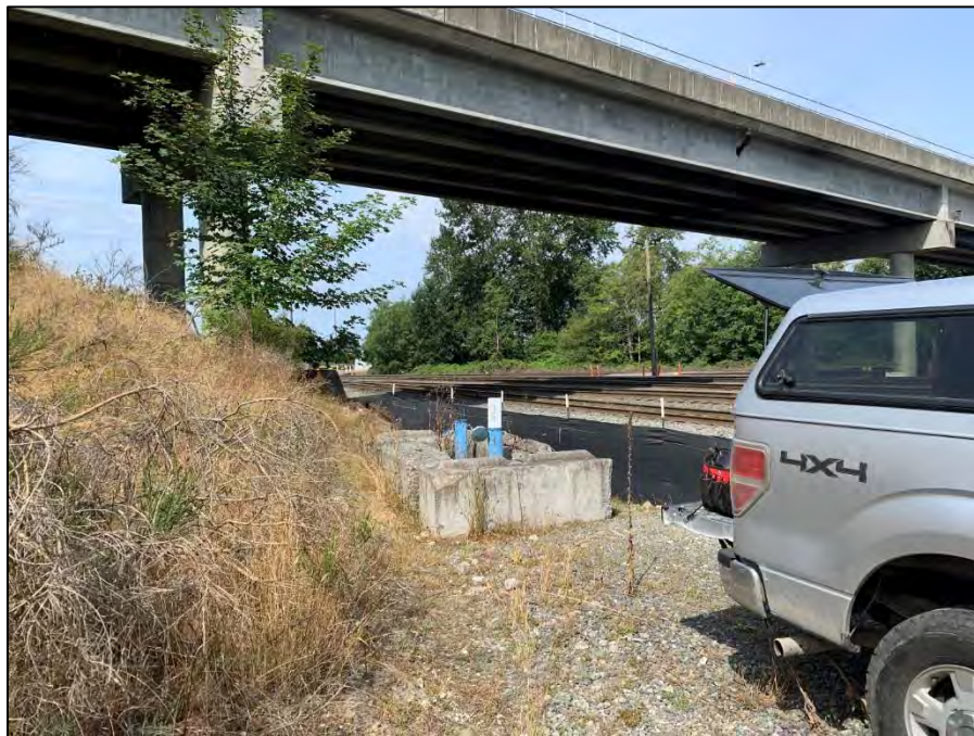
Photograph 2. Well BP-02D location
