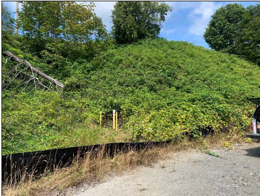
Photograph 2. Well LLMW-36D location
