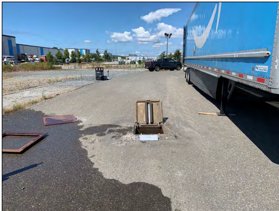
Photograph 2. Well PZ-1B location
