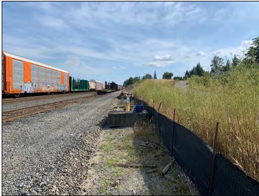
Photograph 2. Well BP-06D location
