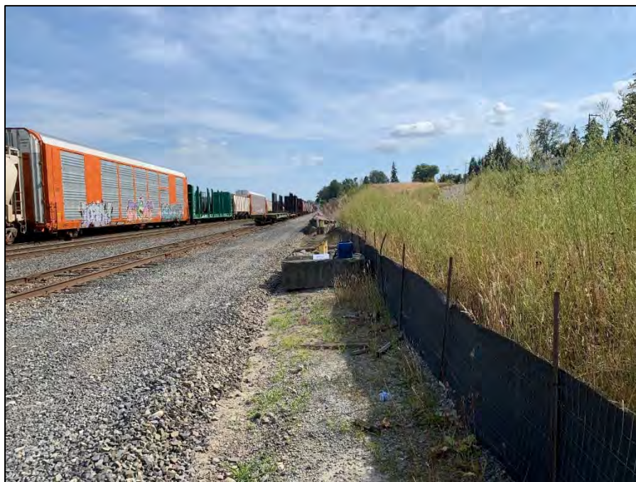
Photograph 2. Well BP-06S location
