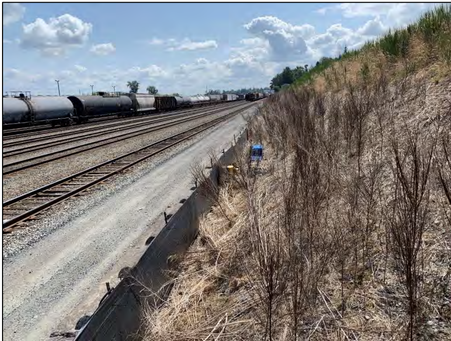
Photograph 2. Well BP-08D location
