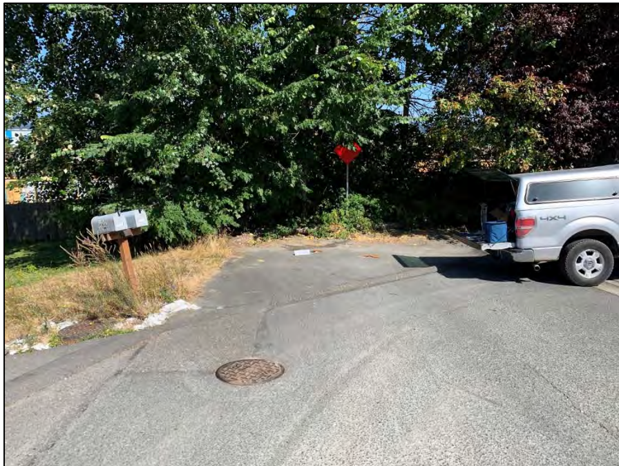
Photograph 2. Well LLMW-33D location
