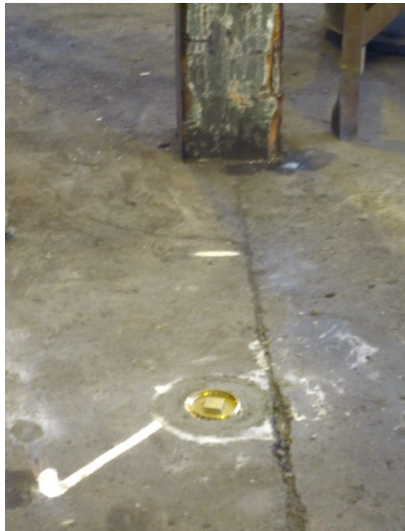
Photograph 2. Completed Vapor Point with Protective Brass Cover.
