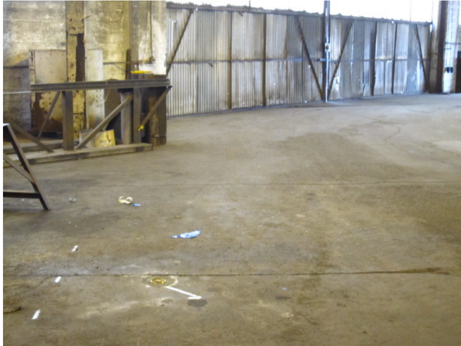
Photograph 3. Alternative View of Completed Soil Vapor Point.
