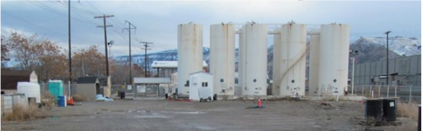
Coleman Oil Biodiesel Spill
