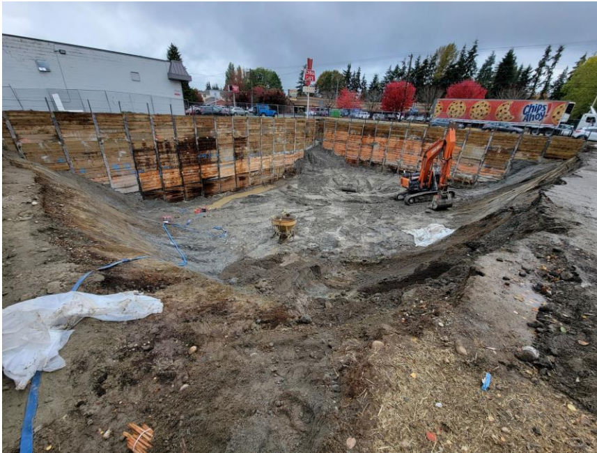
Photograph 1. Final excavation extends facing northwest
