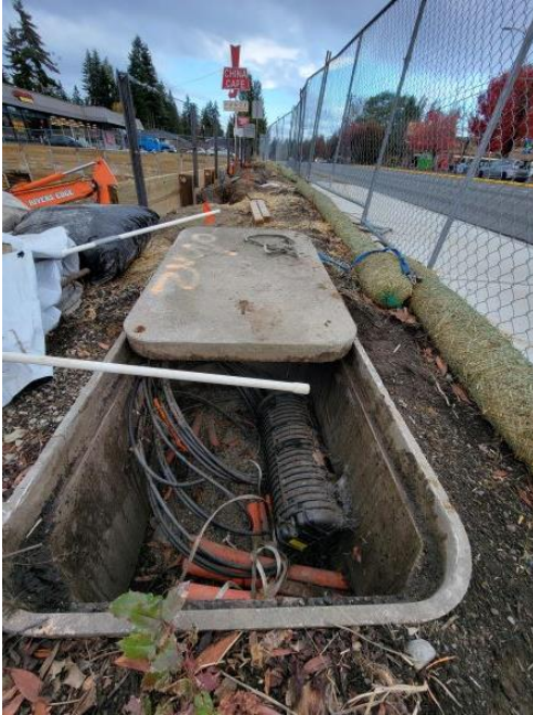
Photograph 3. Area between north shoring wall and the sidewalk right-of-way
