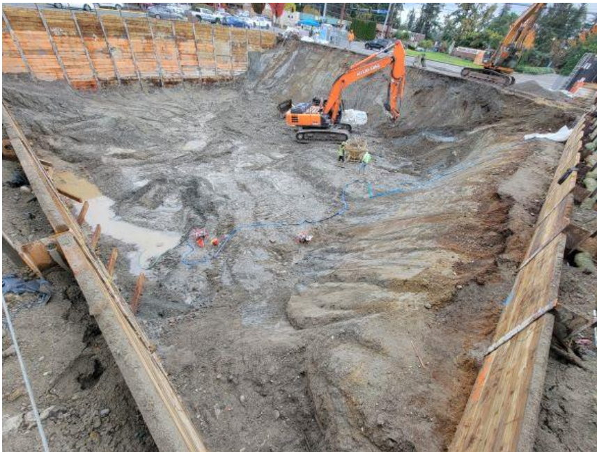
Photograph 2. Final excavation extends facing northeast
