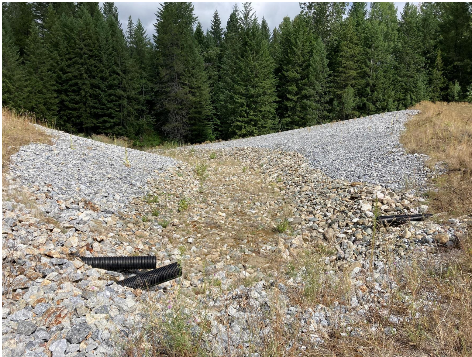
Photo 8: Drainage ditch 2A coming off TDF-2
