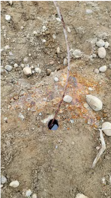
Photo 3. Uncovered inlet of UST 3 with sample tubing showing the burgundy stain and material that sticks to the side of the tubing.
