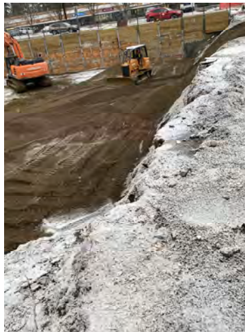
Grading Import Material 12" Lift
