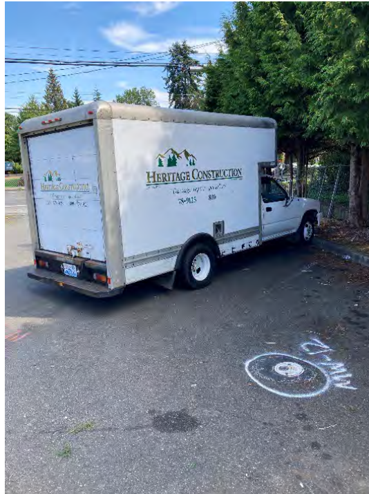
Photo 3: Box truck parked in site southeast corner.
