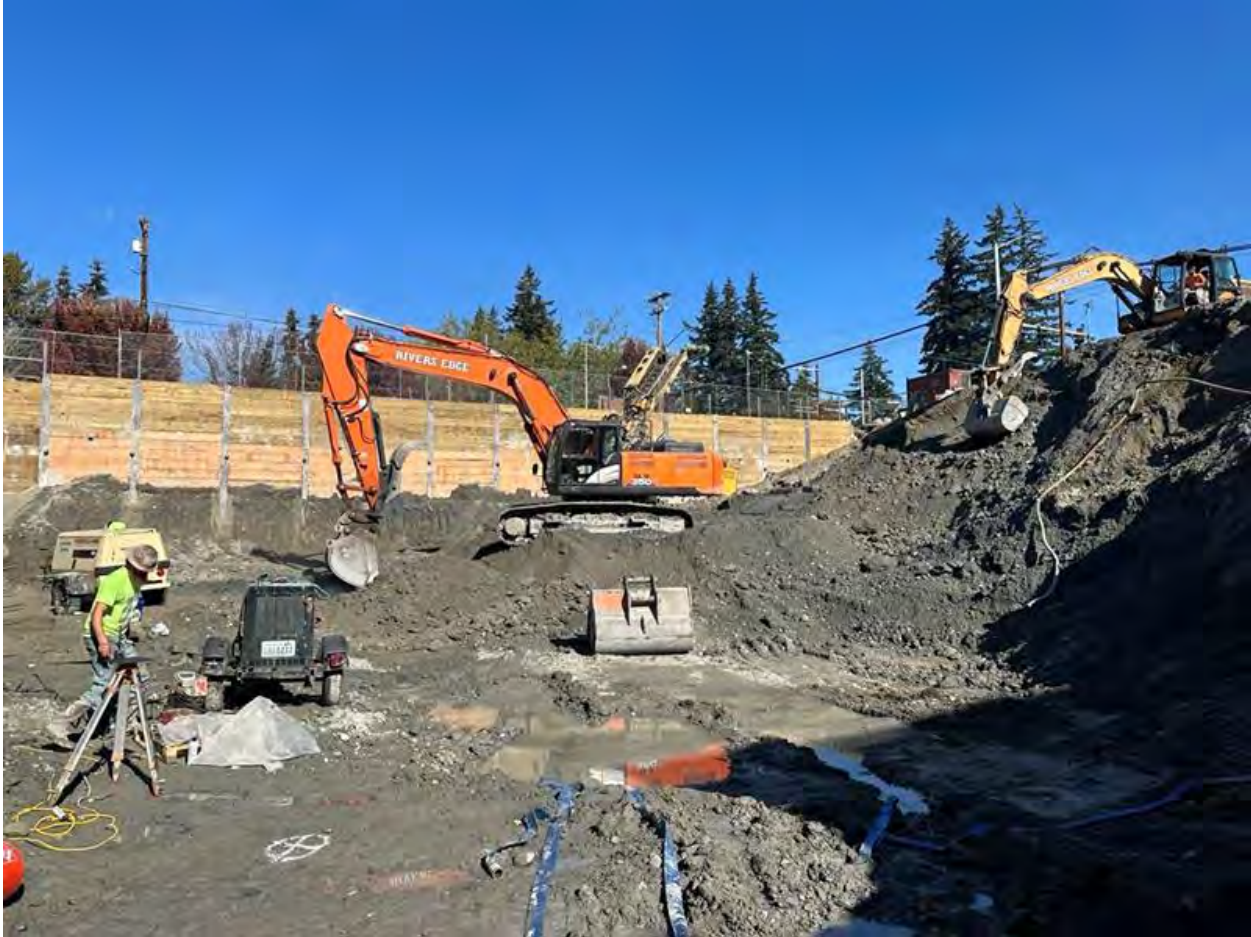
Photo 1: Excavation progression at elevation ~431 facing North.
