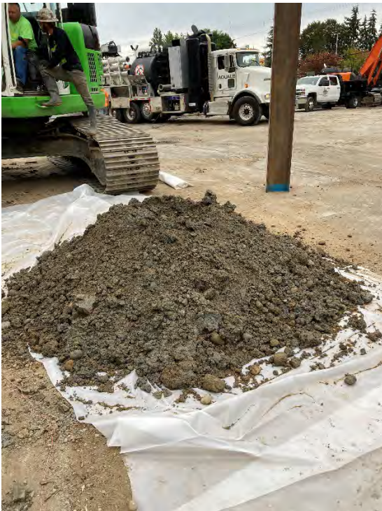
Photo 2: Soldier pile installation cuttings being placed on plastic.
