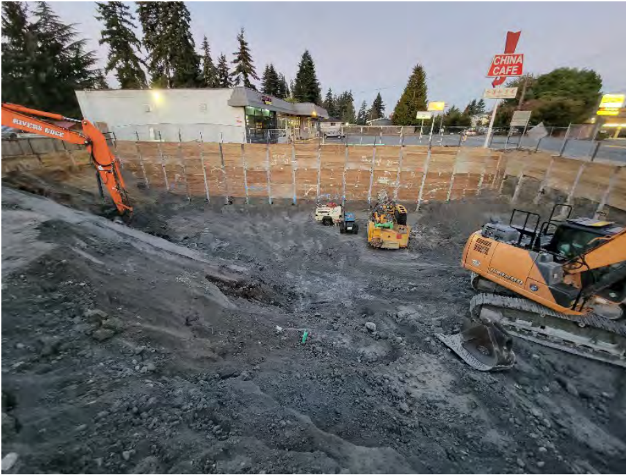
Photo 1: Current excavation extents at the beginning of the day, looking west.
