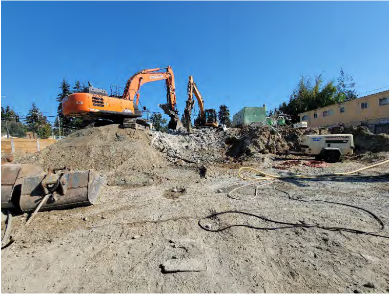
Figure 1 REES removing slab and footing of former building
