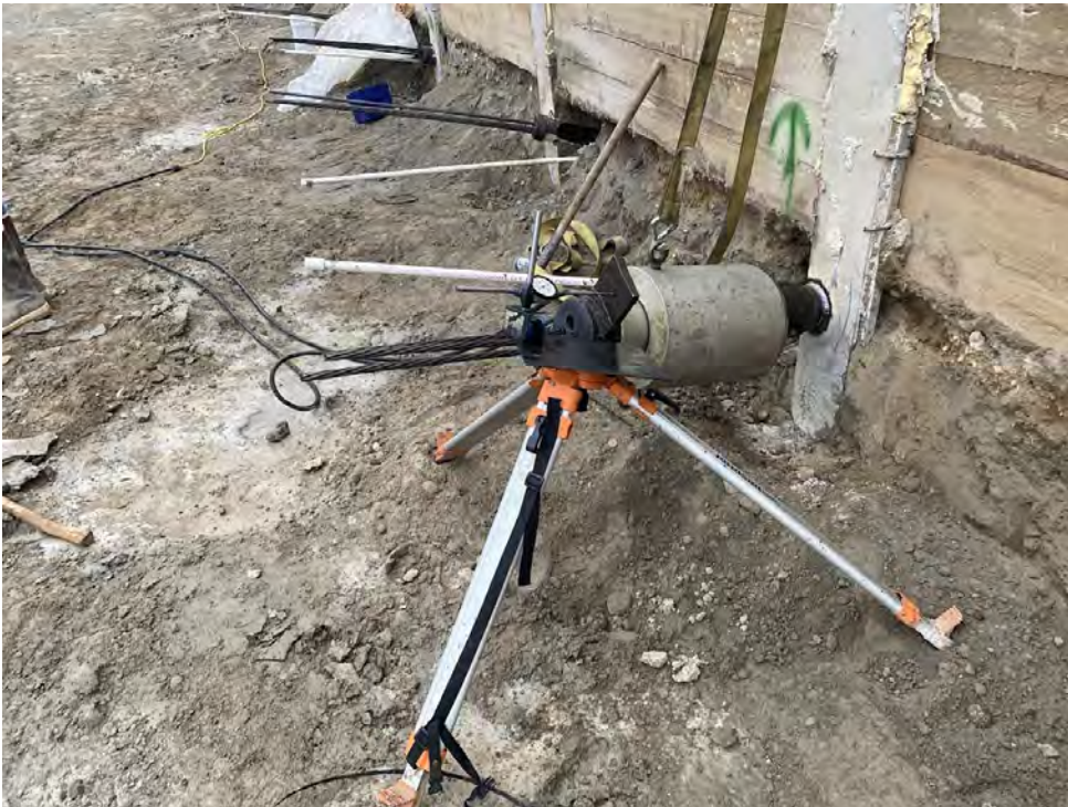
Photo 4: Rig setup to test tieback in west wall.
