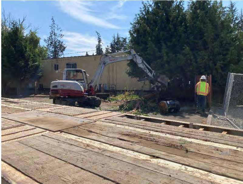
Photo 1: Brush and dumpster area demolition and clearing, viewing south.
