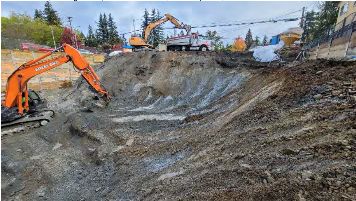
Figure 1. Looking northeast, showing the eastern sidewall of the excavation.
