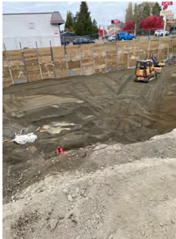
Grading 1 st 12" Lift @ 18' BG
