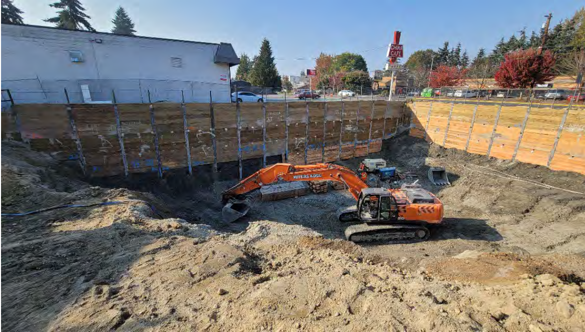
Figure 2. The site towards the end of the day, facing northwest.
