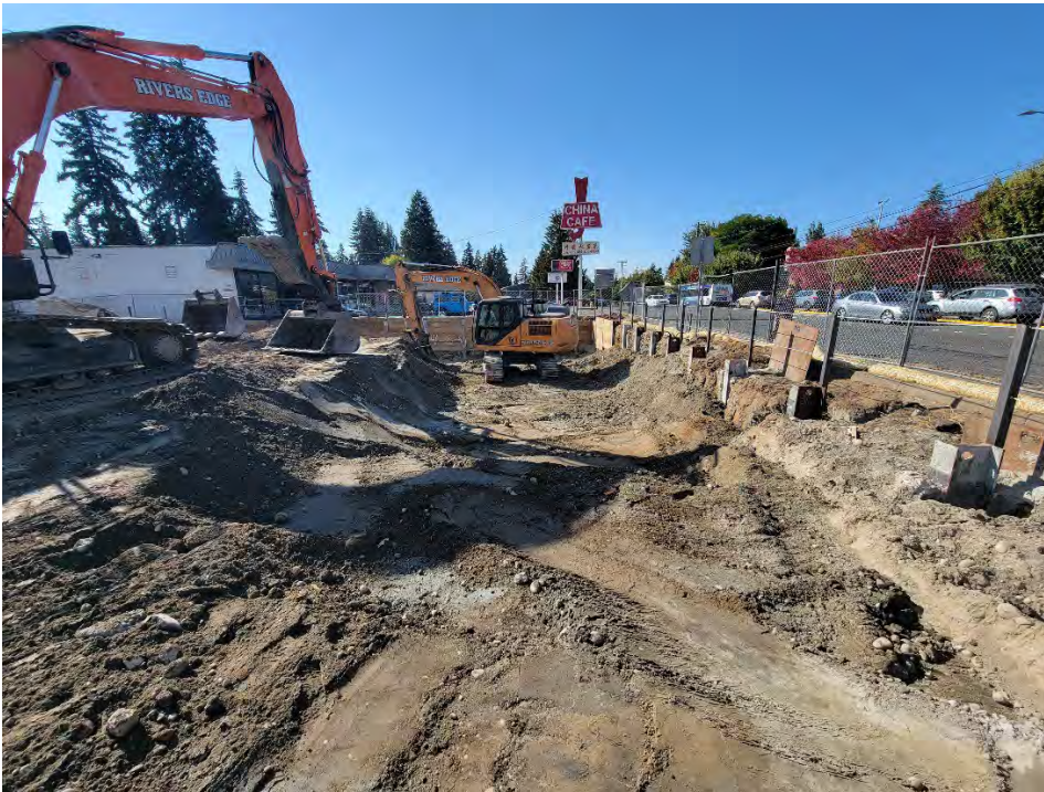
Photo 2: North Sidewalk facing West
