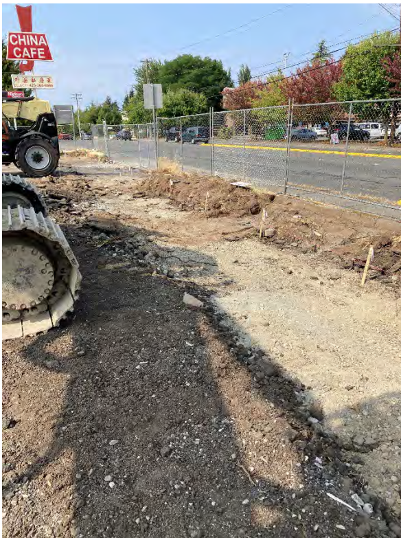
Photo 2: Northern shoring wall with piling staked out.
