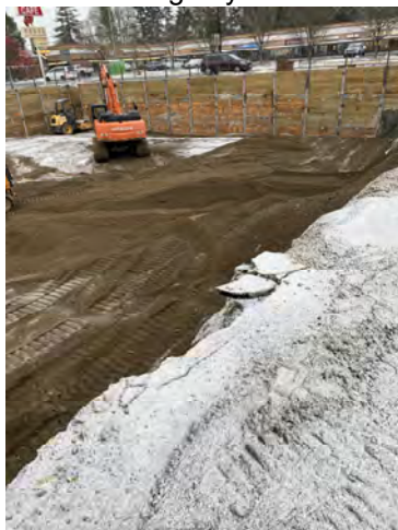
Placing Import Material @ Access Ramp / East Area
