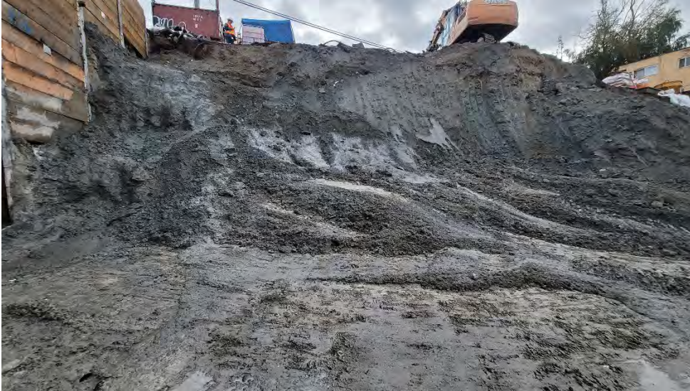
Figure 1. Eastern extent of the excavation near the beginning of the day.
