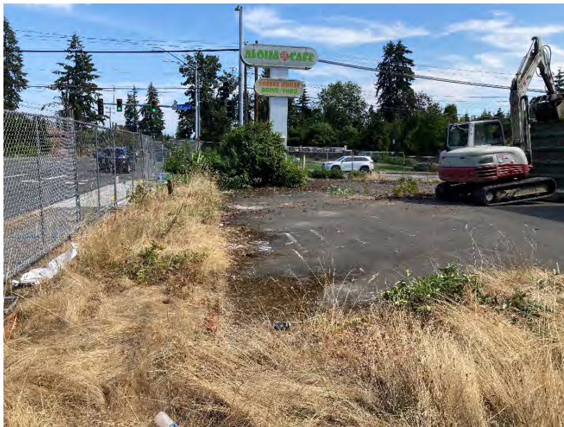
Photo 2: Perimeter fence installed, viewing east.
