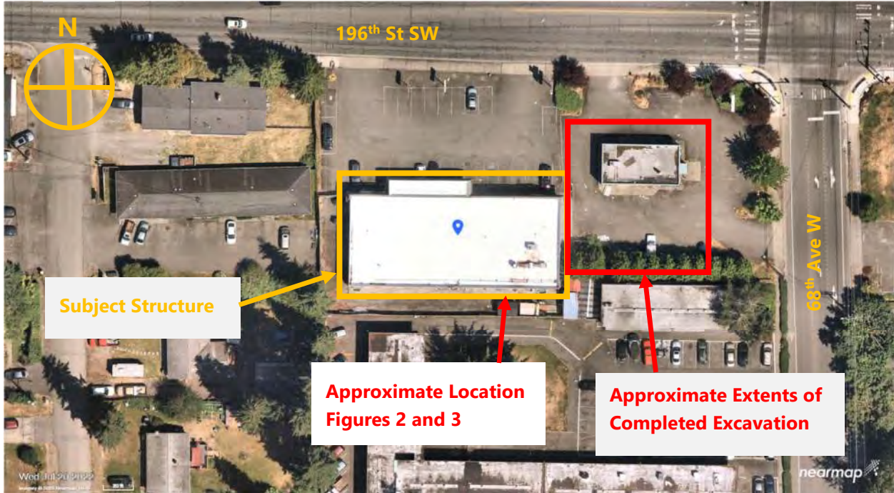
Figure 1. Aerial view of subject property on July 20, 2022. Image © 2022 Nearmap.
