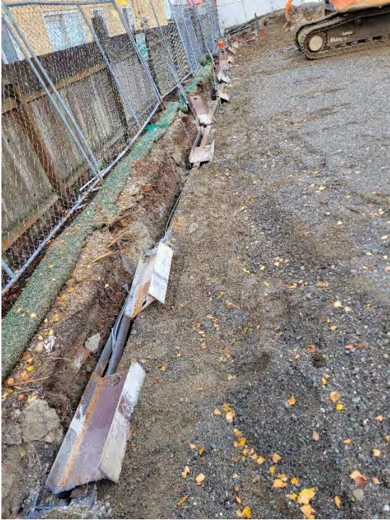
Photo 2. Top approximately 2-feet of soldier piles removed along the south wall.
