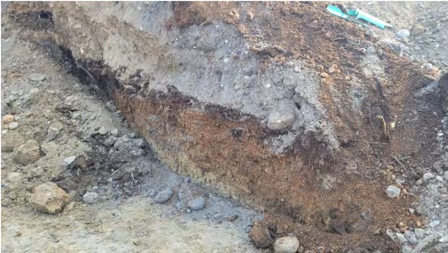
Photo 2. Contact between fill and native material near the southeast corner of the site.
