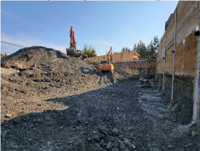
Photo 2: Western section of site at end of day (facing south)
