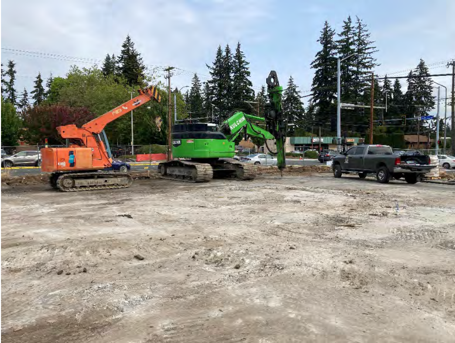
Photo 1: Kulchin's drill rig has been delivered to the site.
