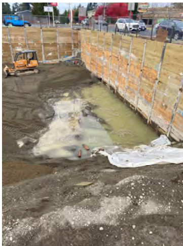
Ground Water @ North Wall
