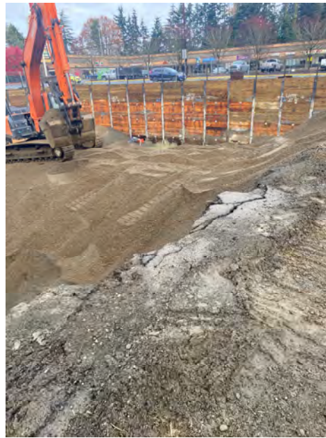
Removing Import Material @ Access Ramp
