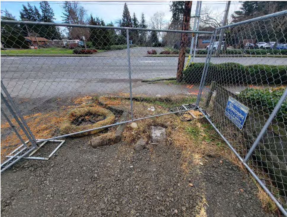
Photo 4. Site TESC measures in-place as of 1/6/2023.
