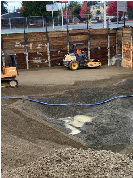
Compacting @ NW Area
