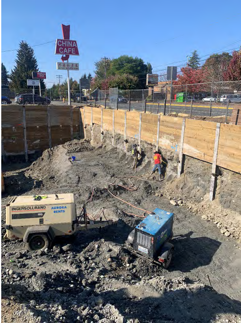
Photo 2. Preparing the north wall for lagging.
