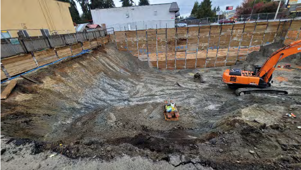
Figure 2. Looking west showing the mostly completed southern edge of the excavation.
