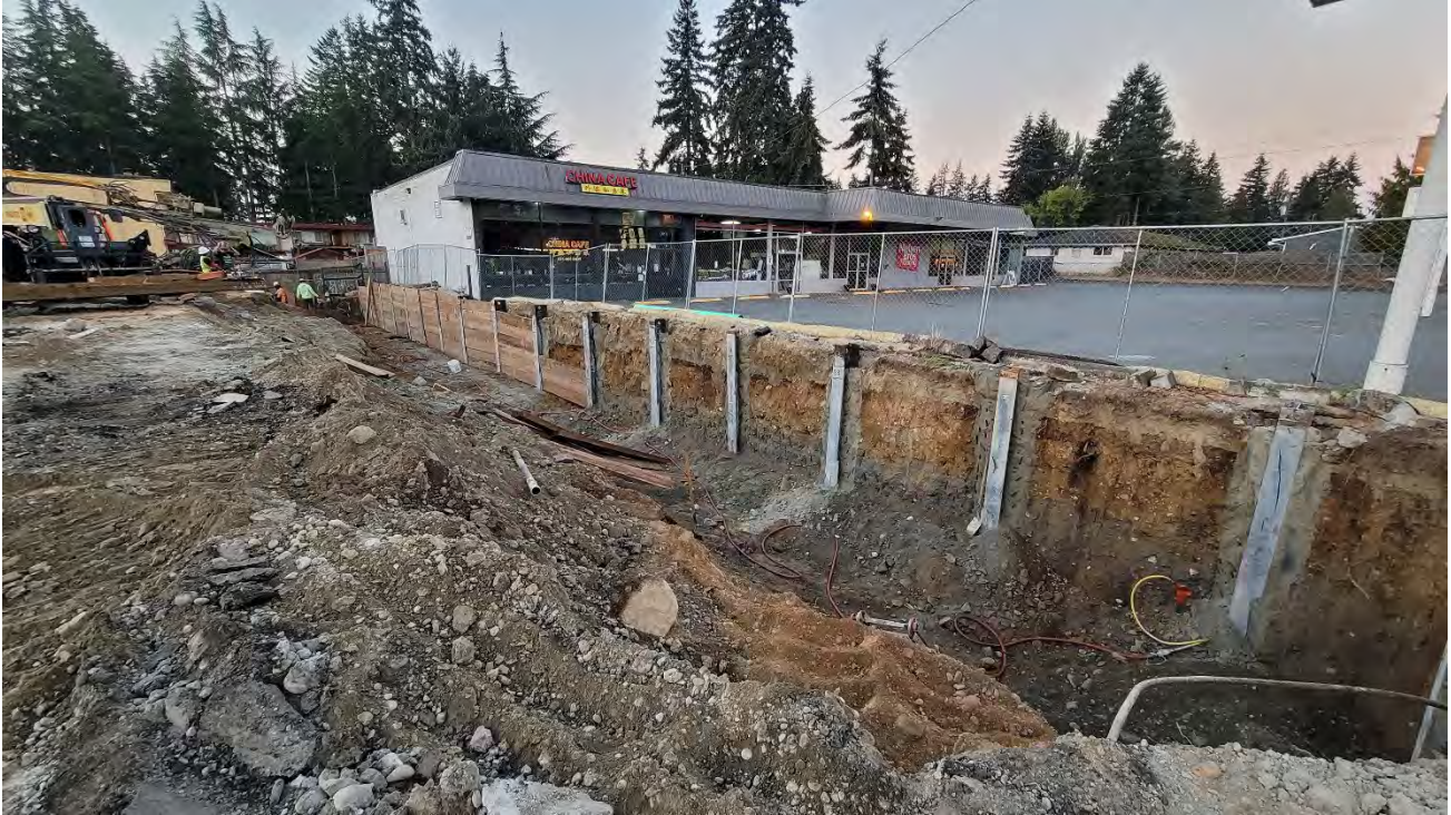
Photo 1: Extent of excavation at the end of 9/26/22. Photo looking west.
