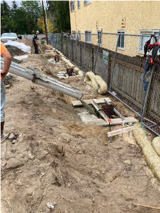
Photo 4: Soldier pile installation progress along the south shoring wall.
