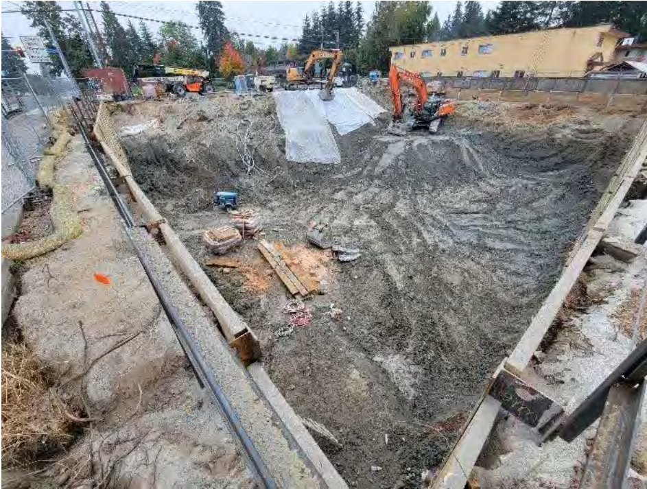
Photo 1: End of day excavation extends facing southeast
