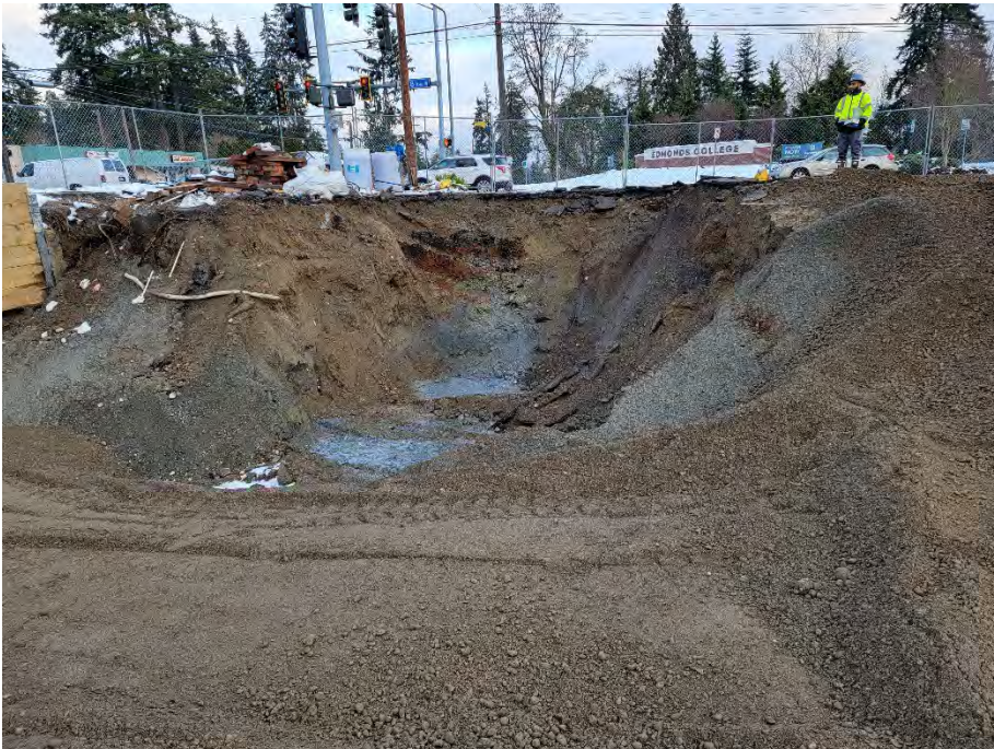
Photo 1. Eastern slope overexcavation in progress, looking south. Contaminated soil is gray.
