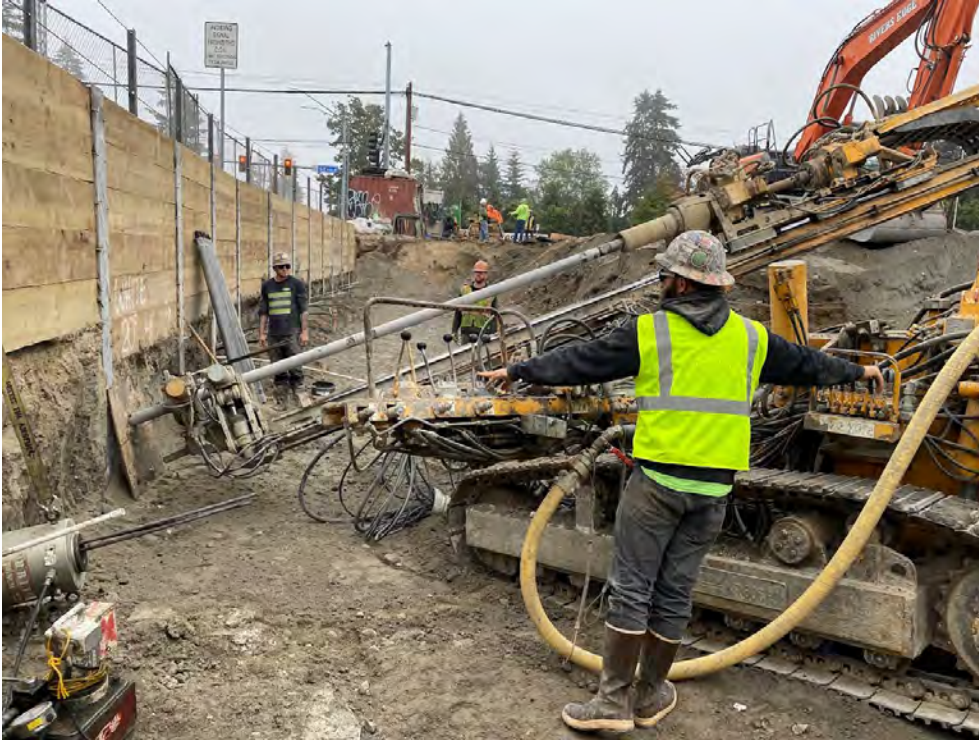
Photo 3: Drill rig positioned to drill the tieback in north wall
