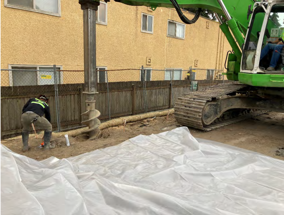
Photo 1: Drilling of the first soldier pile wall by Kulchin.
