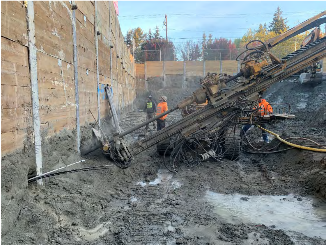
Photo 1. Installation of W6/R2 1' lower than original location.
