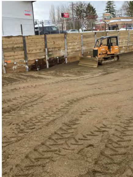
Tested West Area of Site
