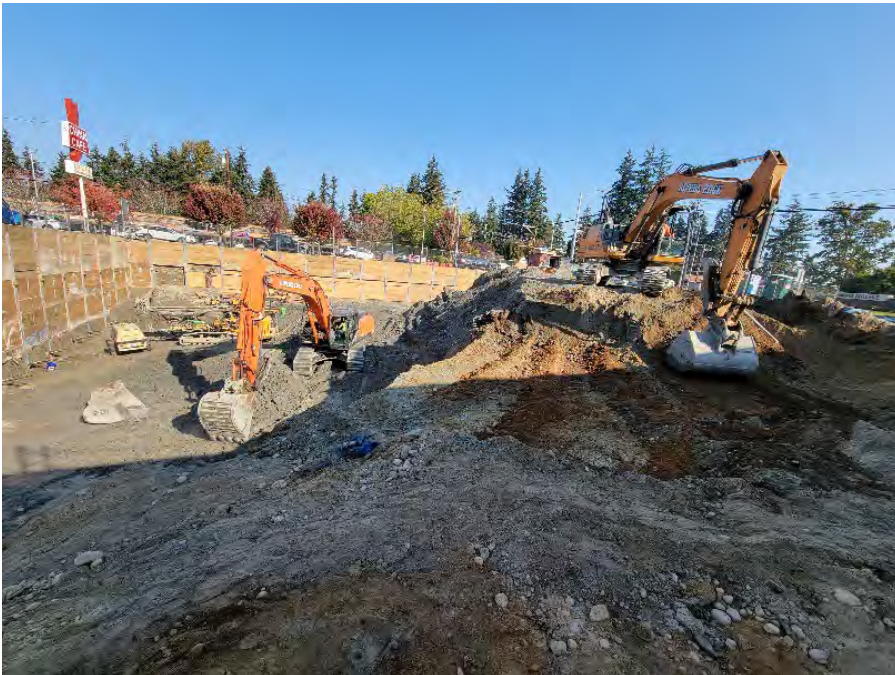
Photo 2: Excavation progression, excavating in contaminated (left) and clean (right).
