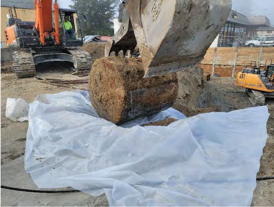
Photo 1: UST 3 after being pulled.
