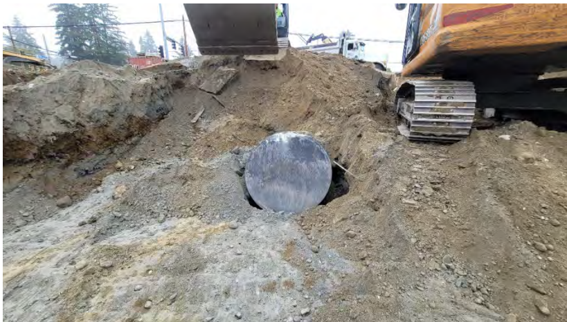
Photo 1. UST 2, just after discovery.
