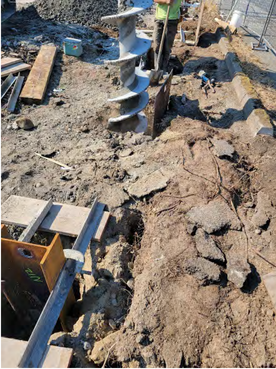
Photo 1: Drilling of soldier pile.
