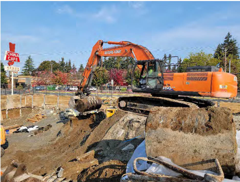
Photo 2: UST 1 being pulled (background) UST 3 in foreground.
