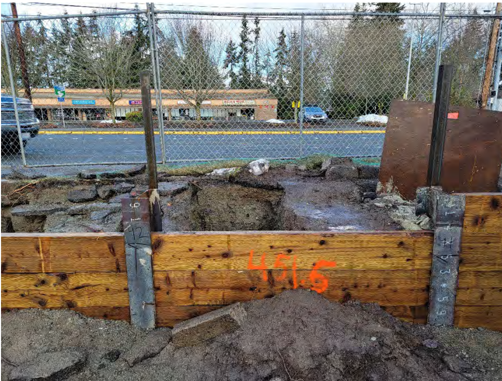
Photo 3. Photo of cell N08-N08.5 after vector excavation completed.
