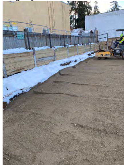
Compacting Import Material / South Area
