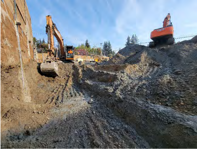
Photo 1: Actively excavating western sidewall (facing north)
