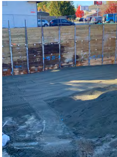
Rolled, Compacted & Tested Area
