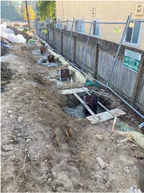
Photo 1: South Soldier Pile Wall, all piles installed viewing east.
