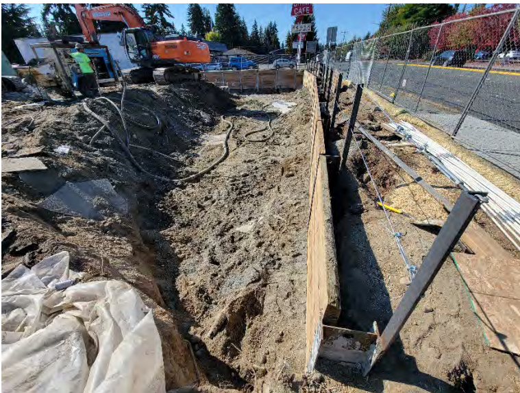
Figure 2 Northern sidewall benched and lagged
