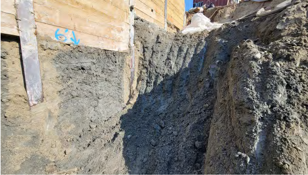
Figure 2. Photo of the northeast corner of the site, near pile N12 and N13, showing the amount of groundwater seepage in this location.
