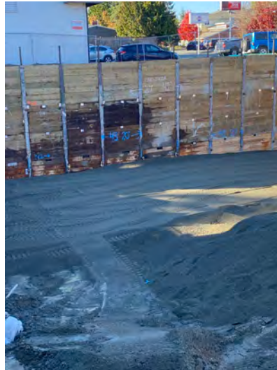
Placed & Compacted Gravel Barrow
