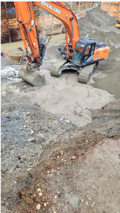
Photo 2. Attempted mud consolidation; the mud being scraped from the base of the site is very saturated by ground and rainwater infiltration.
