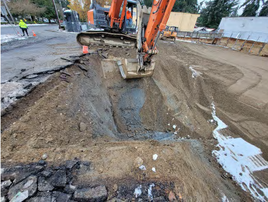
Photo 1. Eastern slope overexcavation in progress, looking south. Contaminated soil is gray.
