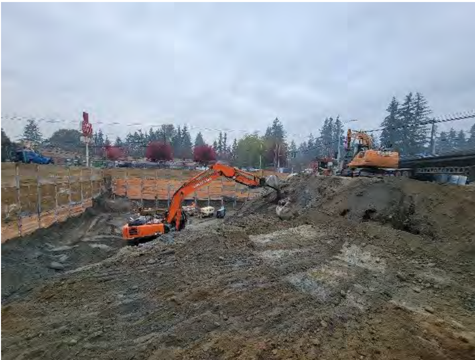
Photo 2: Excavator actively moving contaminated soil to the loading zone
