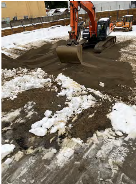
Placing Material Import Material @ Access Ramp / South Area
