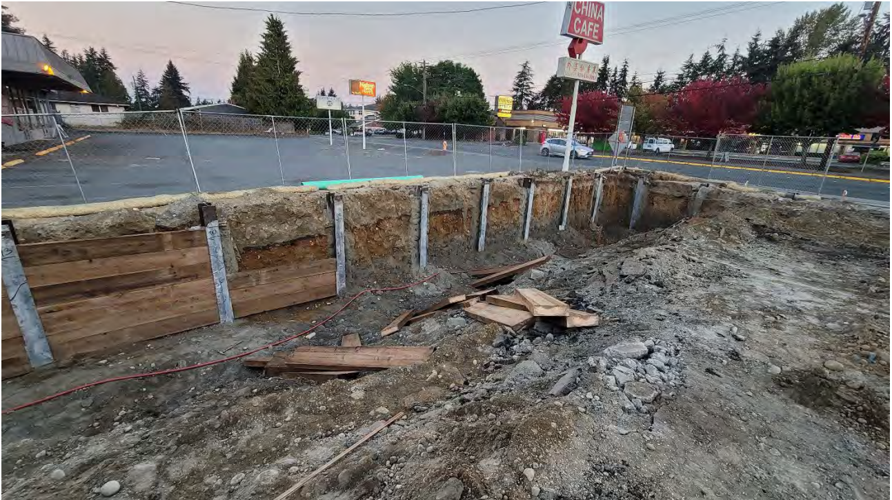
Photo 2: Extent of excavation at the end of 9/26/22. Photo looking northwest.
