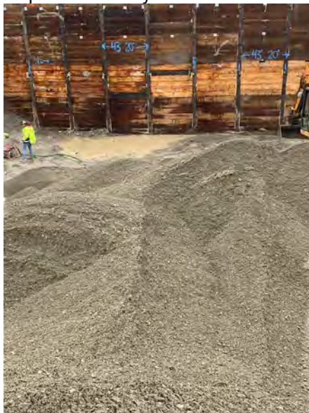
Water Accumulation Area / West Wall
