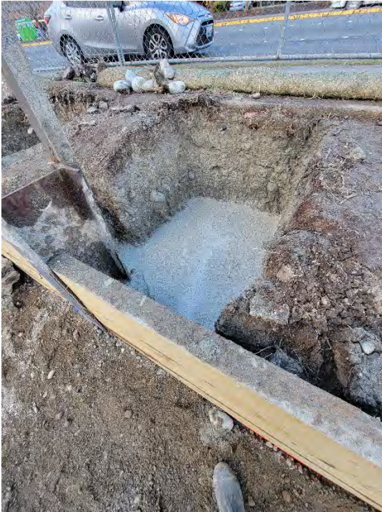
Photo 1. Overexcavation N10 to N10.5 backfilled with CDF.
