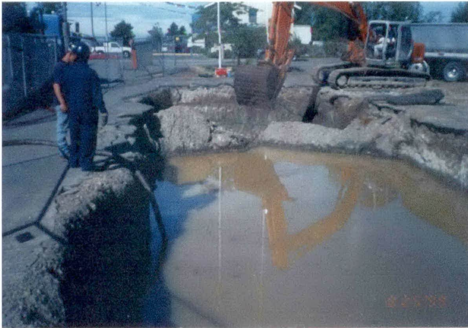
Figure 3. Subject property view to the west. Water in tank pit is approximately 5.0 feet below ground surface in this photograph.
