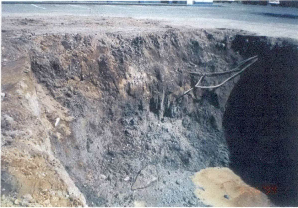
Figure 5. Photograph of west wall of tank pit after water was pumped out. Water at the bottom of the excavation originated from a 1.5 foot thick layer of pea gravel that was underlain by native blue clay.
