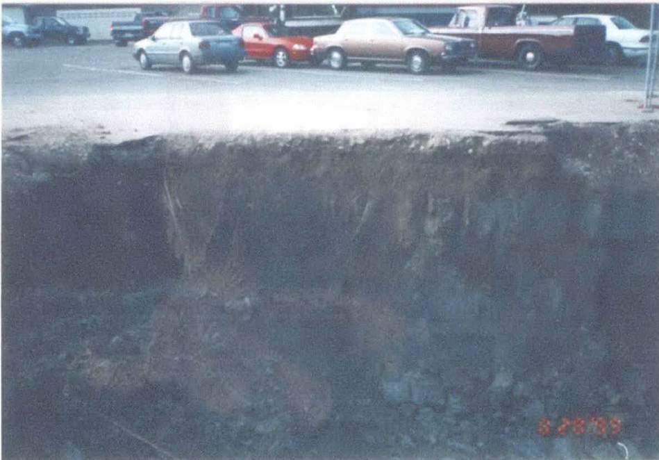
Figure 6. Photograph of the south wall of the excavation. Depth to pit bottom was approximately 14.0 feet.
