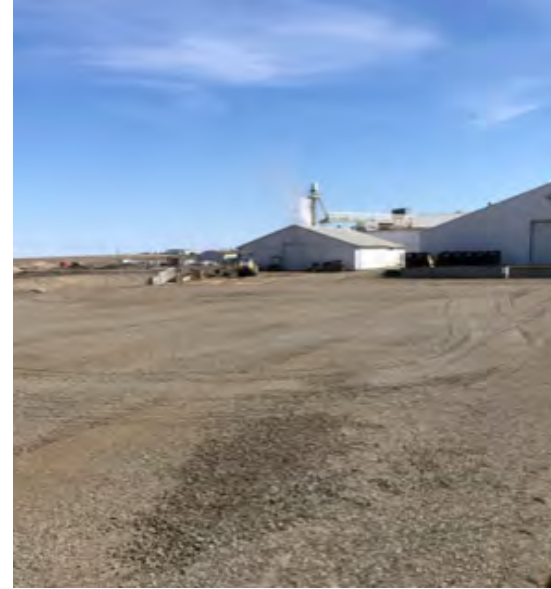
Photo 26. View of SGS site after final grading operations were completed. Photo taken from southwestern boundary facing northeast. Photo taken on March 27, 2023.
