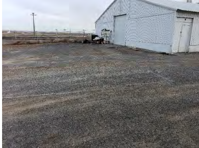
Photo 1. View of SGS site storage shed and east pit prior to excavation. Photo facing northeast, taken on March 8, 2021.
