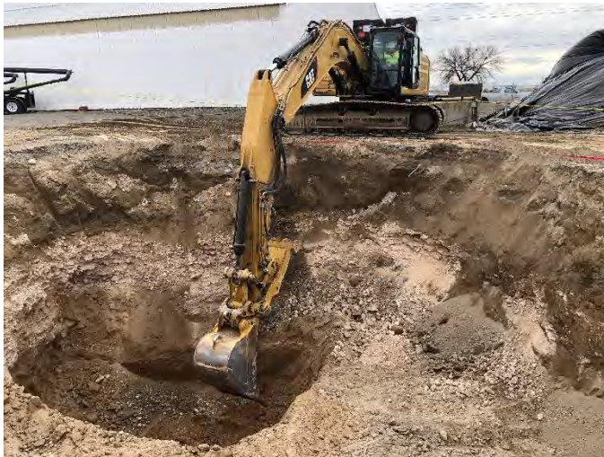
Photo 7. View of east pit excavation area on March 15, 2021. Photo facing south.
