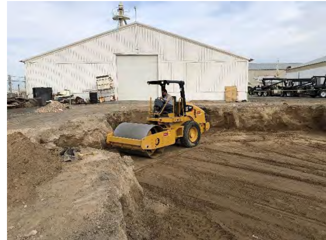
Photo 10. View compaction activities in east pit. Photo taken on April 2, 2021.
