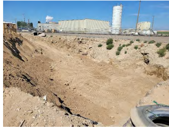
Photo 22. View of west pit backfilling. Photo taken on August 10, 2022, facing southwest.
