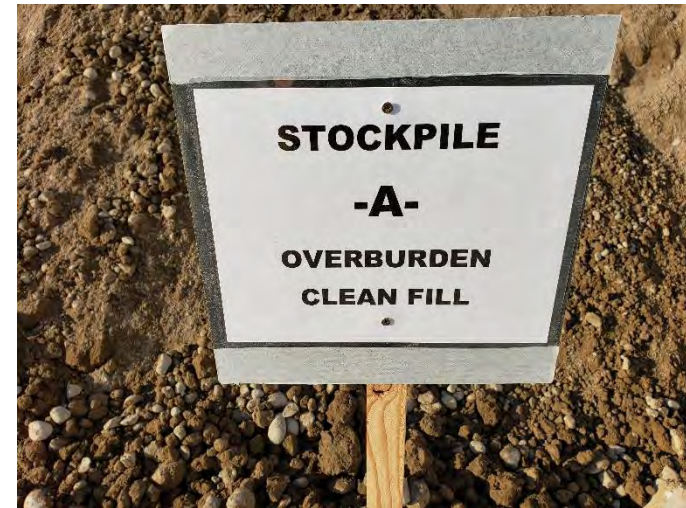
Photo 4. Detail of signage used to label clean overburden soil stockpiles during excavation activities.
