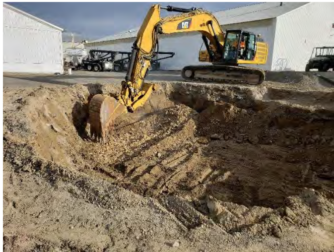
Photo 3. View of east pit facing southeast, taken on March 9, 2021.
