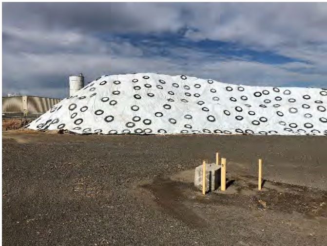
Photo 15. View of final soil contaminated pile with winter protection practices implemented. Photo taken on October 4, 2021.
