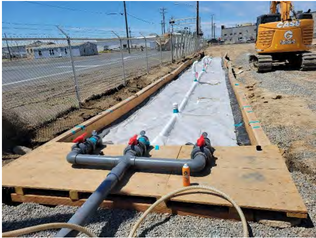
Photo 21. View of negative pressure observed during SVE treatment. Photo taken on June 15, 2022.
