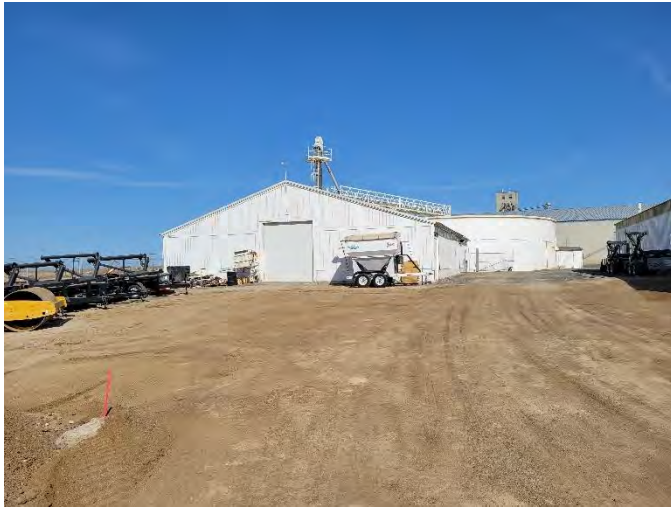
Photo 13. View of backfilled east pit. Photo taken on April 6, 2021, facing east.
