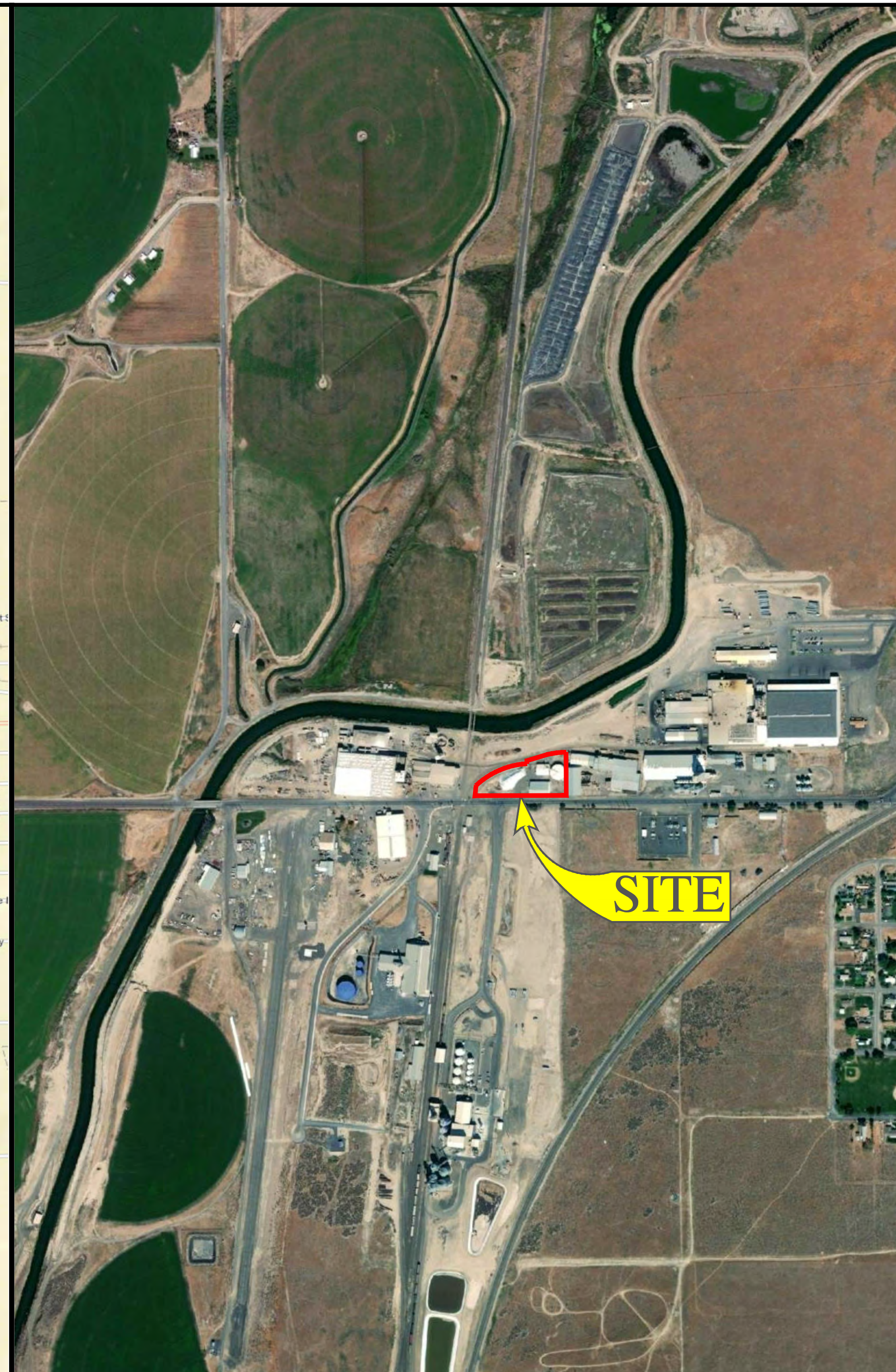
VICINITY AERIAL PHOTOGRAPH
