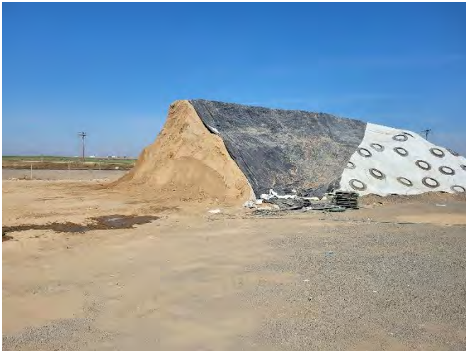
Photo 23. View of contaminated pile during SVE treatment operation. Photo taken on October 12, 2021.
