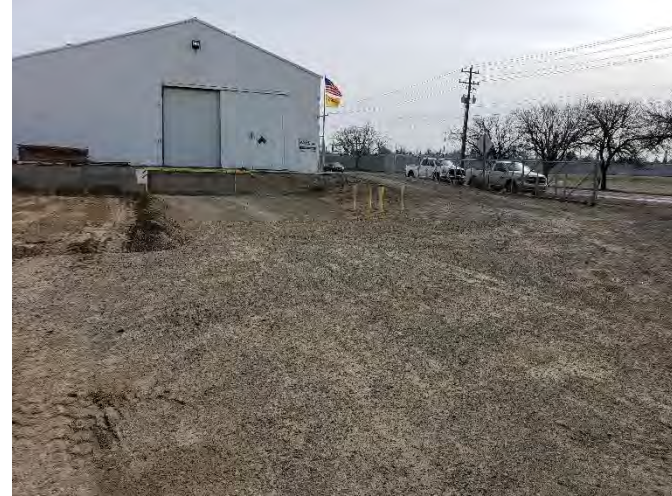
Photo 2. View of SGS site warehouse/office building. Photo taken on March 8, 2021.
