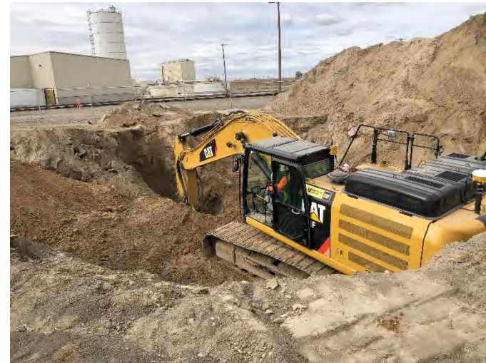
Photo 8. View of west pit excavation area on March 15, 2021. Photo facing northwest.
