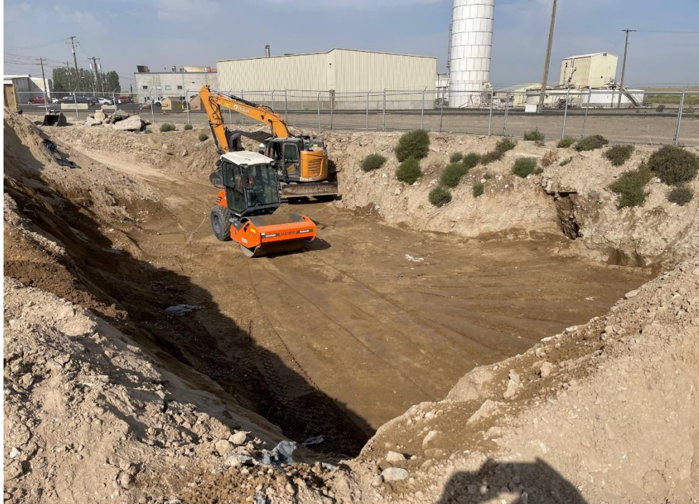
Rolling 1st lift of the day
