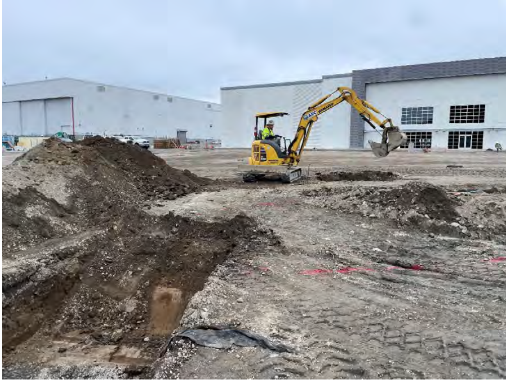
Figure 94: Overview at End of Day 3/9/2023
