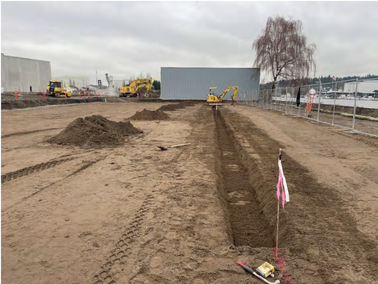
Figure 3: Overview of northern trench at end of excavation, facing South
