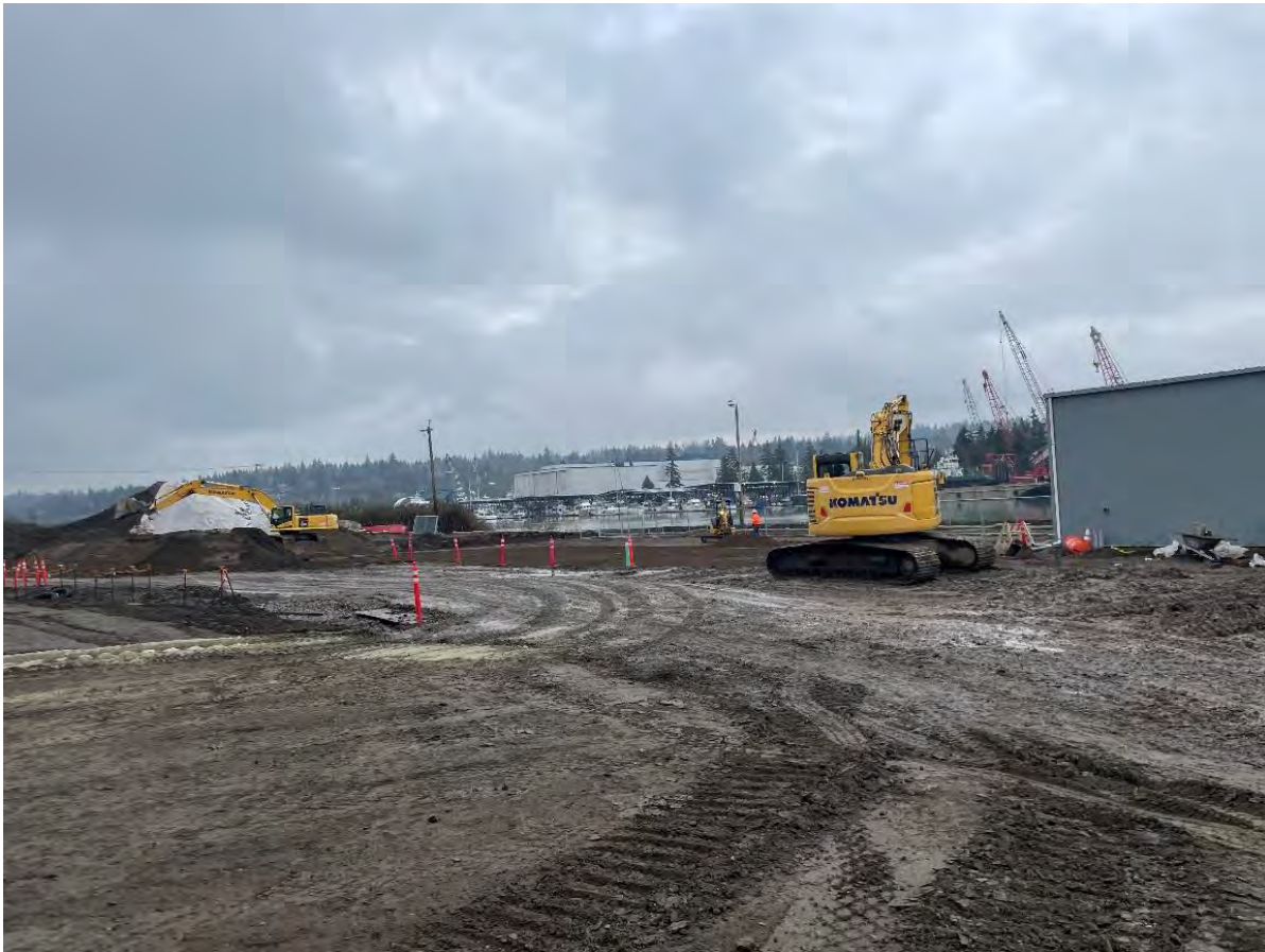
Figure 4: Overview of southern trench before excavation, facing Southwest
