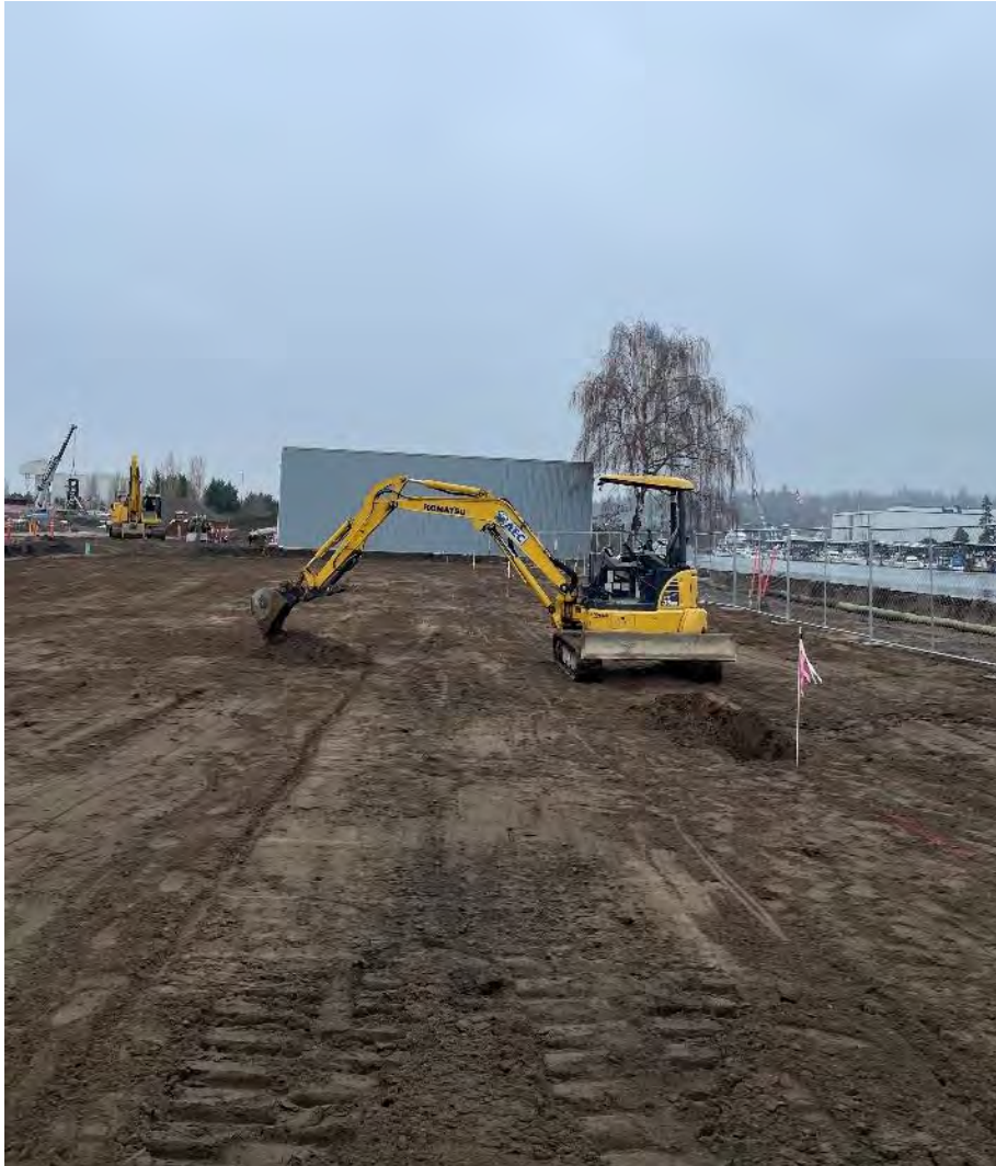
Figure 2: Overview of northern trench at start of excavation, facing South
