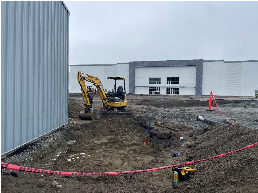
Figure 86: Overview at Start of Excavation
