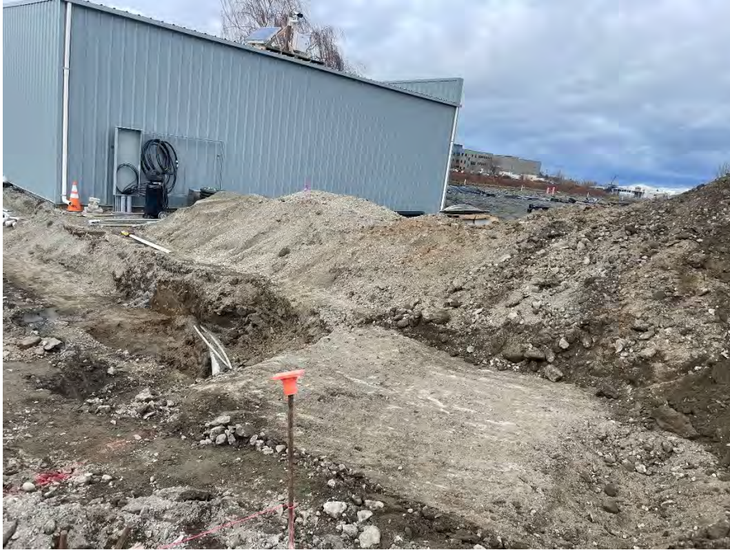
Figure 98: Concrete Layer and Unaffiliated Pipes, Briefly Paused Excavation
