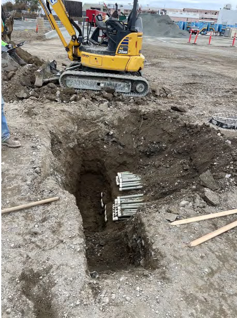
Figure 93: Overview of Pipes Exposed on E Side
