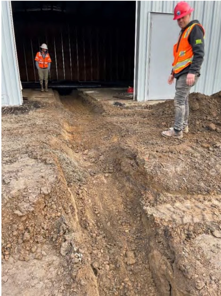
Figure 10: Overview of AS/SVE Building trench connecting to southern trench, facing North
