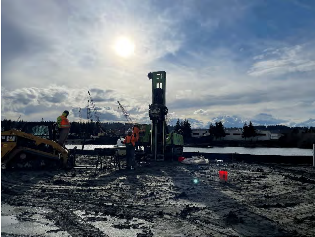
Figure 51: ASW-39 Overview at Start of Drilling
