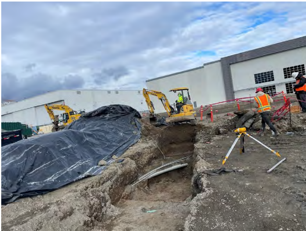
Figure 103: End of Day Overview Over W Trench
