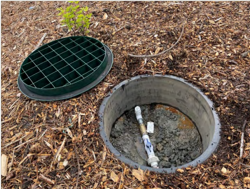
Exhibit A-2: Photo of an AS Well Monument in the Landscaped Berm
