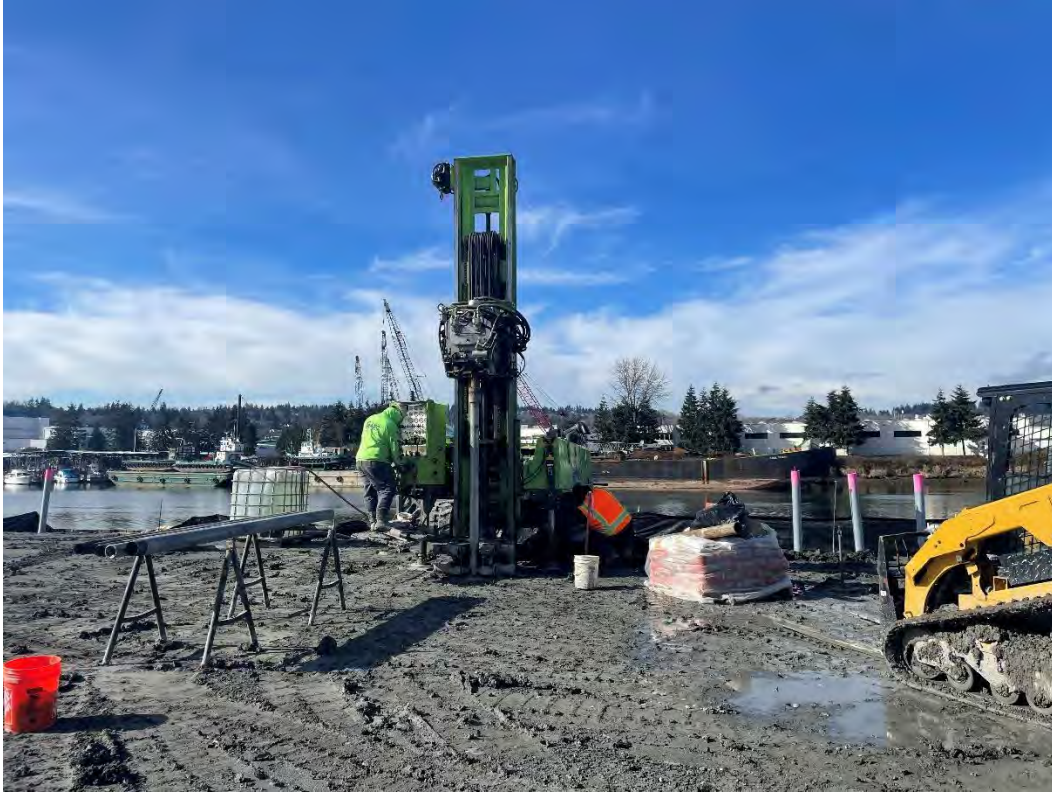
Figure 61: ASW-37 Overview at Start of Drilling
