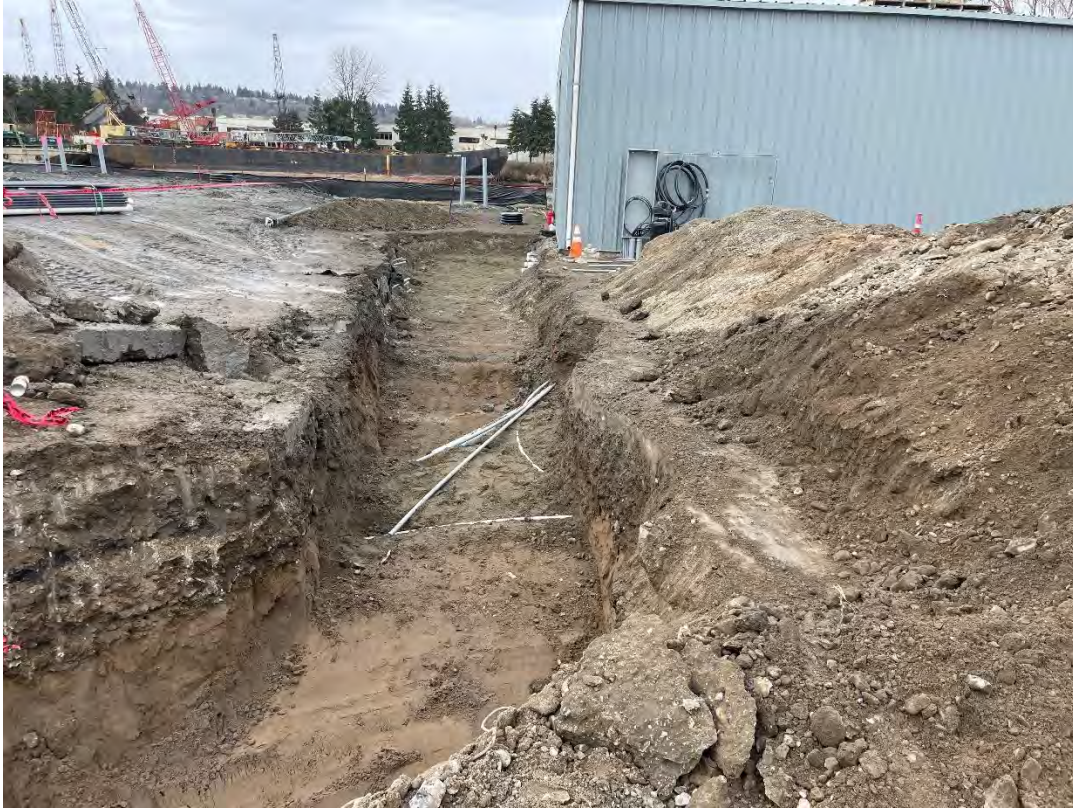
Figure 108: E and W Trenches Merge
