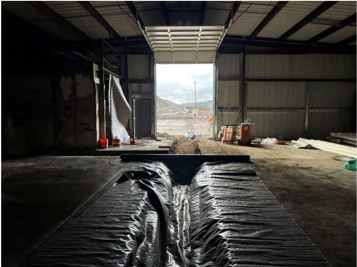
Figure 11: Overview of AS/SVE Building trench at completion of excavation, facing South
