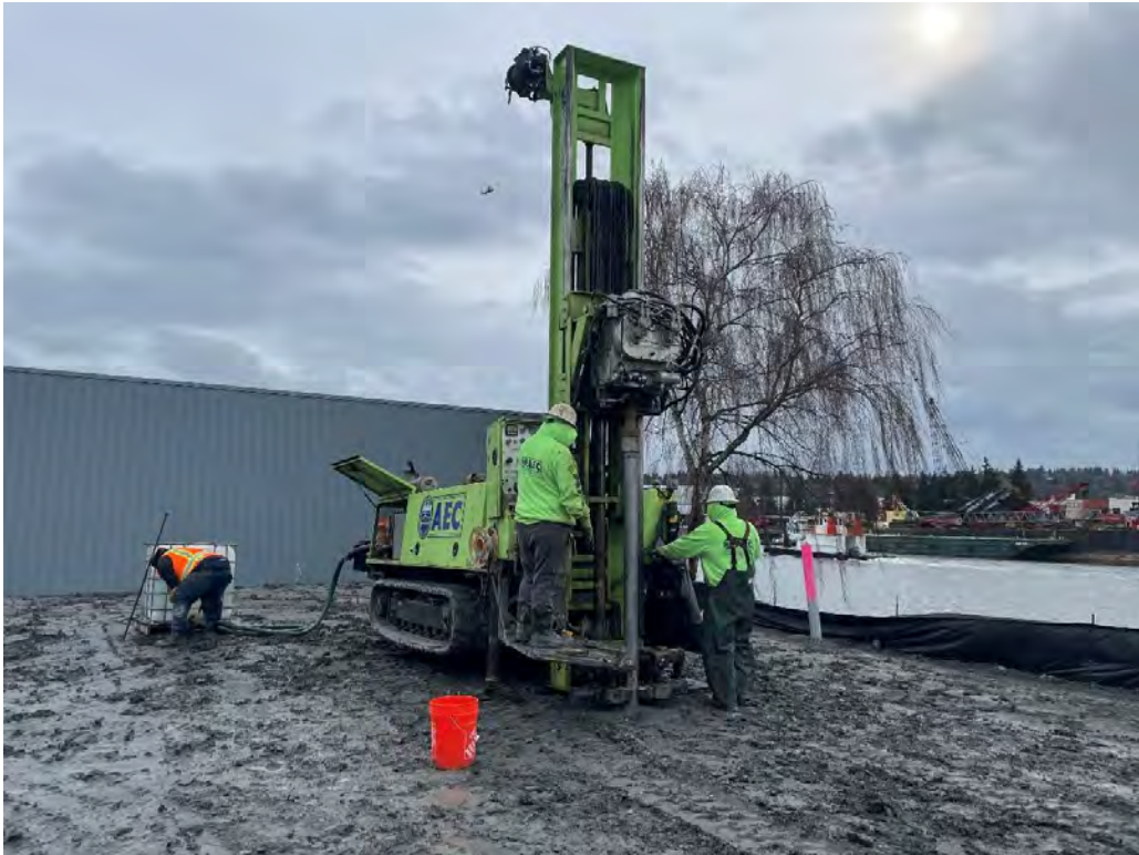
Figure 24: ASW-50 Overview at Start of Drilling
