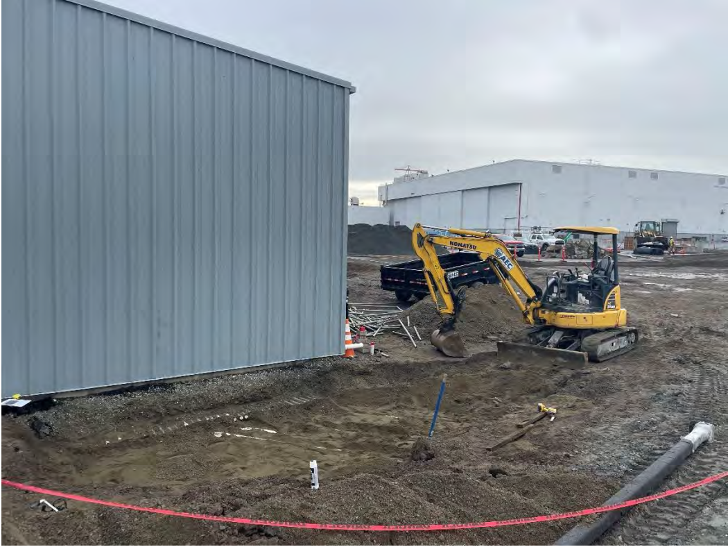
Figure 85: Overview at Start of Excavation
