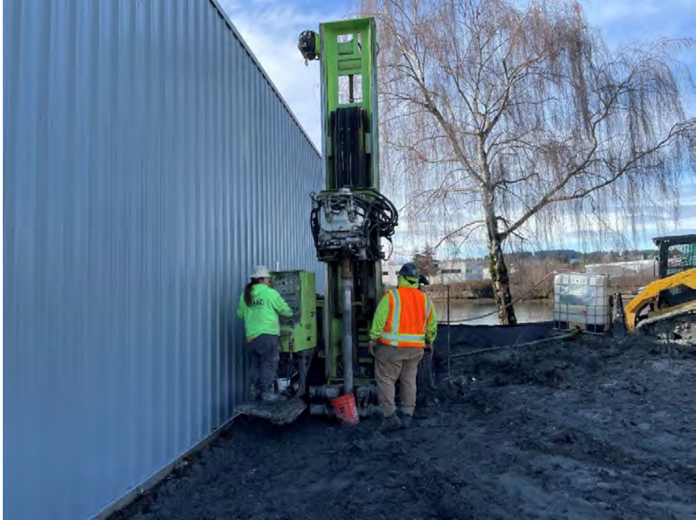
Figure 39: ASW-46 Overview at Start of Drilling
