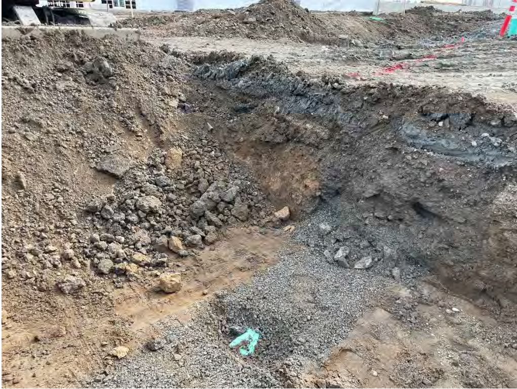
Figure 91: Overview of Blue Unaffiliated Pipe/Abrupt Soil Disturbance Layers
