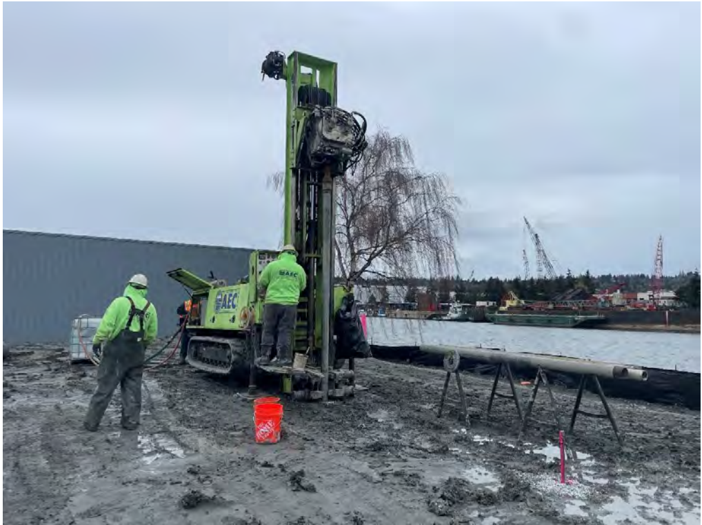
Figure 20: ASW-51 Overview at Start of Drilling
