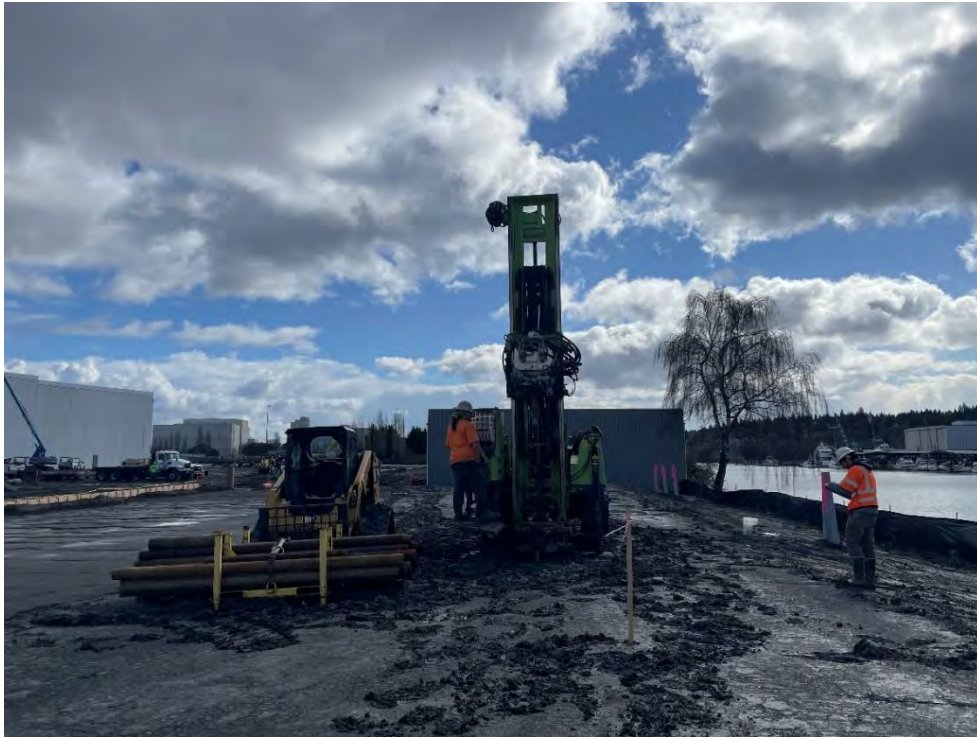
Figure 1: ASW-55 Overview at Start of Drilling
