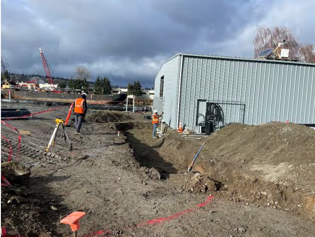
Figure 96: Use of Laser to Measure Differing Pipe Depths
