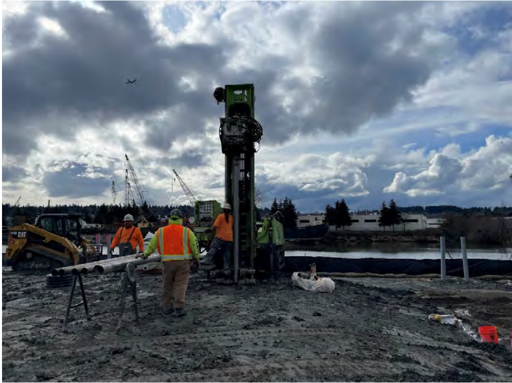
Figure 48: ASW-40 Overview at Start of Drilling
