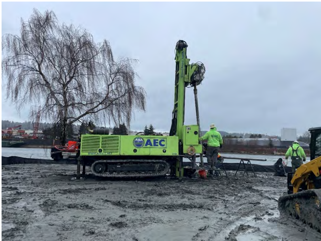
Figure 28: ASW-49 Overview at Start of Drilling
