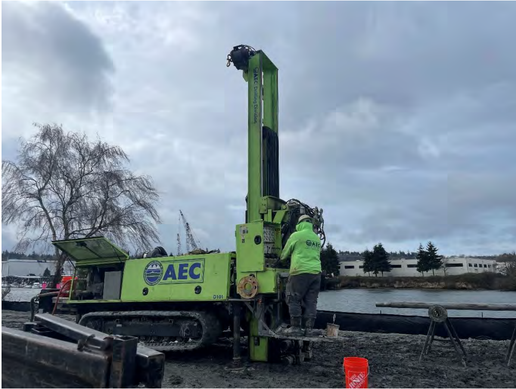
Figure 17: ASW-52 Soil Extraction 0-10 ft bgs
