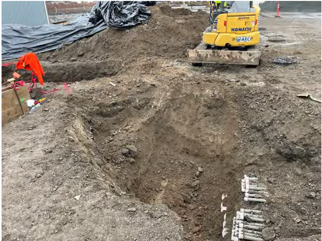
Figure 107: Progress Photo of E Trench Excavation
