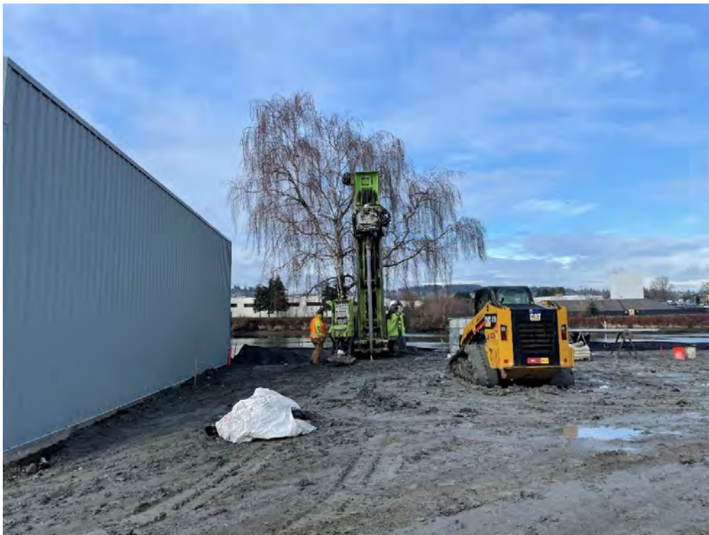
Figure 36: ASW-47 Overview at Start of Drilling
