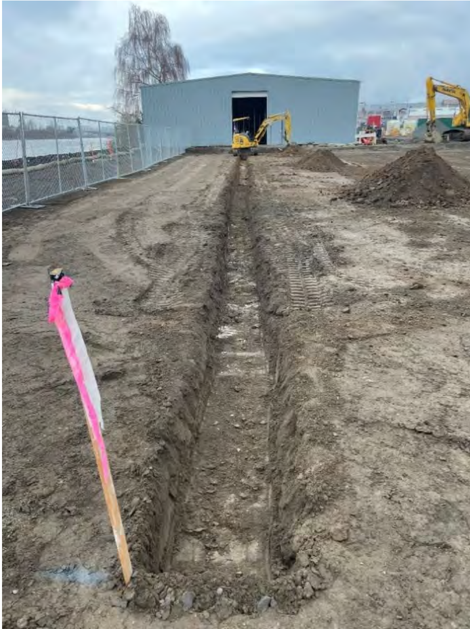
Figure 6: Overview of southern trench at end of excavation, facing North
