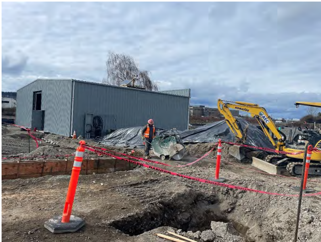
Figure 99: Saw Used to Cut Concrete Layer
