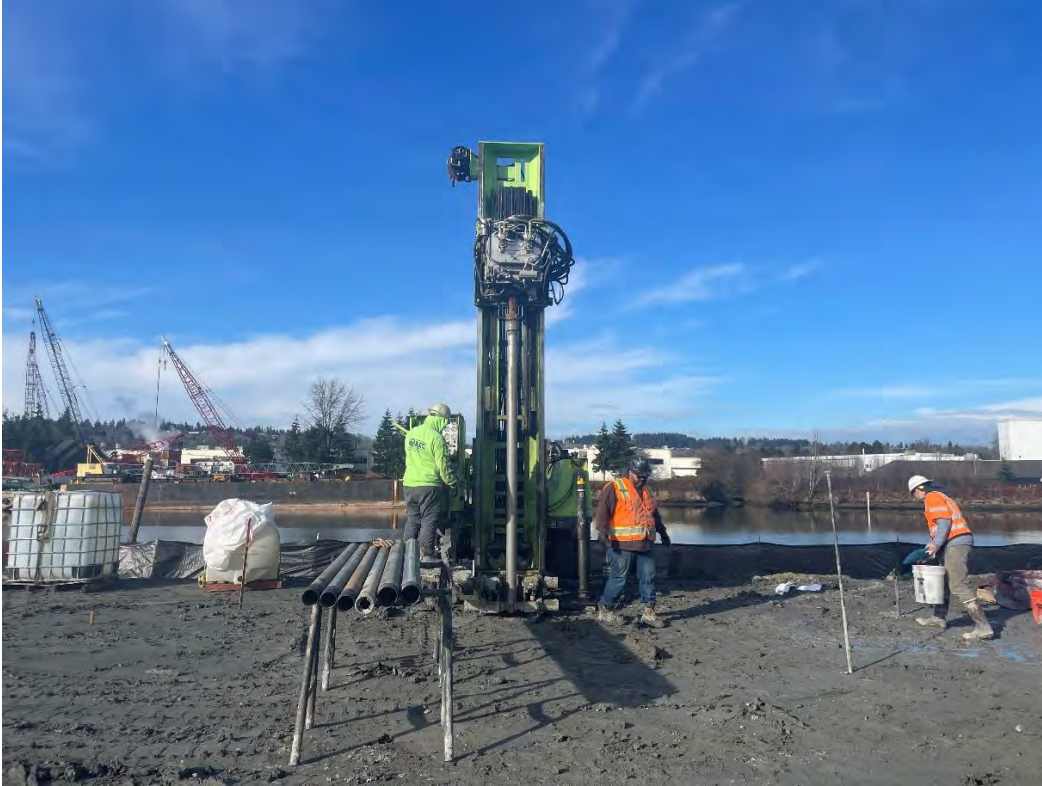
Figure 55: ASW-38 Overview at Start of Drilling
