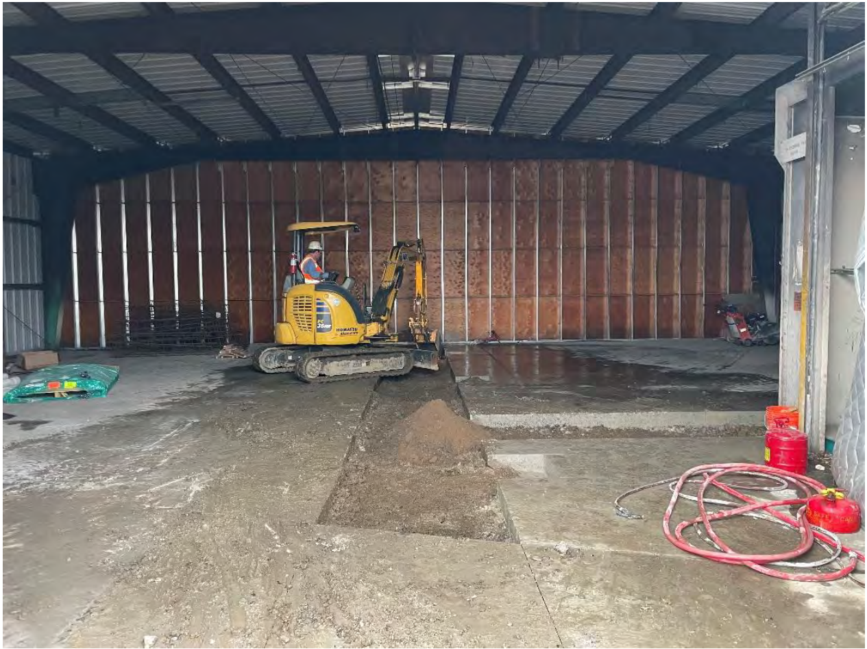
Figure 7: Overview of AS/SVE Building trench at start of excavation, facing North
