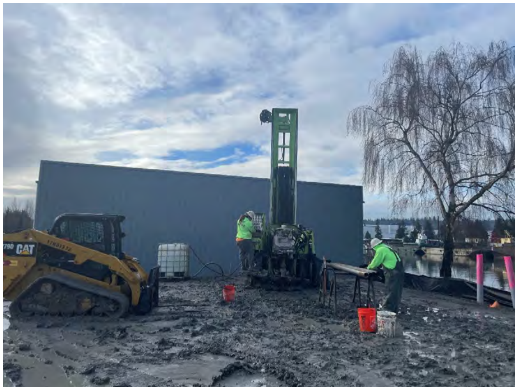
Figure 32: ASW-48 Overview at Start of Drilling
