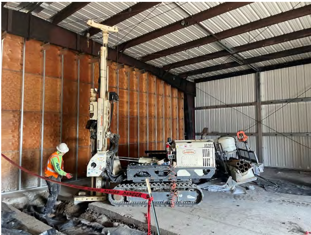
Figure 60: ASW-45 Overview at Start of Drilling
