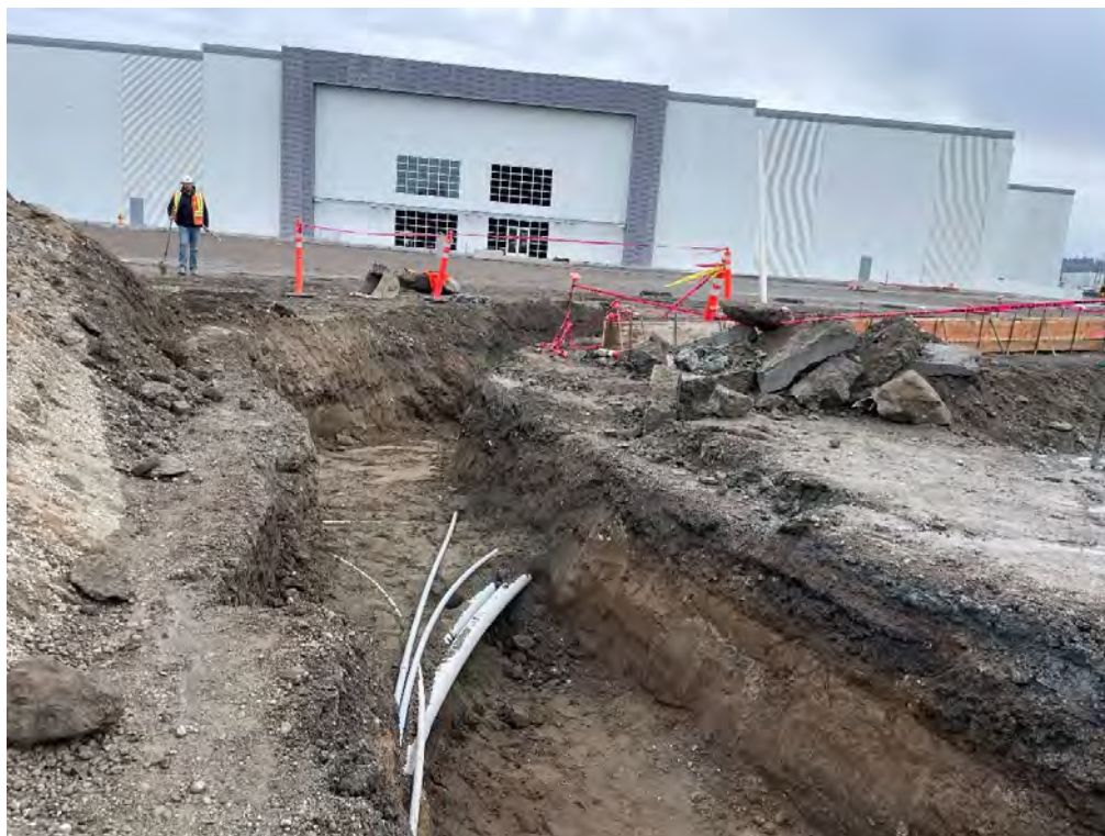
Figure 109: Completion of Trench Excavation Overview
