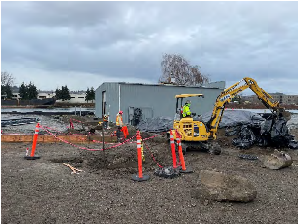
Figure 105: Overview of E and W Trench at Start of Day 3/11/2023
