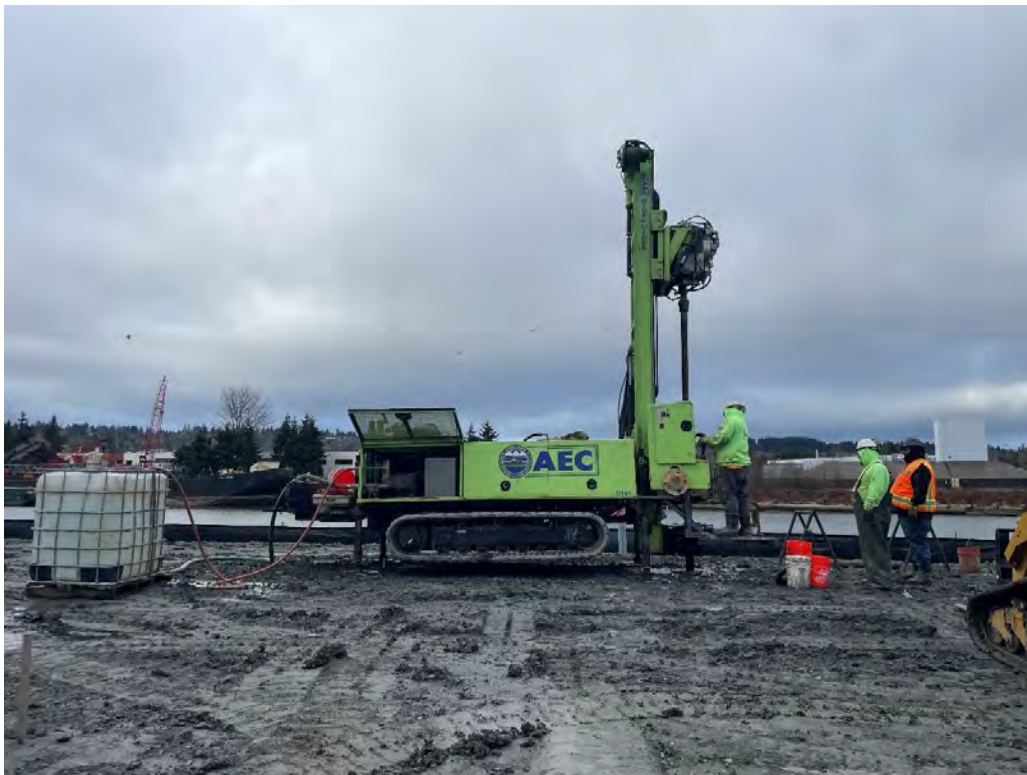
Figure 8: ASW-54 Overview at Start of Drilling
