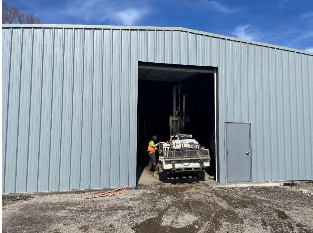
Figure 73: ASW-43 Overview at Start of Drilling
