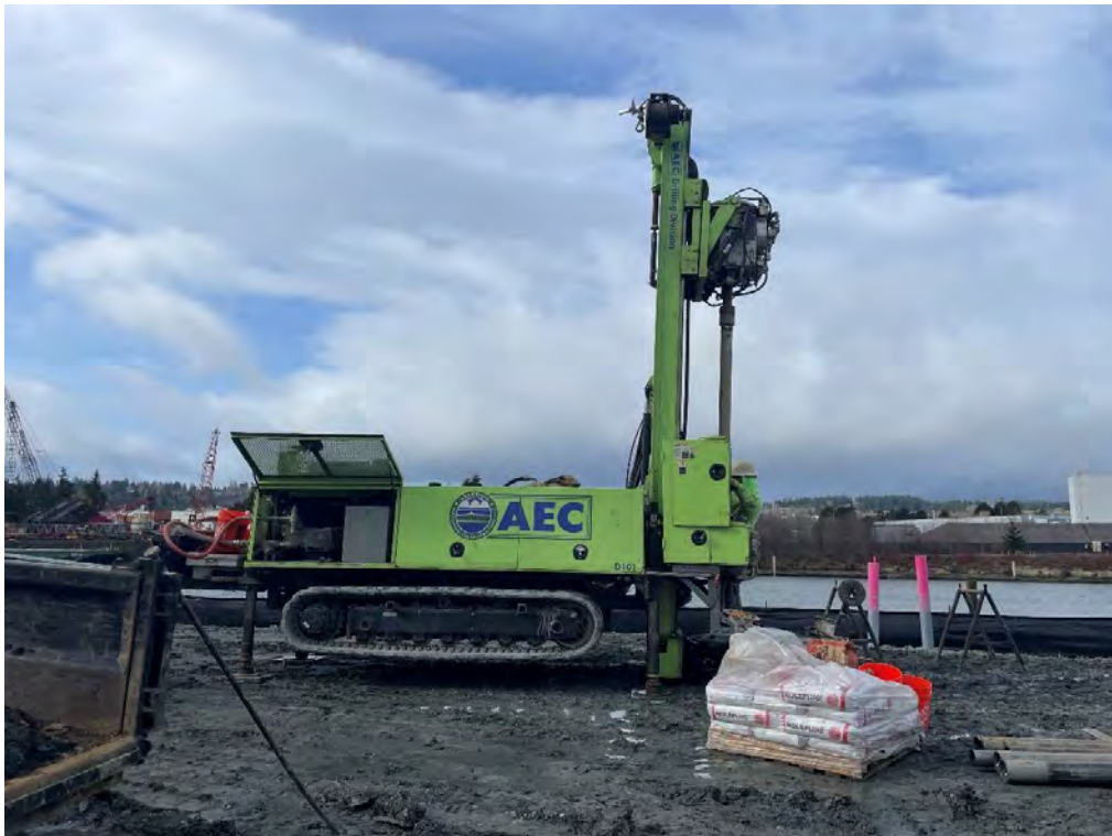
Figure 12: ASW-53 Overview at Start of Drilling
