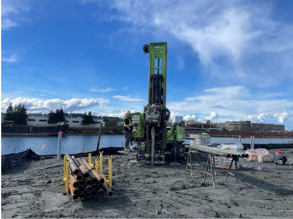
Figure 79: ASW-34 Overview at Start of Drilling
