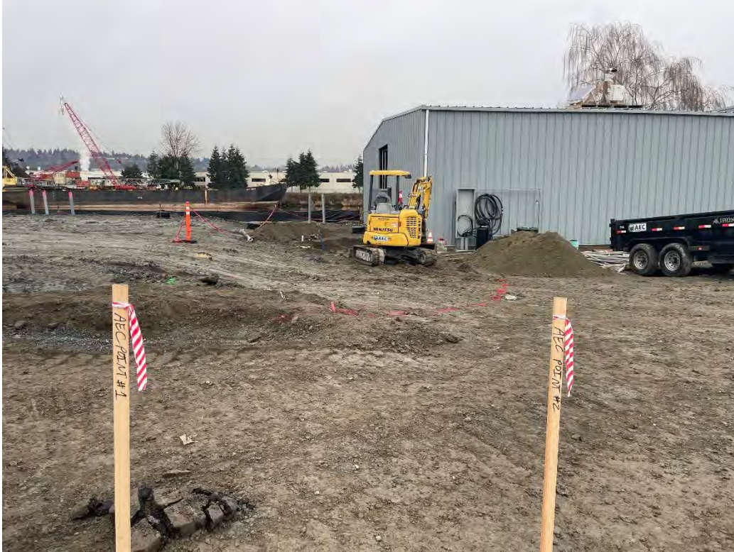
Figure 87: Overview of Trench Layout before Excavation, from E End
