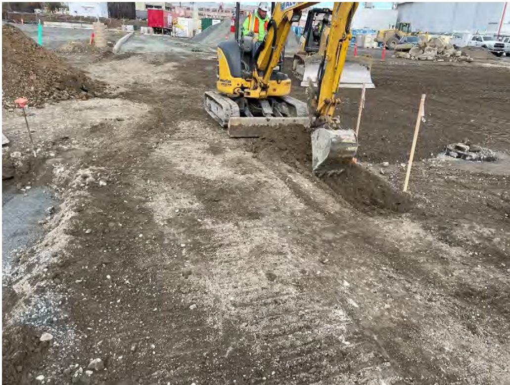
Figure 92: Overview at Start of Excavation on E Side
