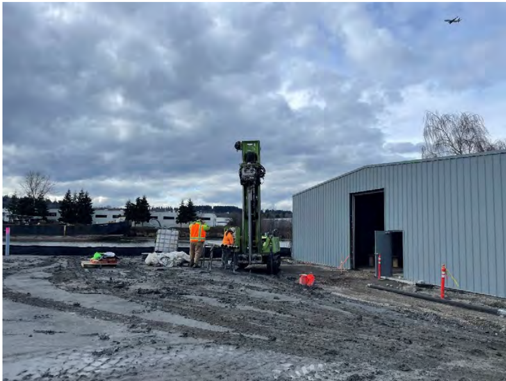
Figure 44: ASW-41 Overview at Start of Drilling
