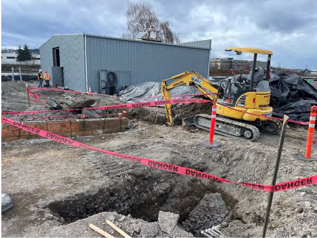
Figure 104: End of Day Overview from E Trench
