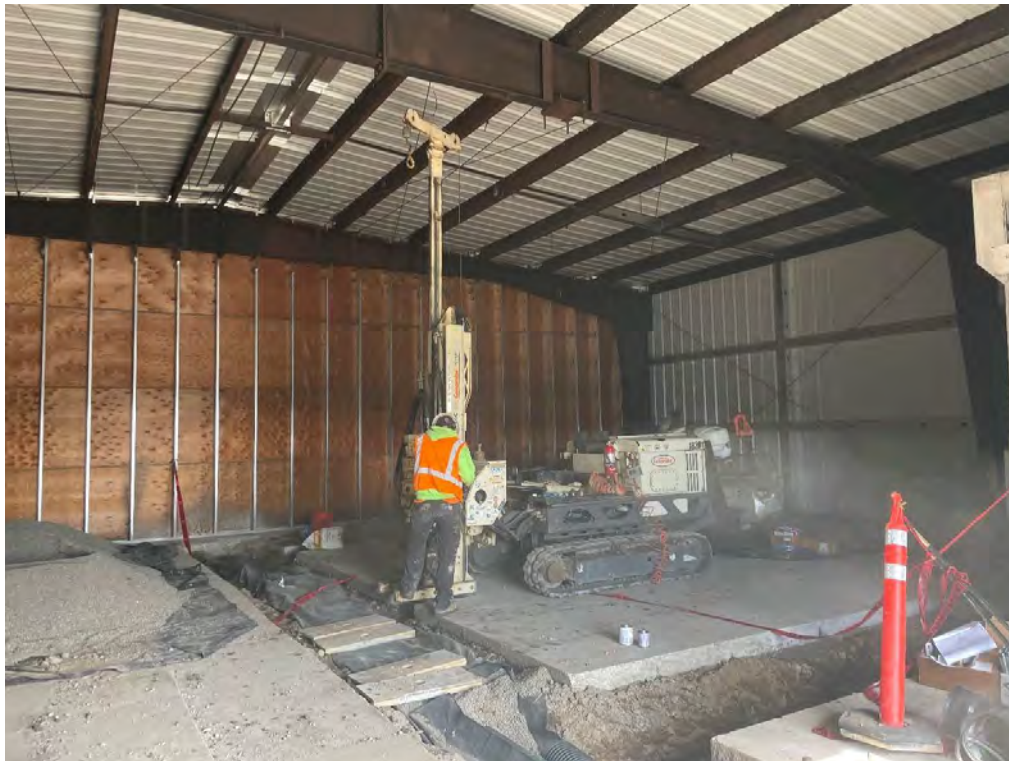
Figure 68: ASW-44 Overview at Start of Drilling
