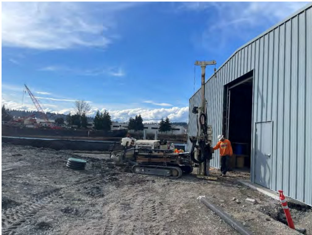
Figure 78: ASW-42 Overview at Start of Drilling
