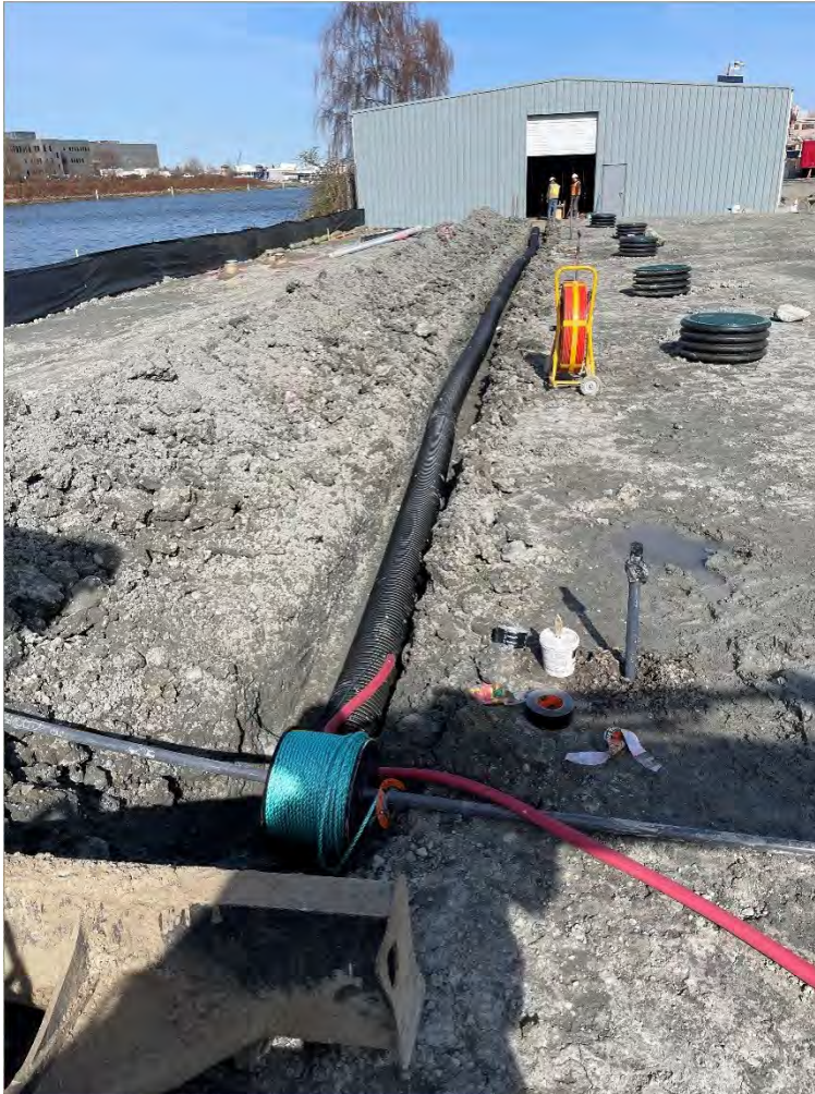
Exhibit A-4: Photo of the AS Conduit to the South of the AS/SVE Building, Looking North
