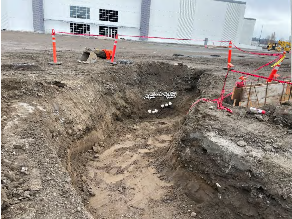
Figure 110: Completion of Trench Excavation Overview
