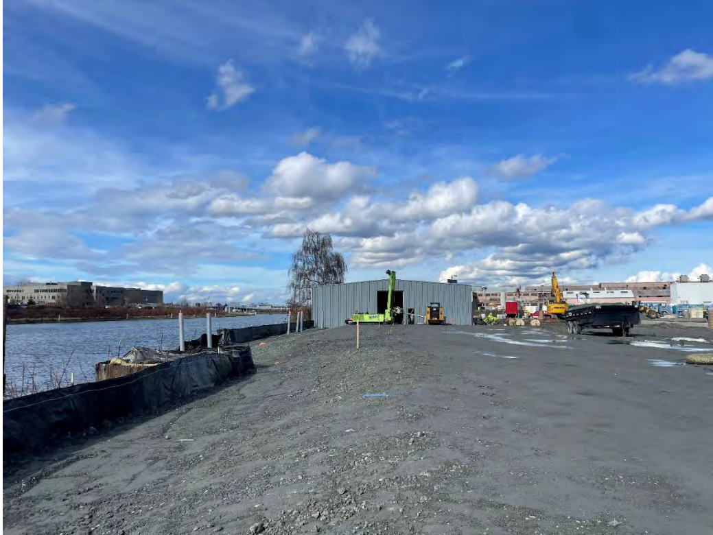
Figure 43: Overview of SW Section Before Drilling/Input of Wells
