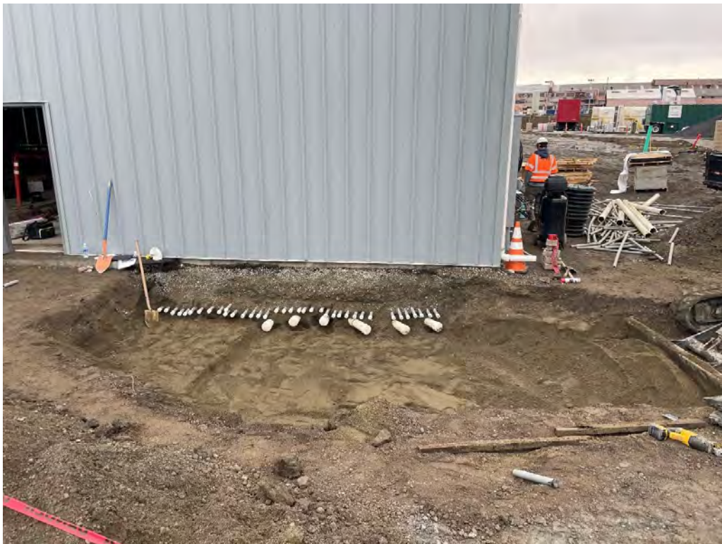
Figure 88: Overview of Pipes Exposed Under S Side of AS/SVE Building
