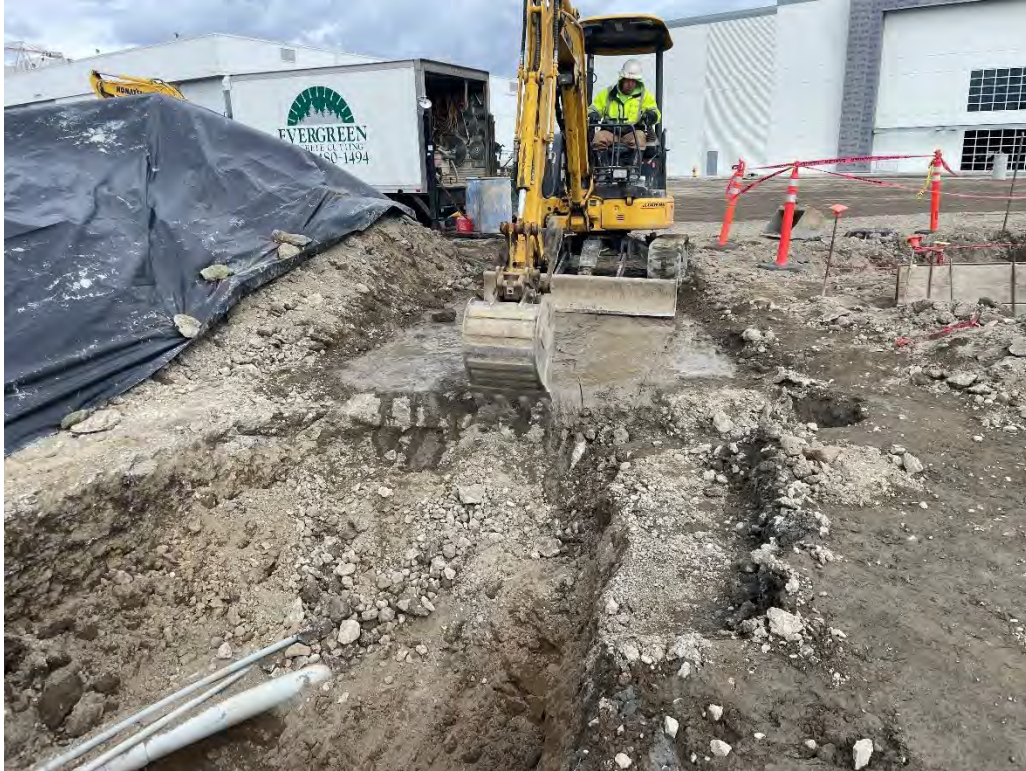
Figure 100: Start Excavating Concrete
