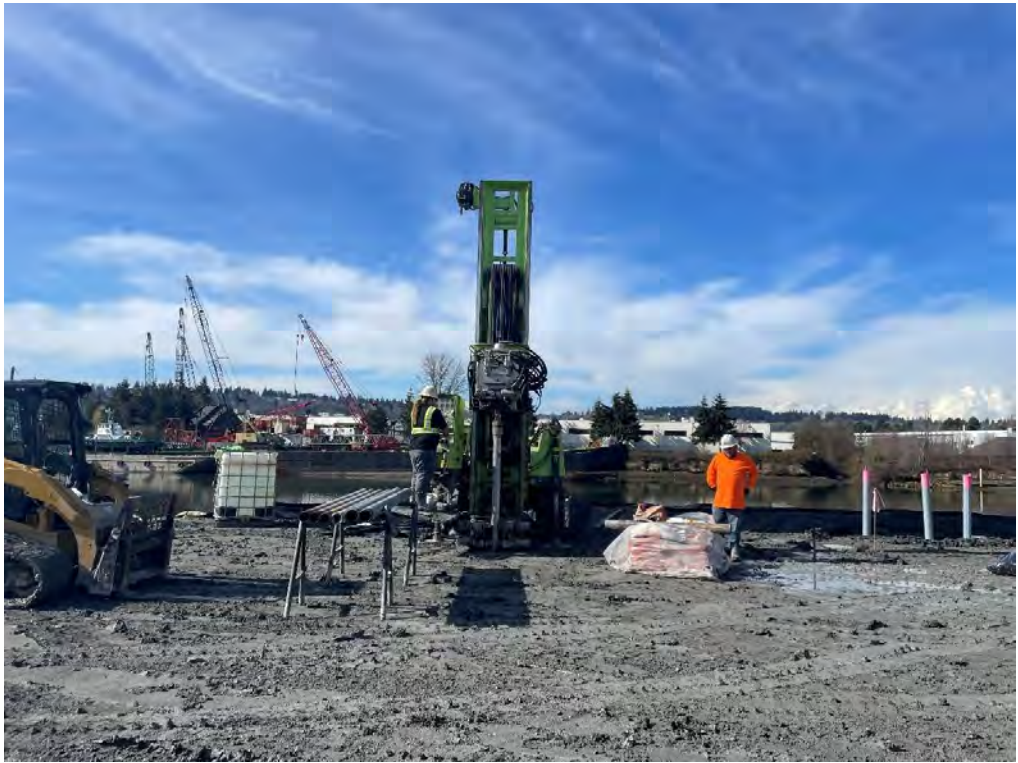
Figure 66: ASW-36 Overview at Start of Drilling
