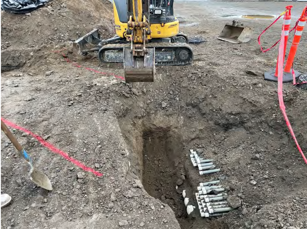
Figure 106: Start Excavation on E Trench
