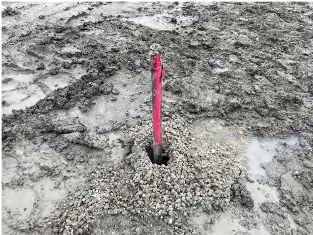
Figure 84: Example of Well Screen after it is inserted into ground/boring hole
