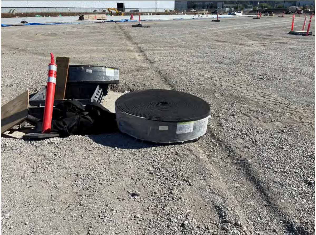
Exhibit 4-2: A Roll of Vent Strip with a “Keyed” Section of Sub-Base for Installation of the Vent Strip
