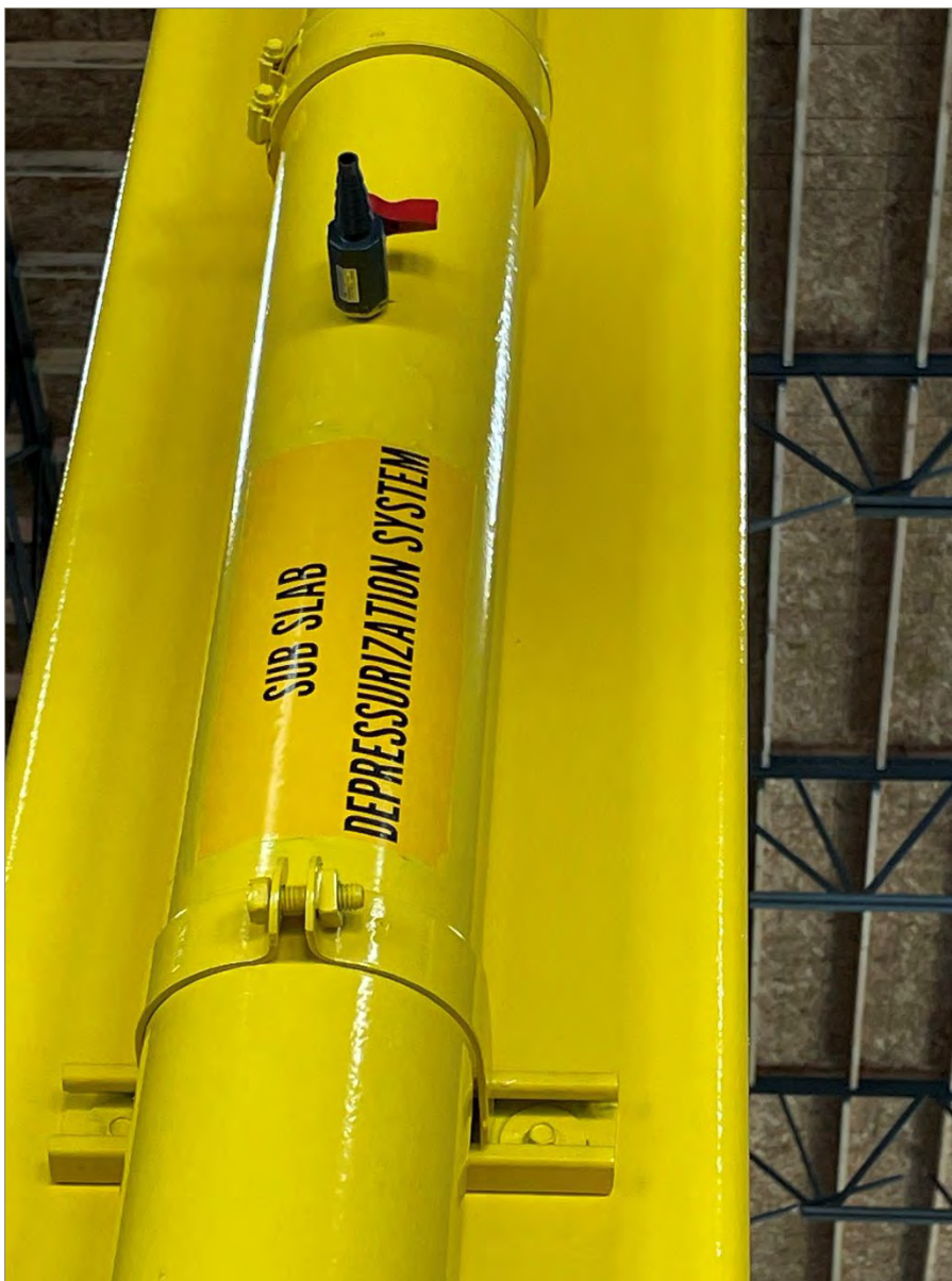
Exhibit 4-7: Riser Pipe with Sample Port and Label
