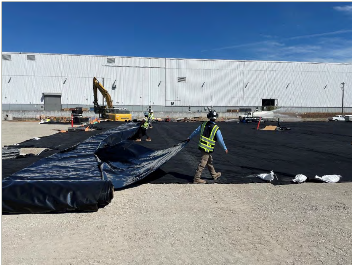
Exhibit 4-3: Unfurling of the Vapor Barrier Over the Geotextile Cushion
