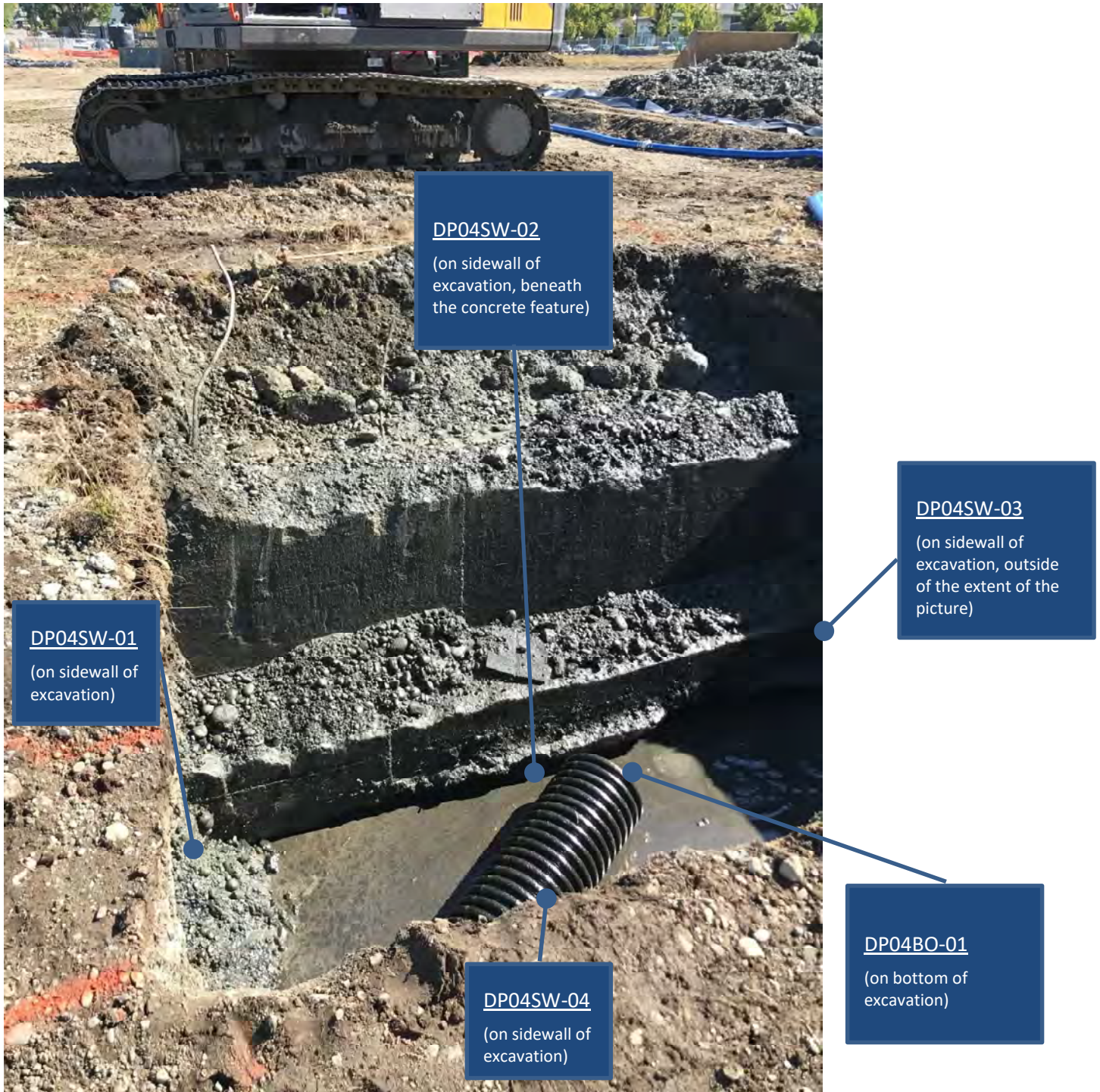
Photo 2: Surgical Excavation DP04 – Round 01 Excavation (looking to the east)
