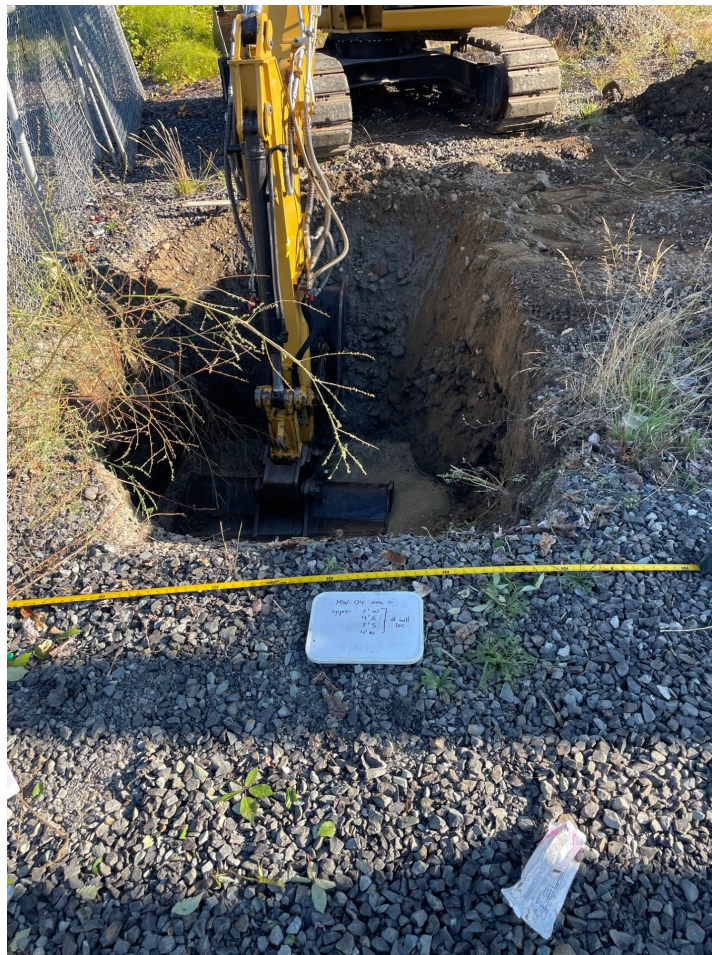
Photograph 6. Completed native soil excavation extent surrounding MW-04 (facing N)
