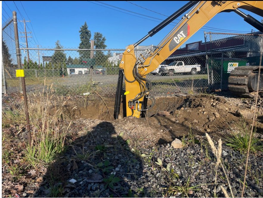
Photograph 5. Excavation to 7.5 foot depth marker on excavator (facing W)
