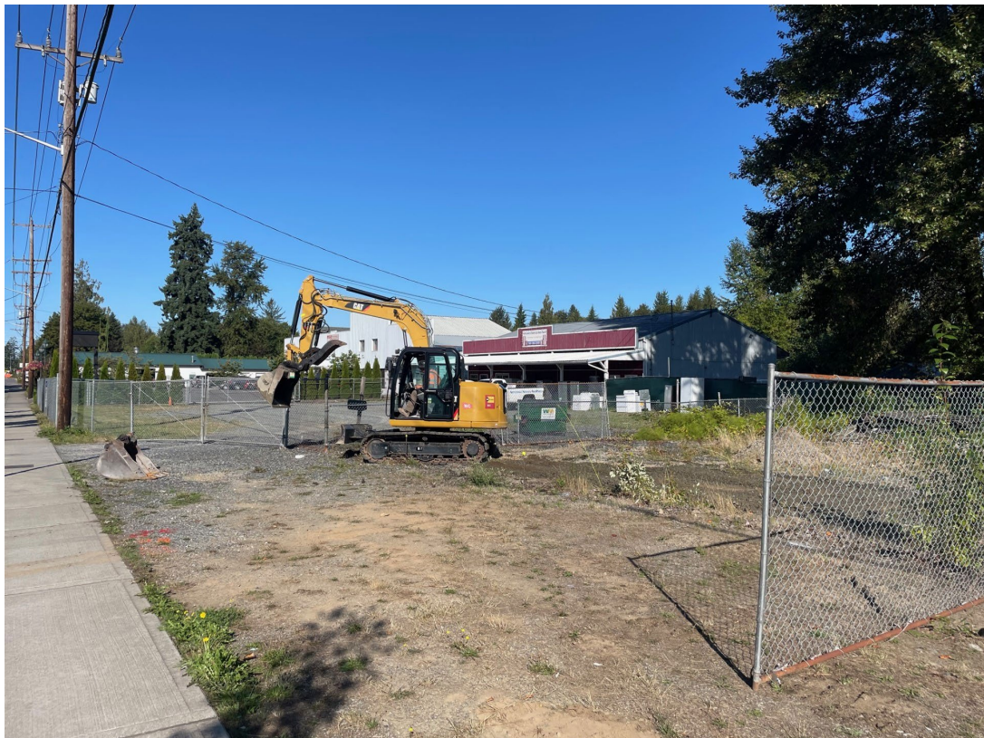
Photograph 10. Excavation backfilled with gravel borrow
