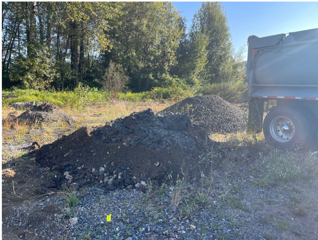
Photograph 7. Temporary contaminated soil stockpile and imported backfill (facing NE)
