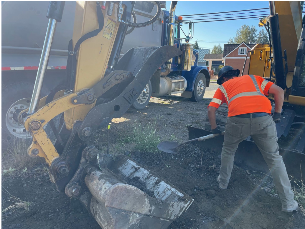
Photograph 9. Full removal of residual contaminated soil stockpile
