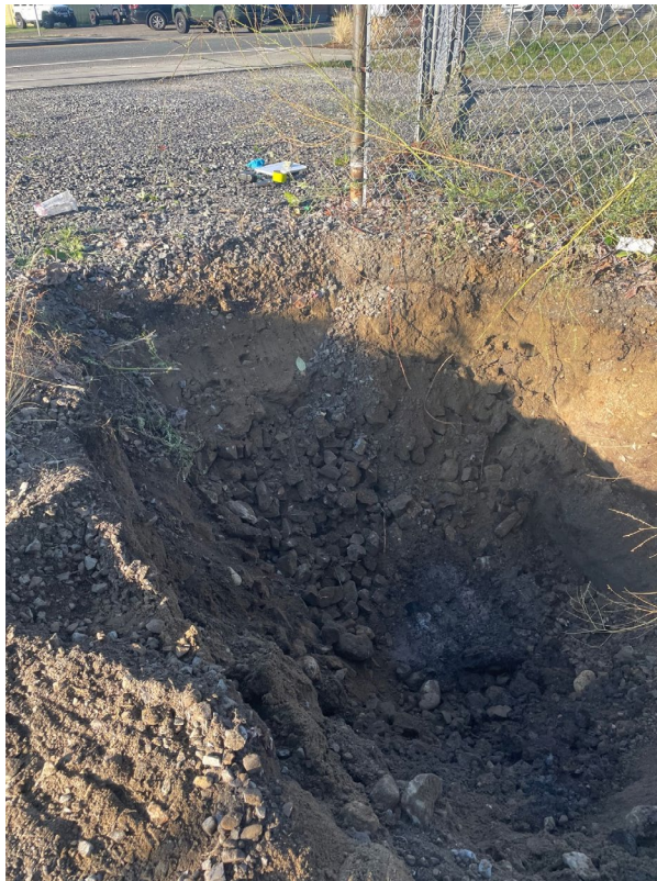
Photograph 3. 2016 excavation quarry spall backfill ~2 feet south of MW-04 (facing SW)
