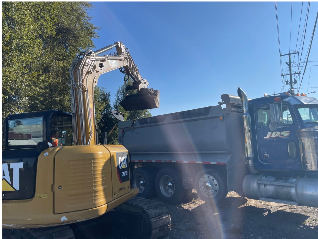
Photograph 8. Contaminated soil loaded for off-site disposal
