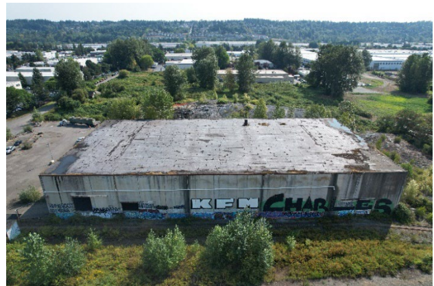
Figure 3: Abandoned smelter building (2023)
