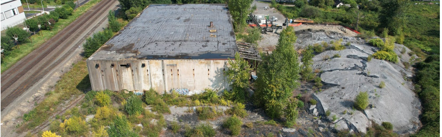
Maralco site aerial photo (2023)
