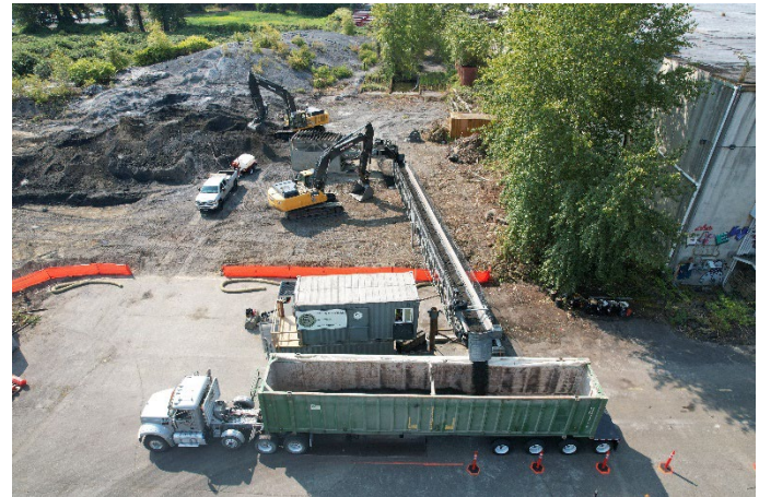
Dross pile removal progress (2023)
