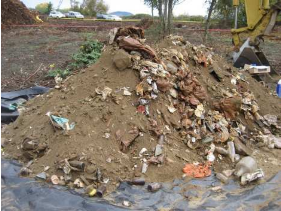
Photo 1. An example of landfill deposits excavated at Whitmarsh Landfill.
