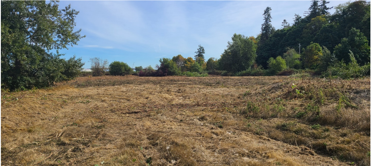
Photo 1 The project site following vegetation removal. View towards the eastern half of the project site.
