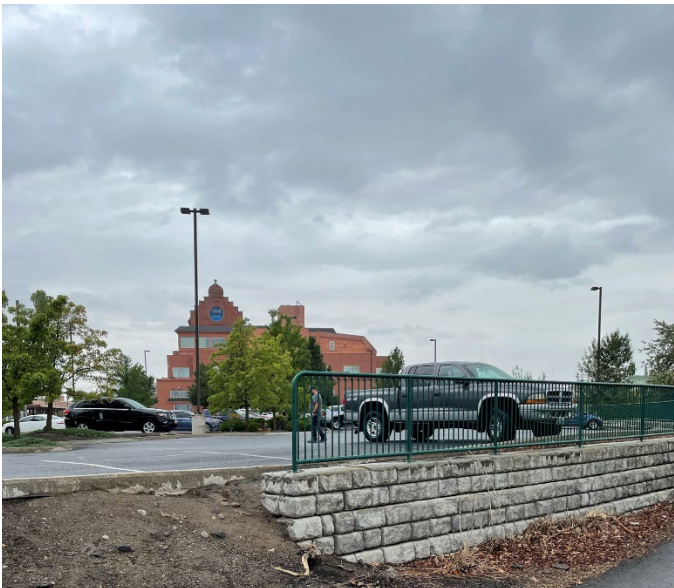
Photo 4: Schade Tower south side of the building – from the east
