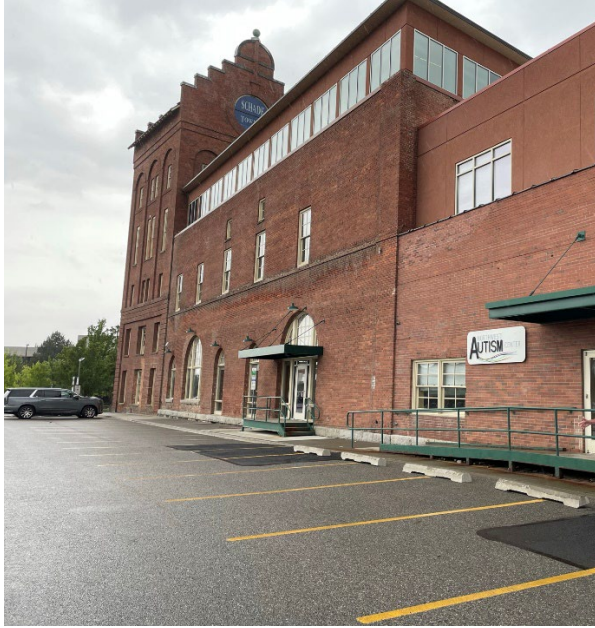
Photo 1: Schade Tower south side of the building – from the east
